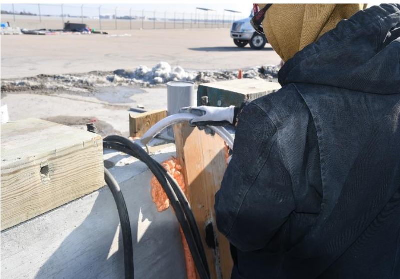
Figure 69. Grout Placement Under Barriers, in Barrier-Barrier Joint Pocket, and Around Inclined Rebar
