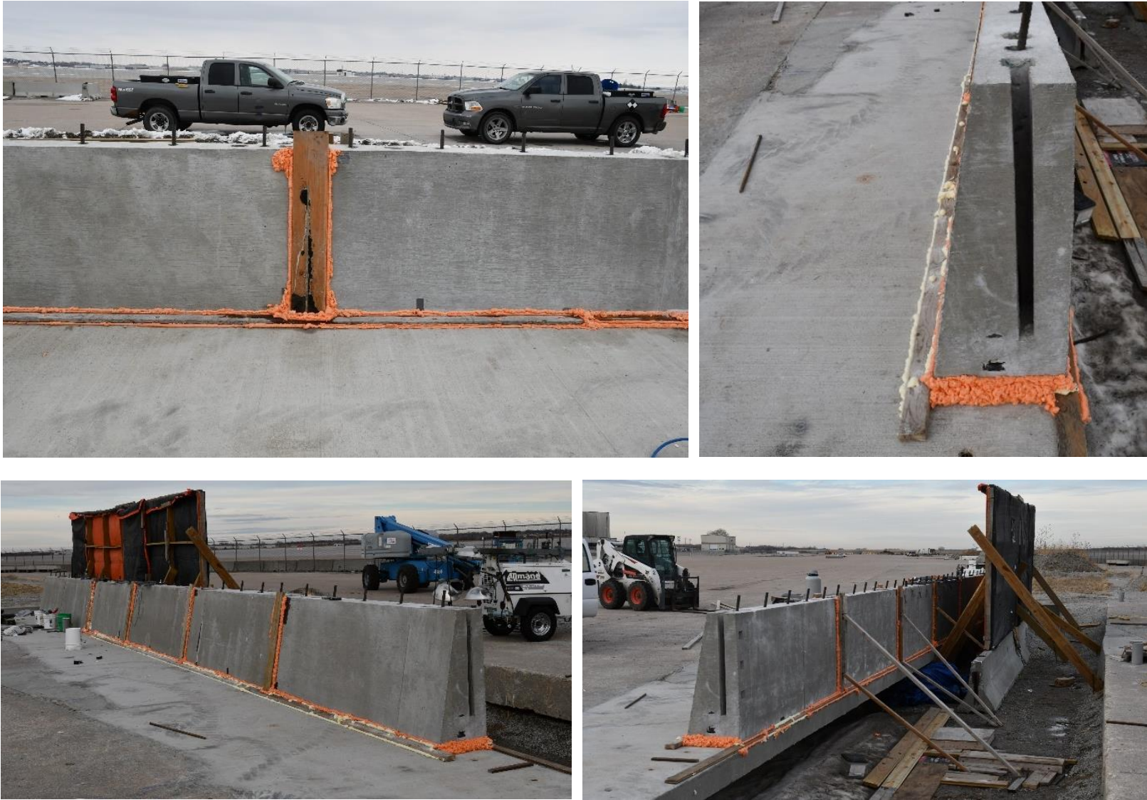
Figure 70. Precast Concrete Barrier Placement Process
