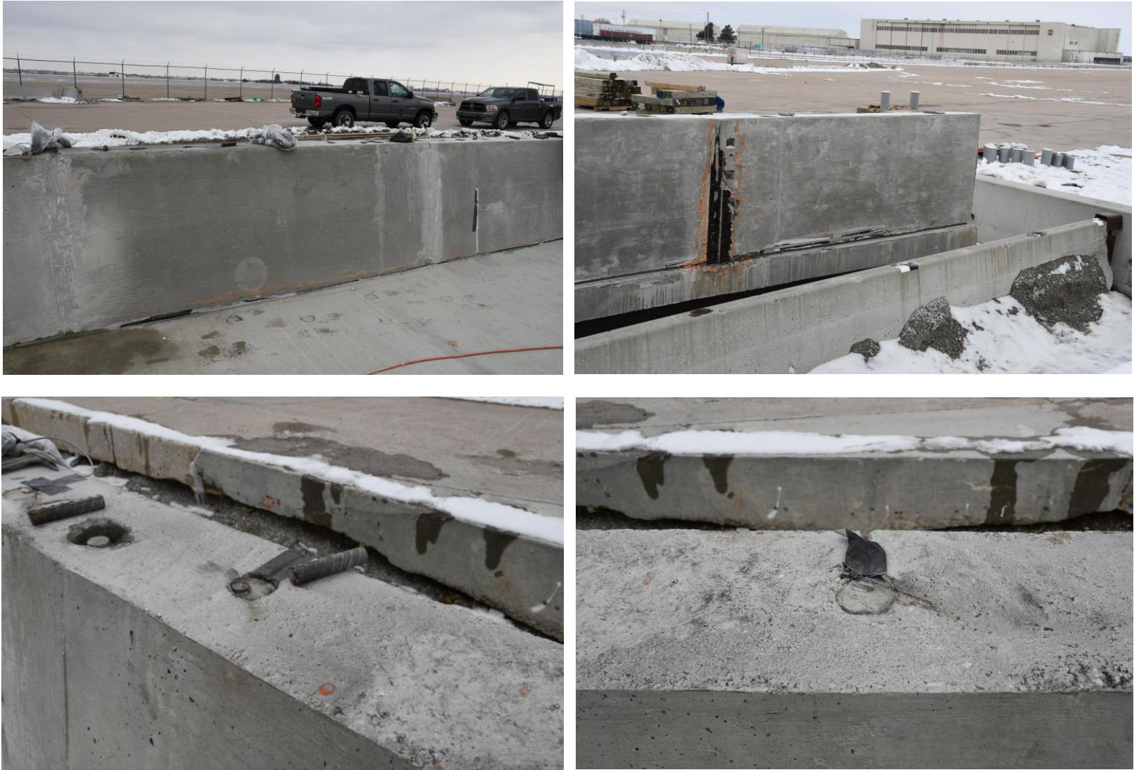
Figure 71. Inclined Bars After Grout Application
