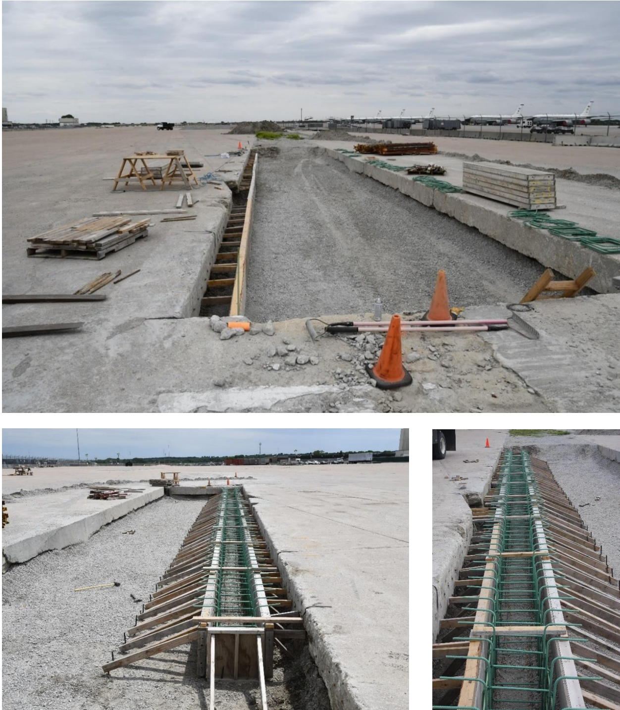
Figure 63. Grade Beam and Anchor Beam Installation
