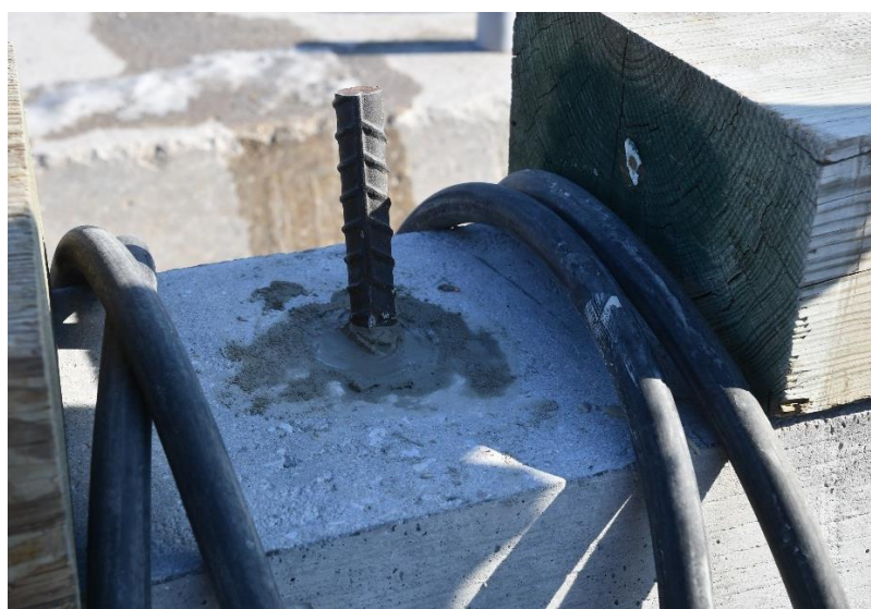
Figure 69. Grout Placement Under Barriers, in Barrier-Barrier Joint Pocket, and Around Inclined Rebar
