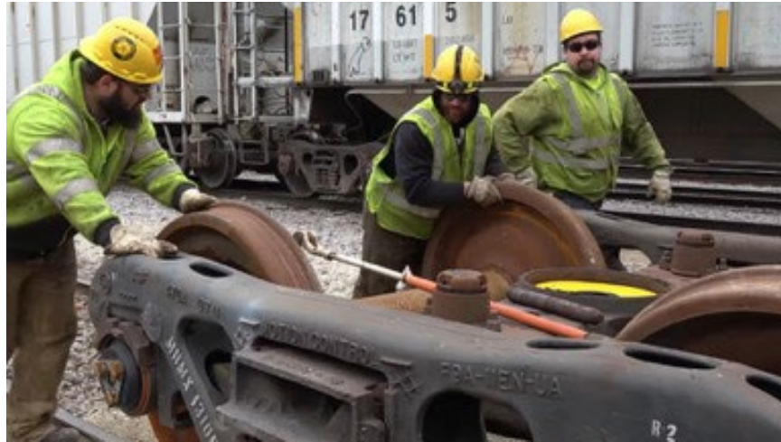
Figure 8. Railcar Wheel Replacement Shows the Stout Pin
