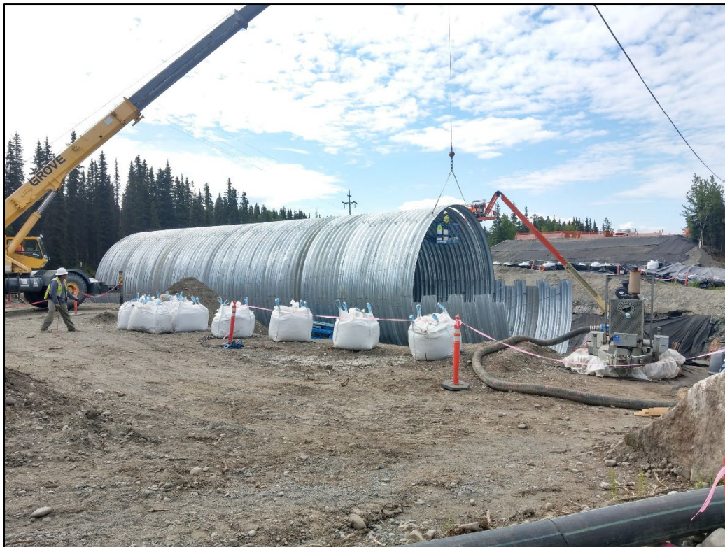
Figure 11. Structural plate pipe being assembled.
