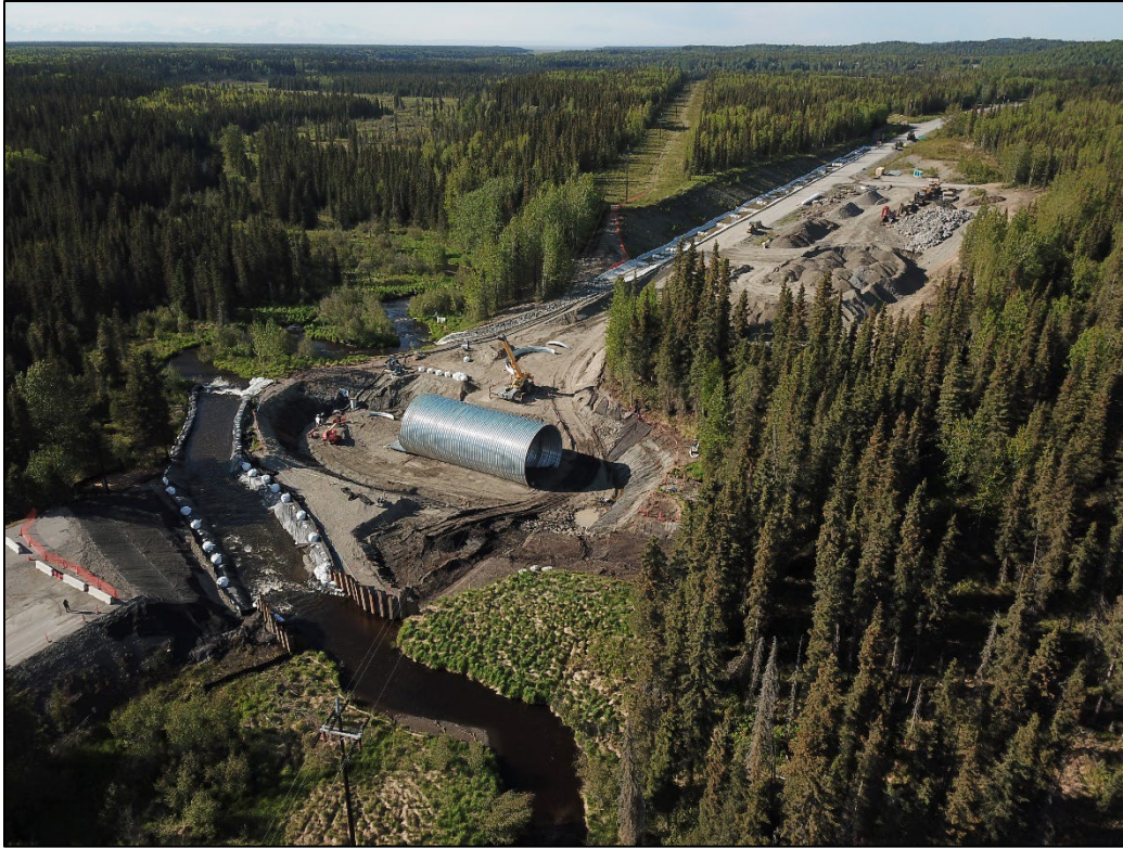
Figure 6. Aerial view of temporary stream diversion and new structure.
