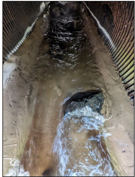
Figure 3. Fish rocks embedded in concrete.
