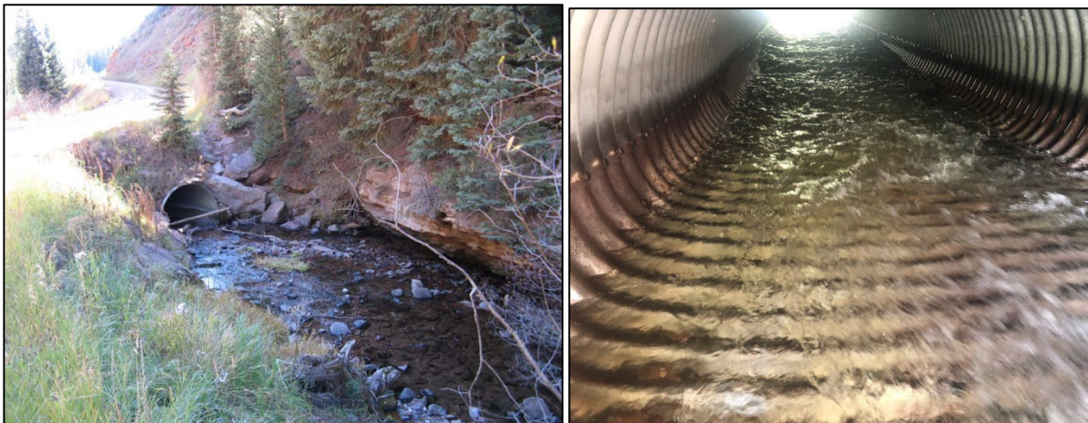
Figure 2. Pre-construction culvert inlet (left) and pre-construction culvert flow conditions (right).
