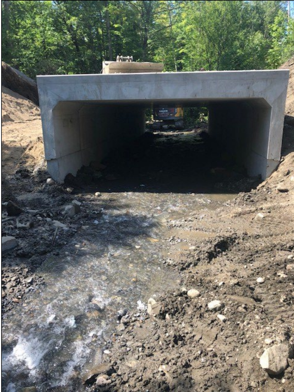
Figure 6. Channel restored, culvert set, beginning of site restoration.
