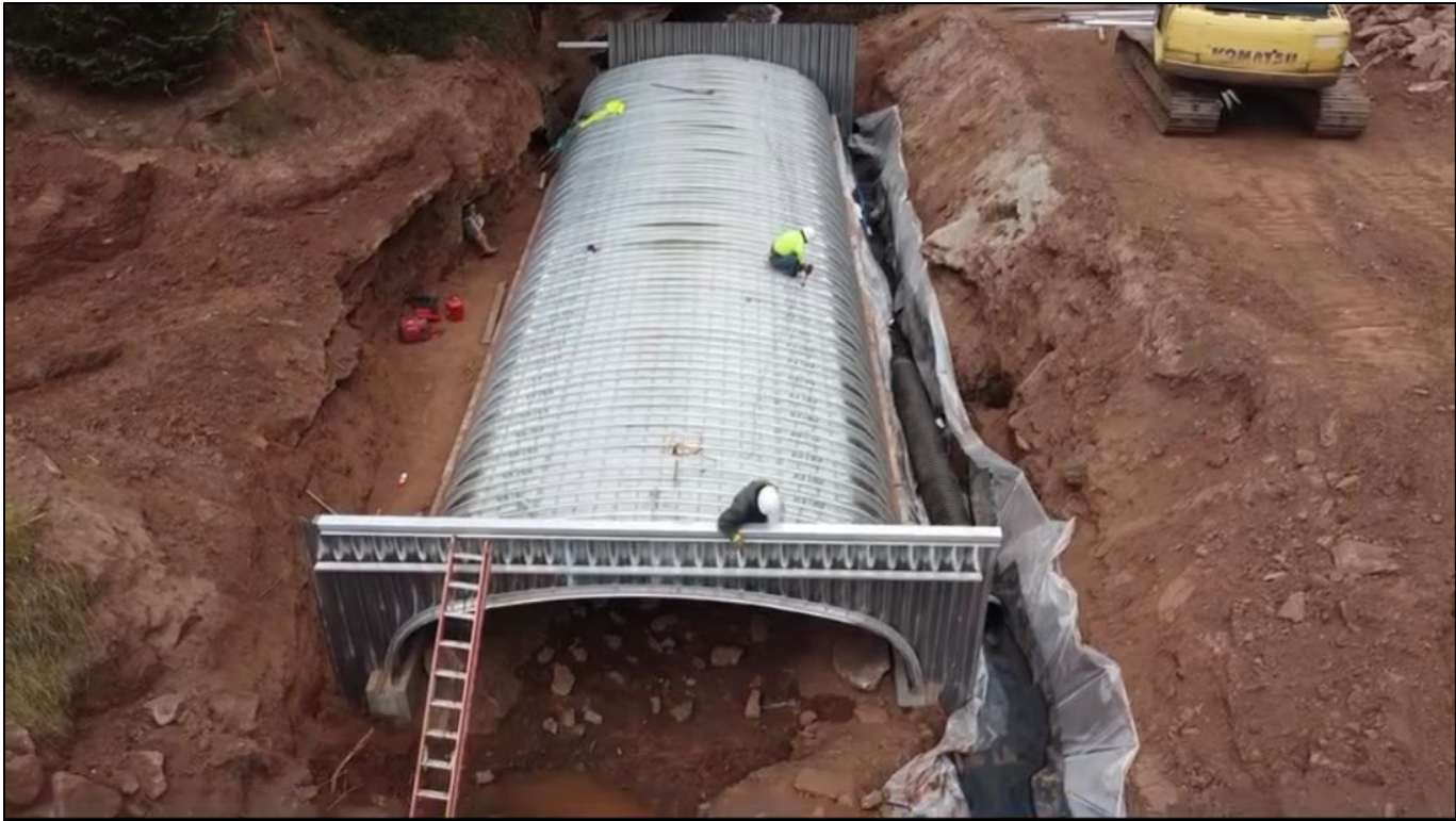
Figure 4. Construction 2022: assembling the structure.
