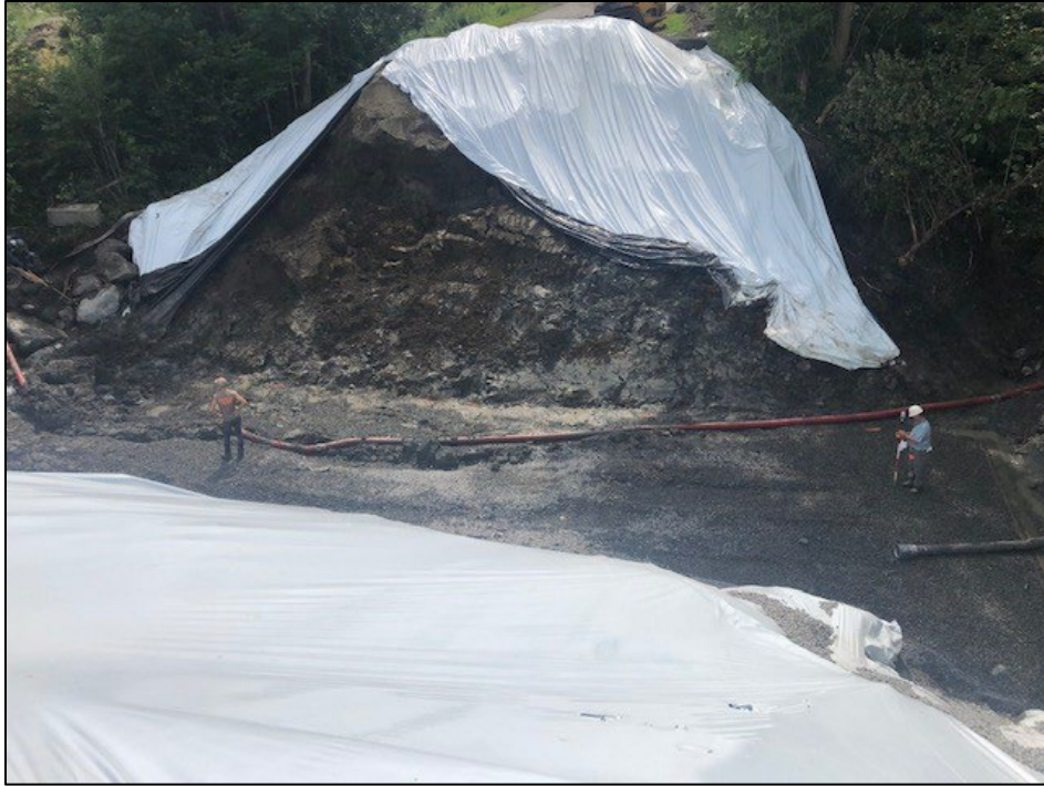
Figure 3. Site prepped for new culvert.
