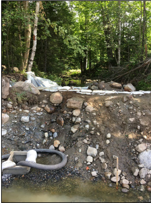
Figure 5. Upstream diversion dam (left) and upstream diversion removed (right).
