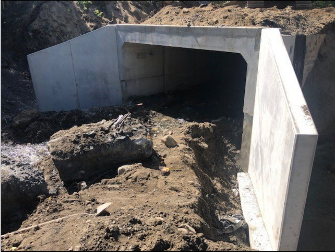
Figure 5. New wing walls set, beginning of channel restoration.
