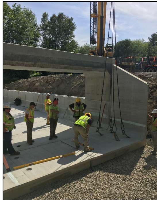
Figure 6. Placing structure segments (left) and placing ends of structure (right).
