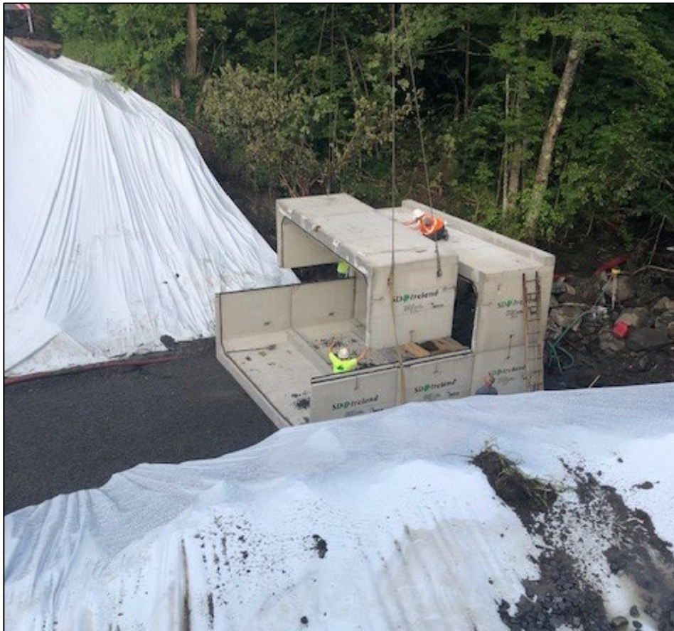
Figure 4. New box culvert placement.
