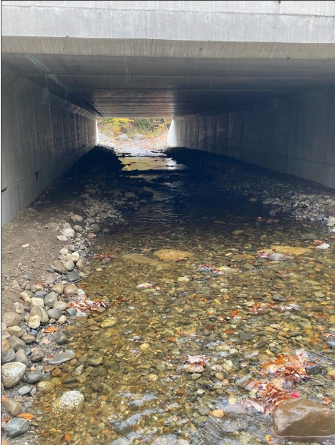
Figure 10. Final constructed streambed with banks.
