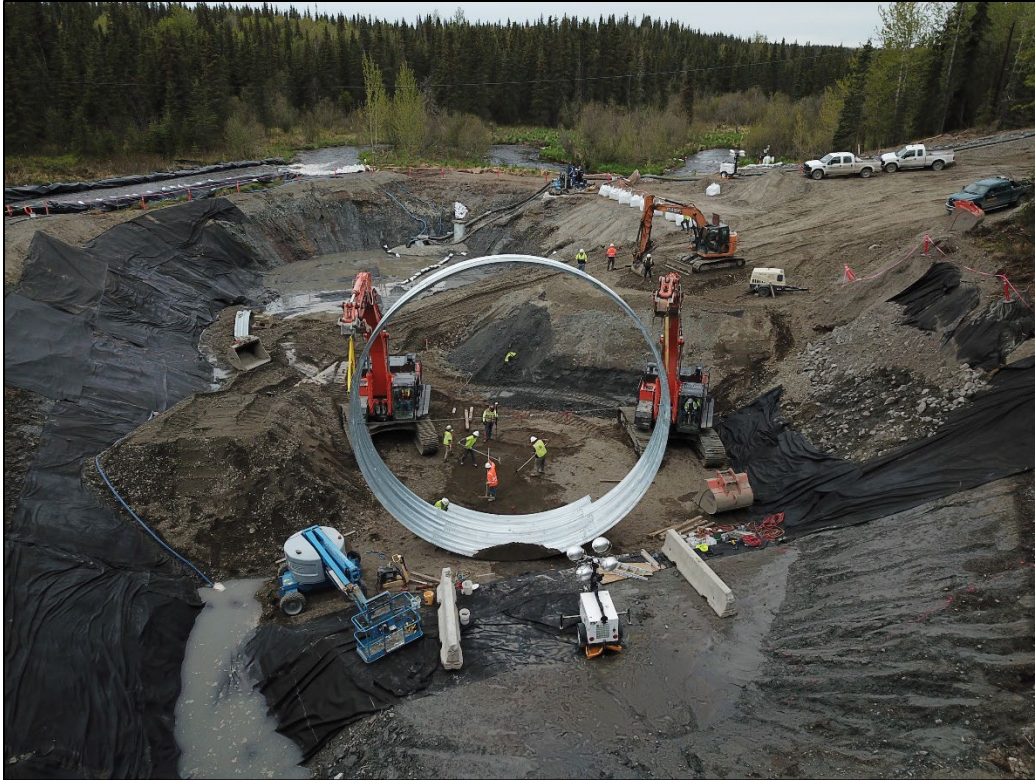
Figure 8. Structural plate pipe being assembled.
