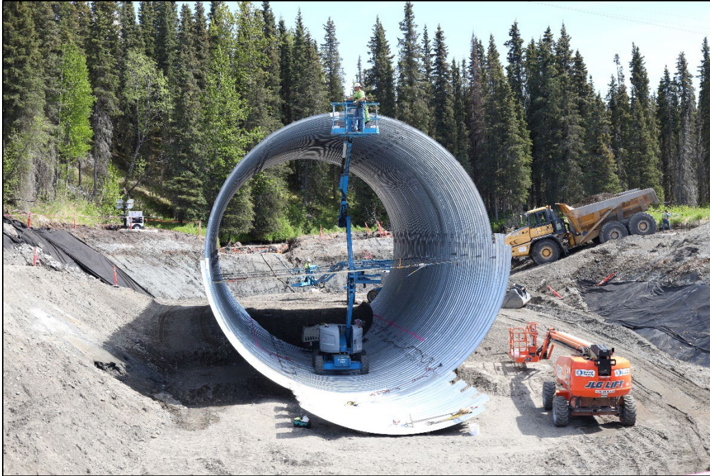
Figure 10. Structural plate pipe being assembled.
