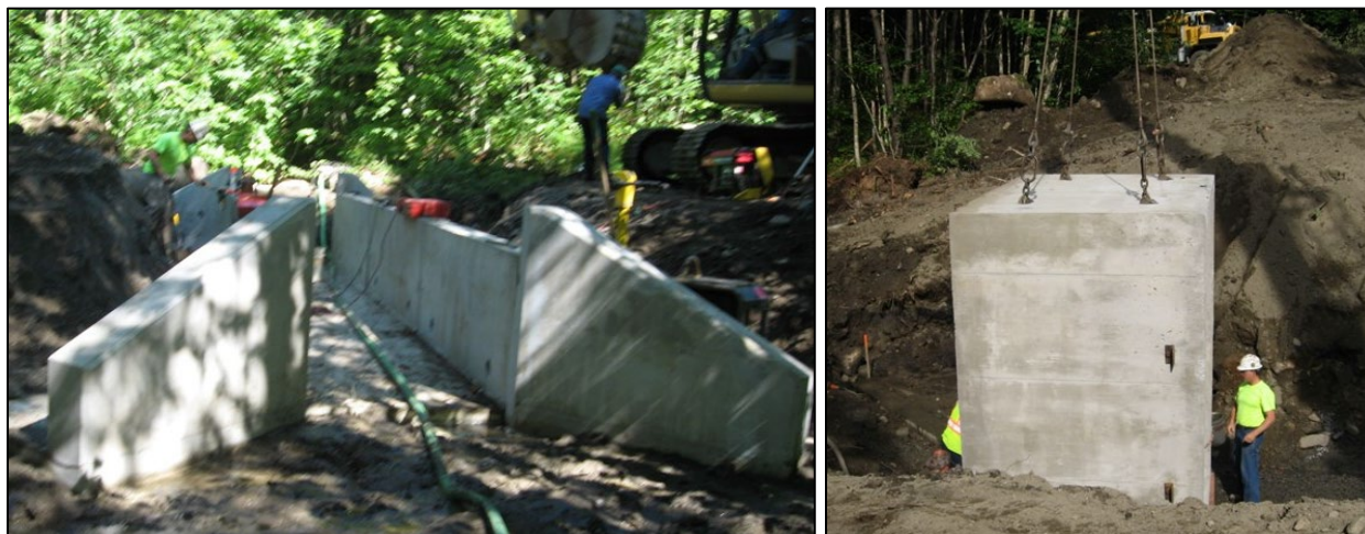
Figure 4. Culvert construction placing the base (left) and top sections (right).
