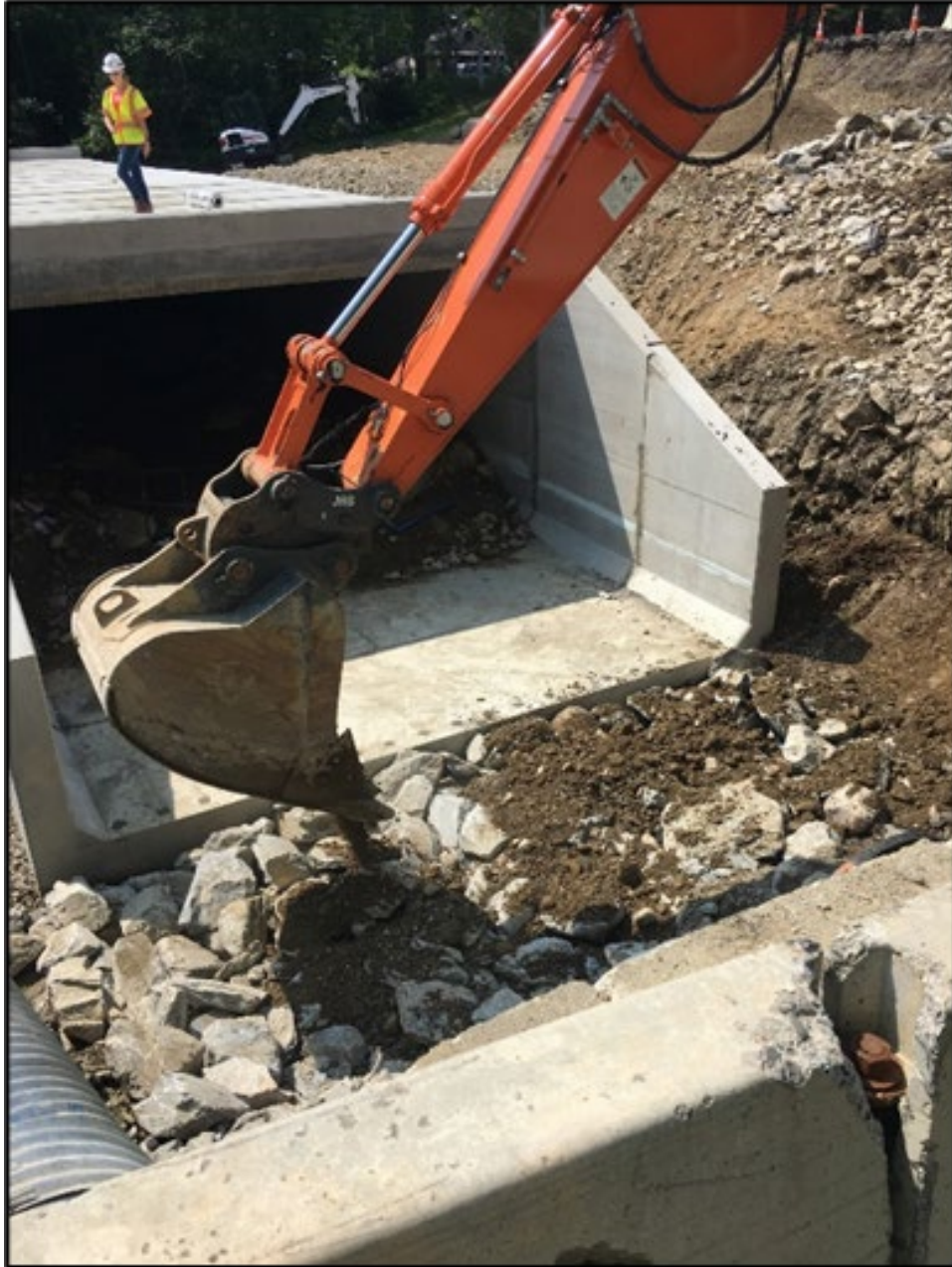
Figure 8. Constructing scour apron.
