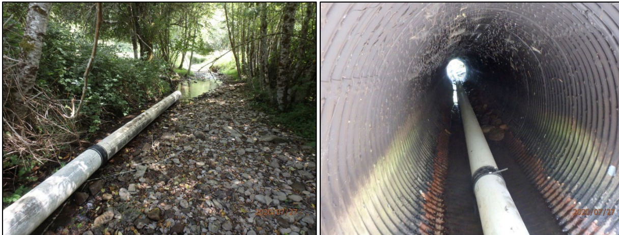
Figure 4. Downstream diversion pipe (left) and diversion pipe in culvert (right).
