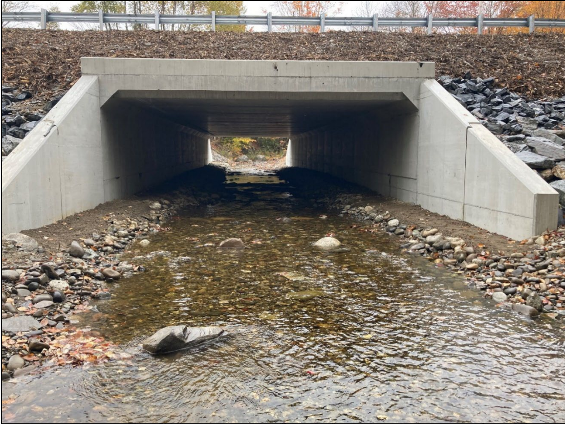
Figure 9. Final constructed water crossing.
