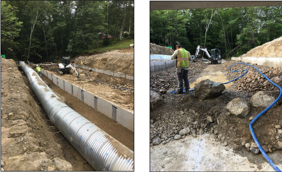
Figure 7. Constructing streambed (left) and constructing streambed and boulders (right).
