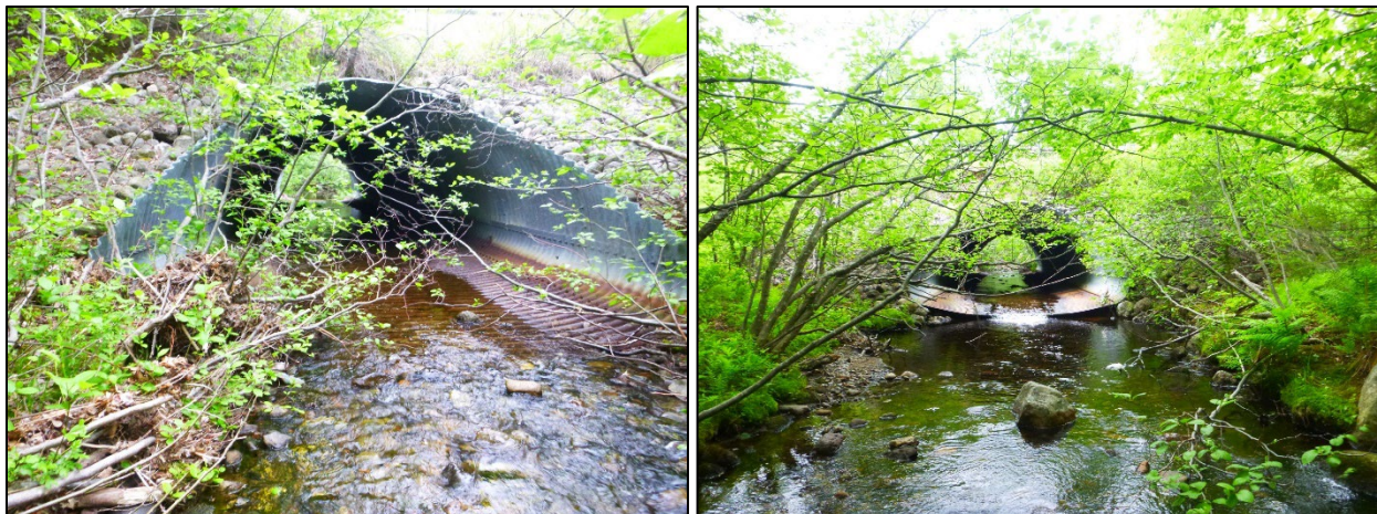
Figure 2. Previous structure inlet (left) and previous structure outlet (right).
