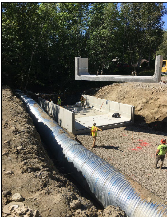
Figure 6. Placing structure segments (left) and placing ends of structure (right).
