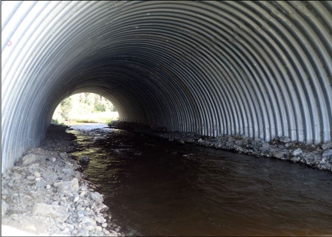
Figure 16. Stable benches in place during 2021 inspection.
