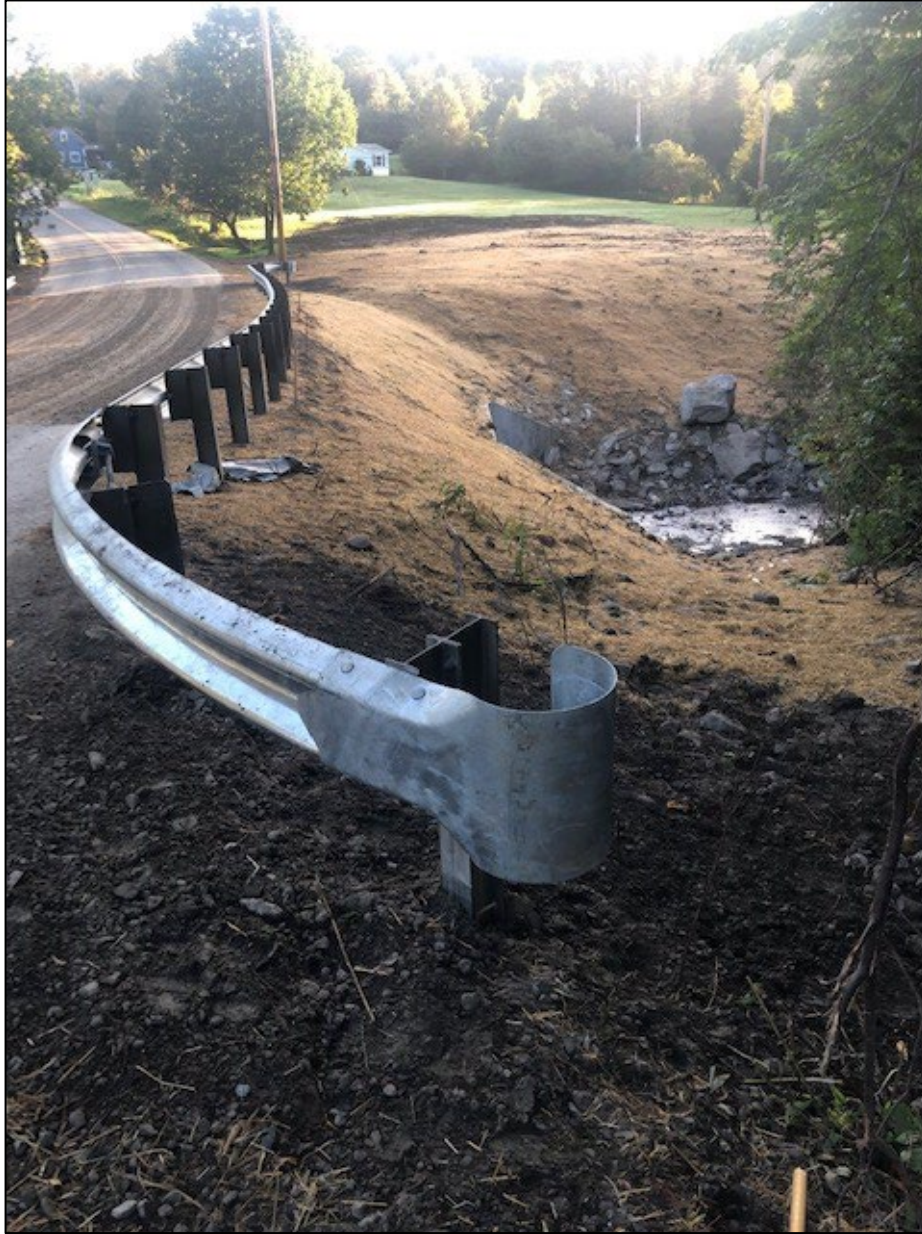
Figure 7. Project completed: site restored and road open.
