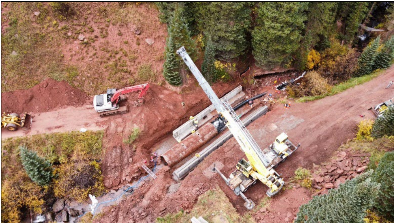
Figure 5. Construction 2022: Setting precast footings with a crane.
