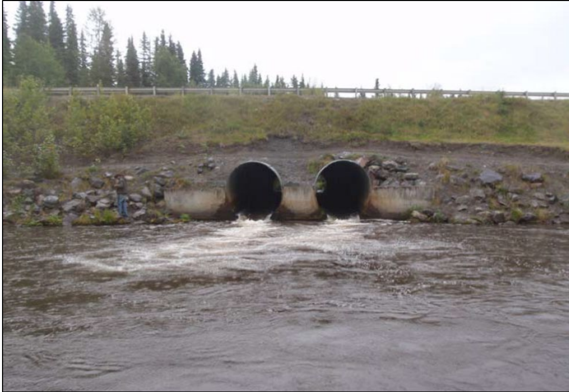
Figure 2. Outlet during 2017 inspection.
