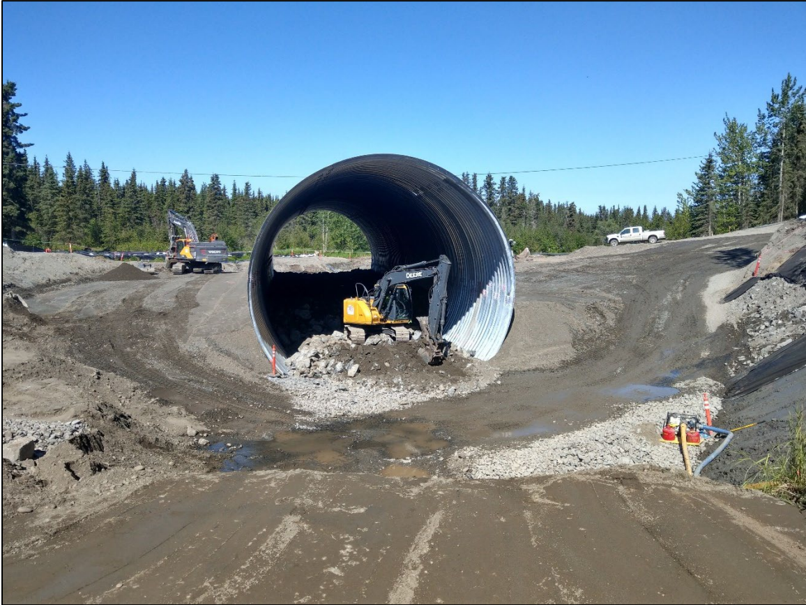
Figure 12. Excavator placing the streambed inside the structure.
