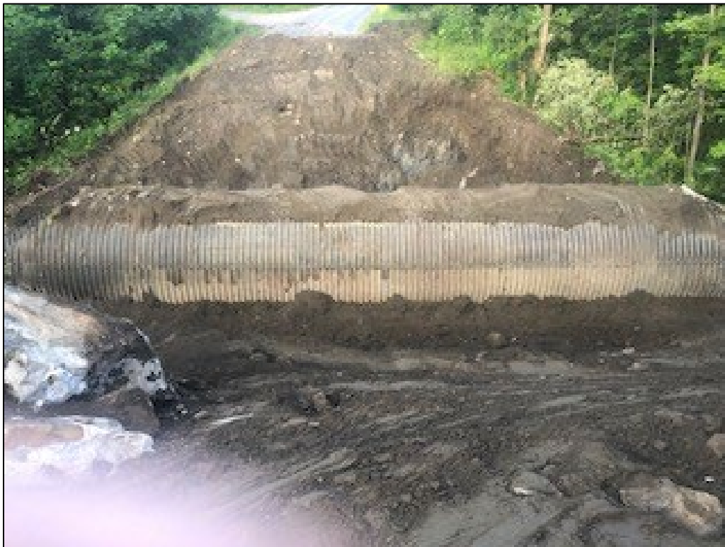
Figure 2. Fill removed and old pipe exposed.
