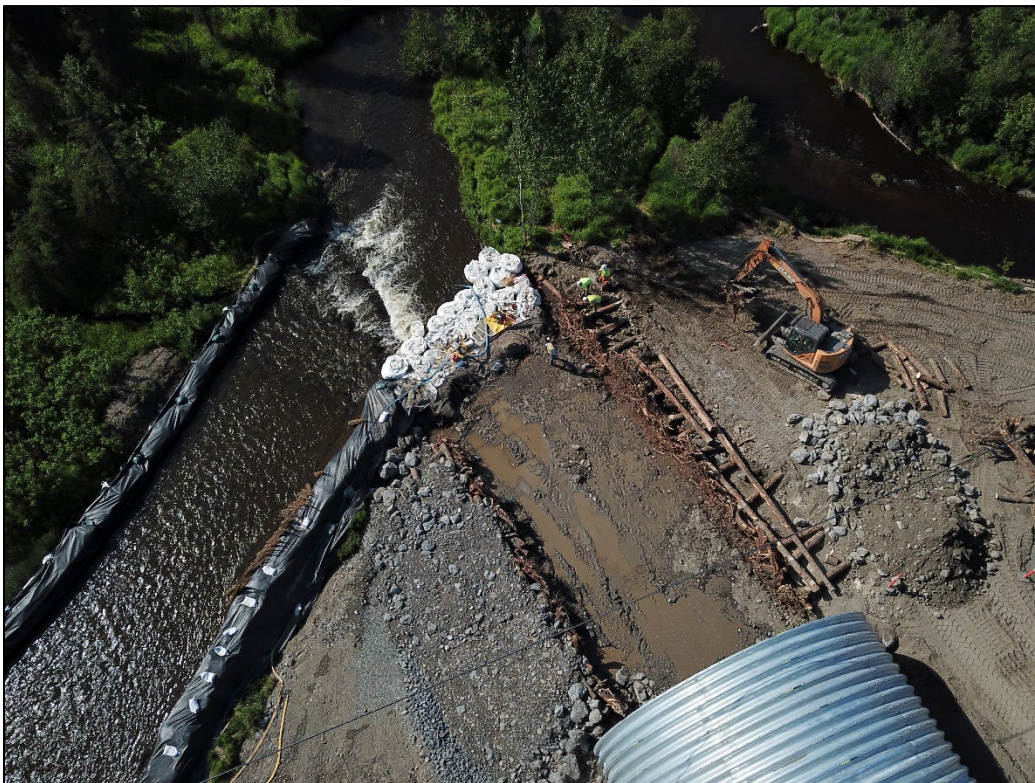
Figure 7. Aerial view of temporary stream diversion.
