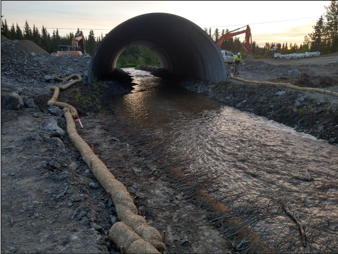
Figure 13. Crooked Creek reintroduced to new water crossing.
