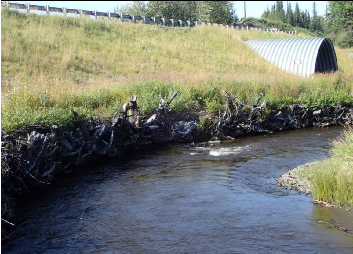
Figure 17. Performance of rootwads upstream during 2021 inspection.
