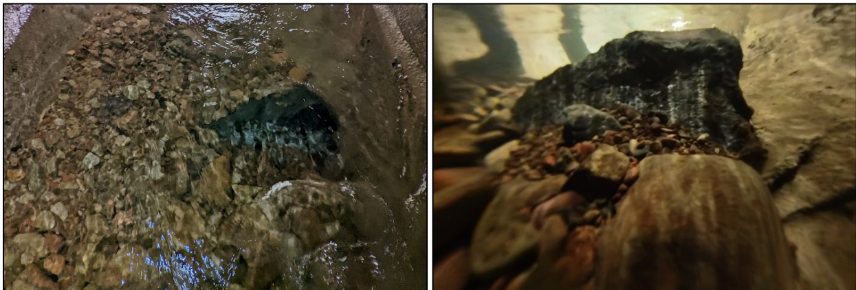
Figure 6. Fish rock with streambed material (left) and downstream side of fish rock with deposition (right).
