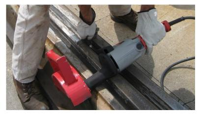
Figure 91. NS grinding of repaired areas back to profile
