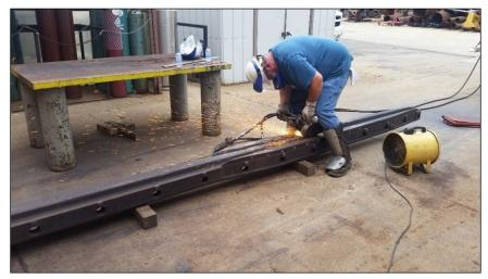
Figure 28. Grinding of repaired CSX frog
