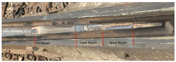
Figure 100. Weld repair segments on point before grinding back to profile
