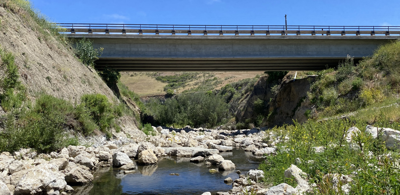
Salsipuedes Creek is one of the largest full-span bridge undercrossings that has been developed and implemented for the primary purpose of fish and wildlife connectivity. Post project monitoring verified successful migration of steelhead trout, mountain lion, bear, fox, and deer. Credit: Photo Courtesy of Caltrans
