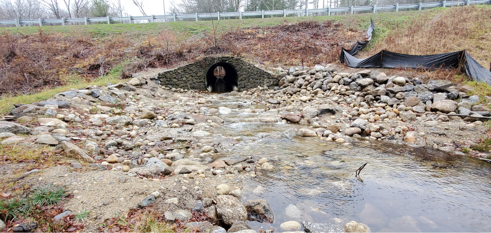
Completed fish weir in Bartlett Brook. Credit: Photo Courtesy of NHDOT
