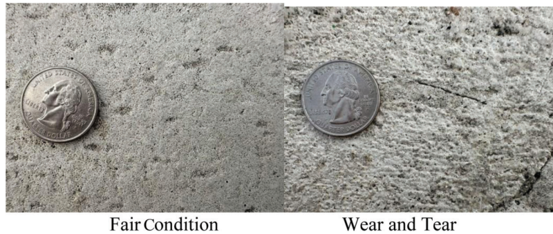
Figure 2.24 Closeups of roundabout crosswalk markings in different conditions.
