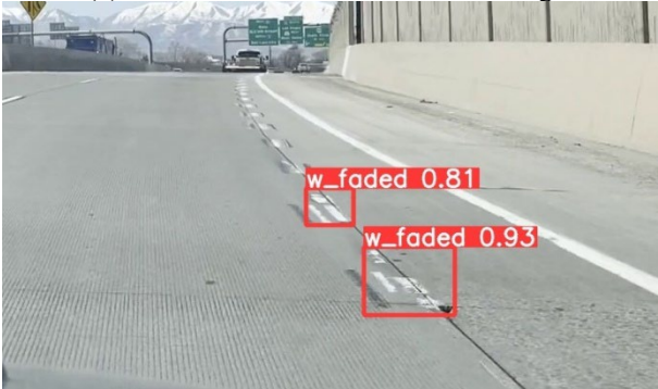
(c) Faded white dot lane marking
