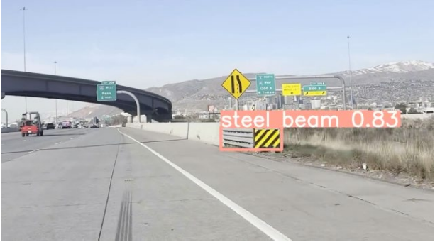
(a) W-beam steel guardrail
