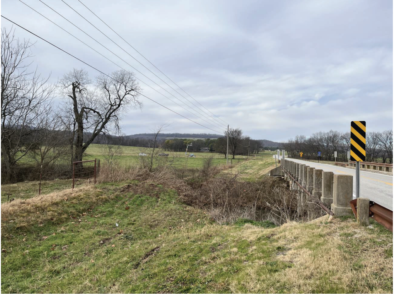
Figure 12. Photo of Lincoln Bridge 1 (East) (Job 040866)
