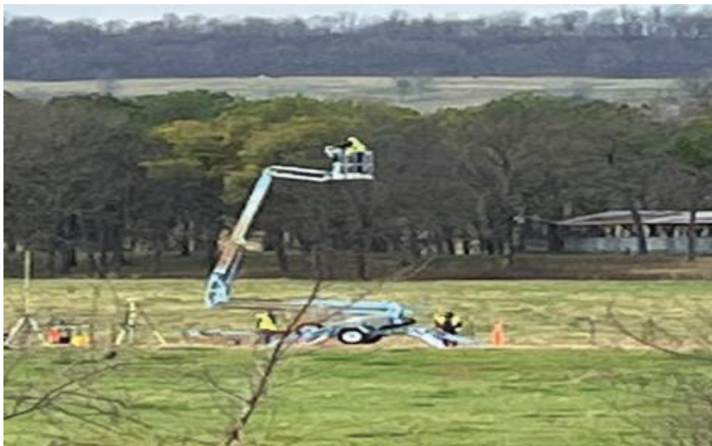
Figure 5. Manlift (55 ft) for Lifting the UAS Operator to Maintain His/Her Visual Line-of-Sight During Flight
