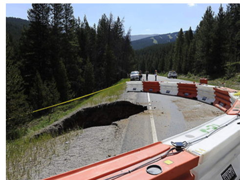
Figure 1. Example of culvert failure (Source: FHWA)
