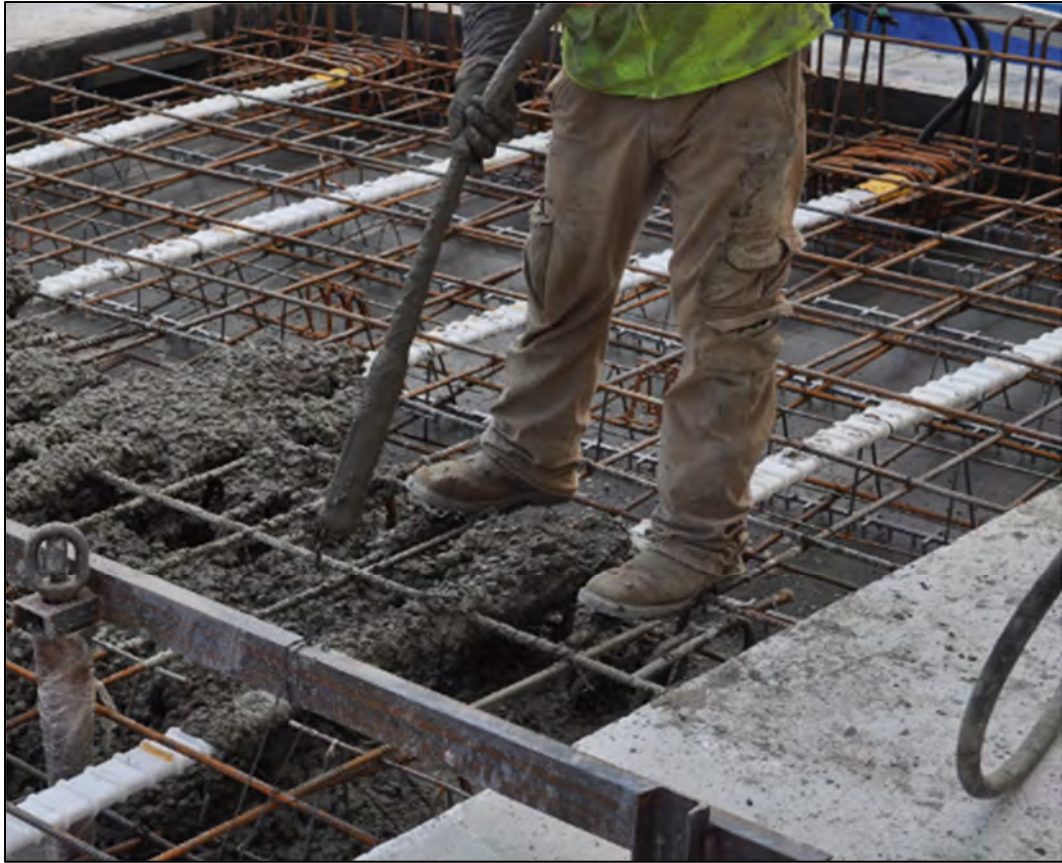
Figure 5-11: Consolidation using a portable vibrator
