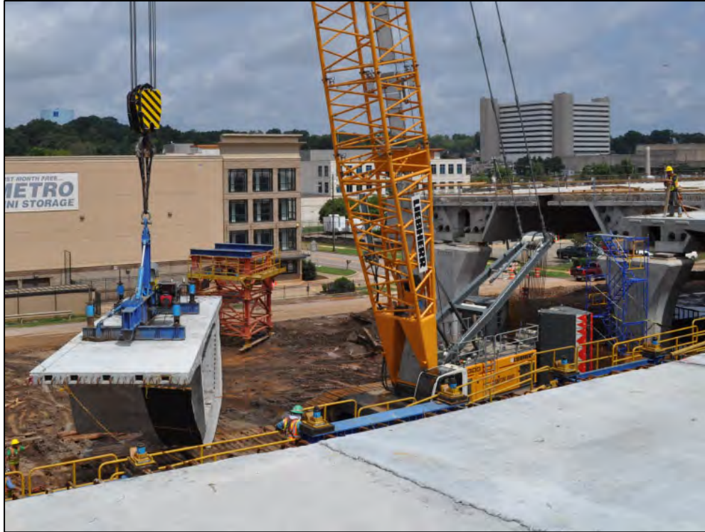
Figure 5-16: Crane lifting a segment into place
