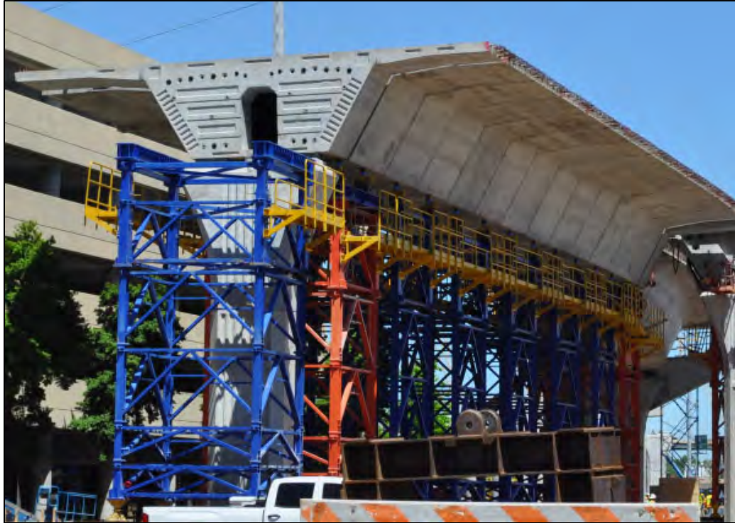
Figure 1-2: Birmingham I-59/I-20 segmental bridge during construction
