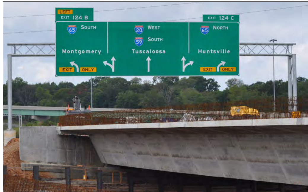
Figure 1-1: Birmingham I-59/I-20 segmental bridge during construction
