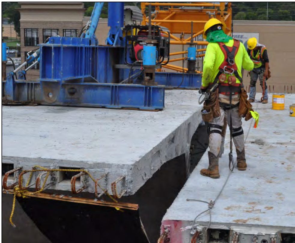
Figure 5-17: Segment being guided into place on falsework
