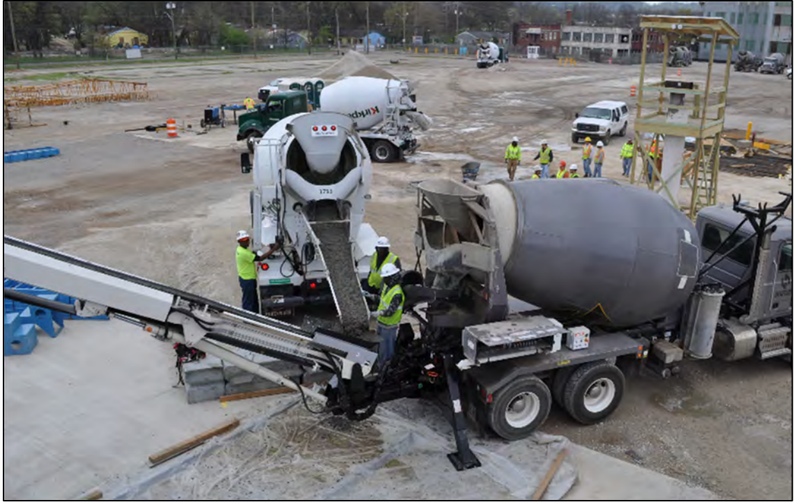
Figure 5-8: Conveyor moving concrete to desired location at the top of the formwork
