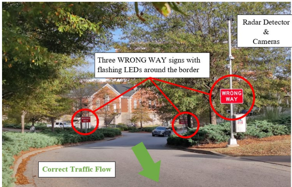
Figure 2 Wrong-way alert system configuration
