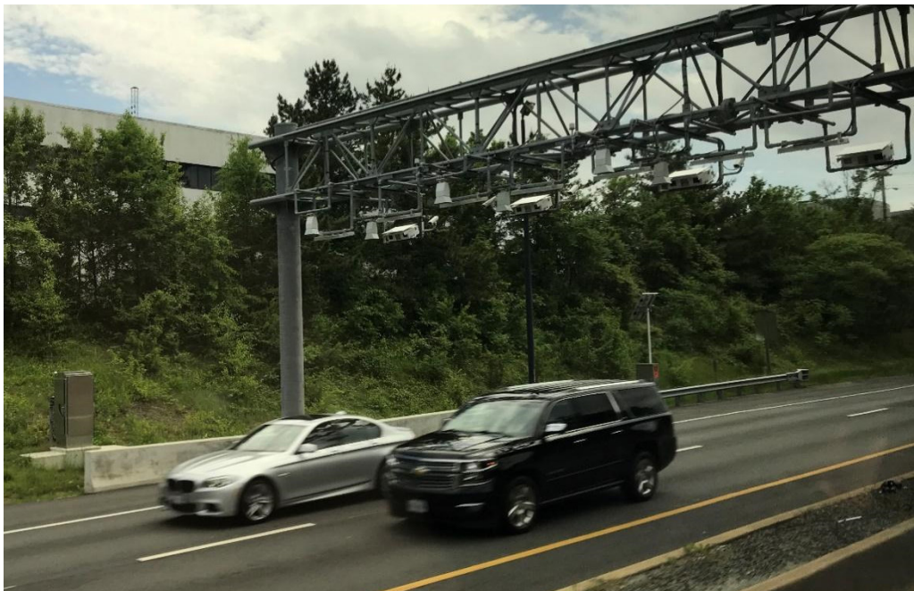
Figure 13. Photo. High-speed toll collection gantry.
