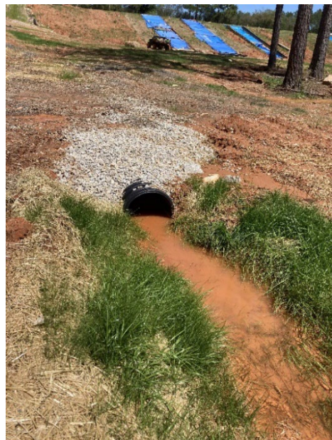
(b) drainage pipe outlet
