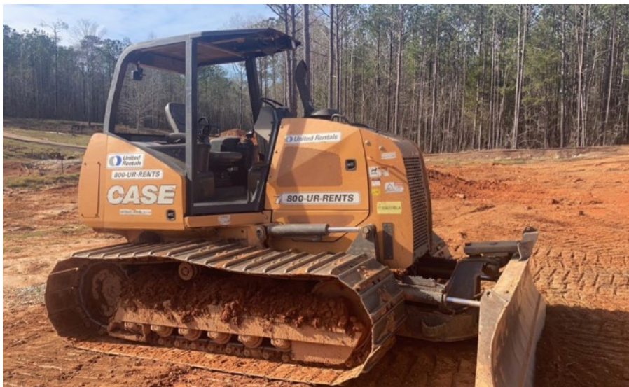
Figure 3-8: Bulldozer for Regrading
