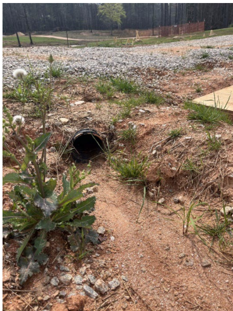
(a) plot 7 culvert
