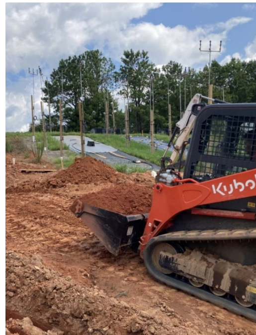
(b) adding soil to plot with skidsteer
