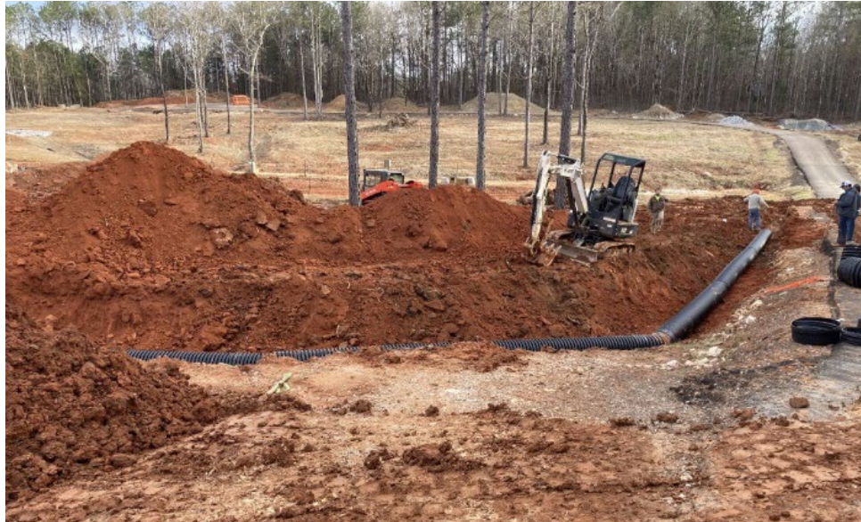
Figure 3-13: Drainage Pipe Installation
