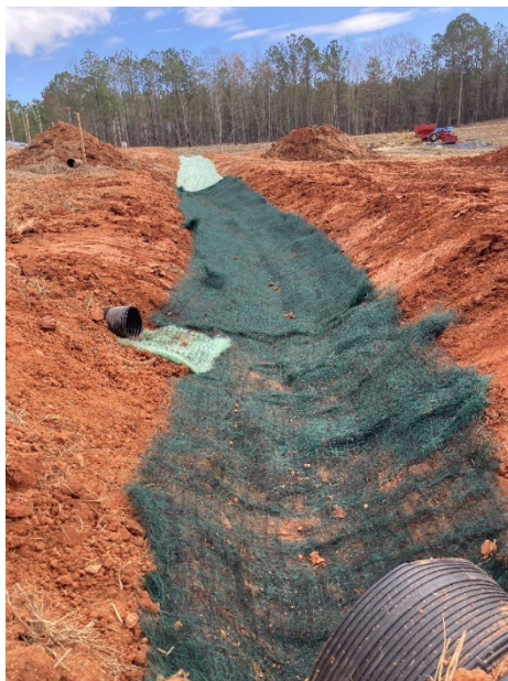
(a) TRM installation
