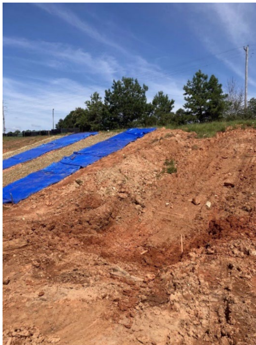
(a) plot 8 excavation
