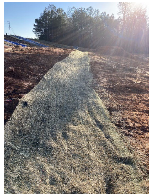
(b) ECB installation
