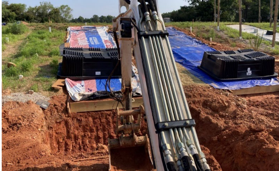
Figure 3-11: Excavation for Catchment Basin and Anchoring
