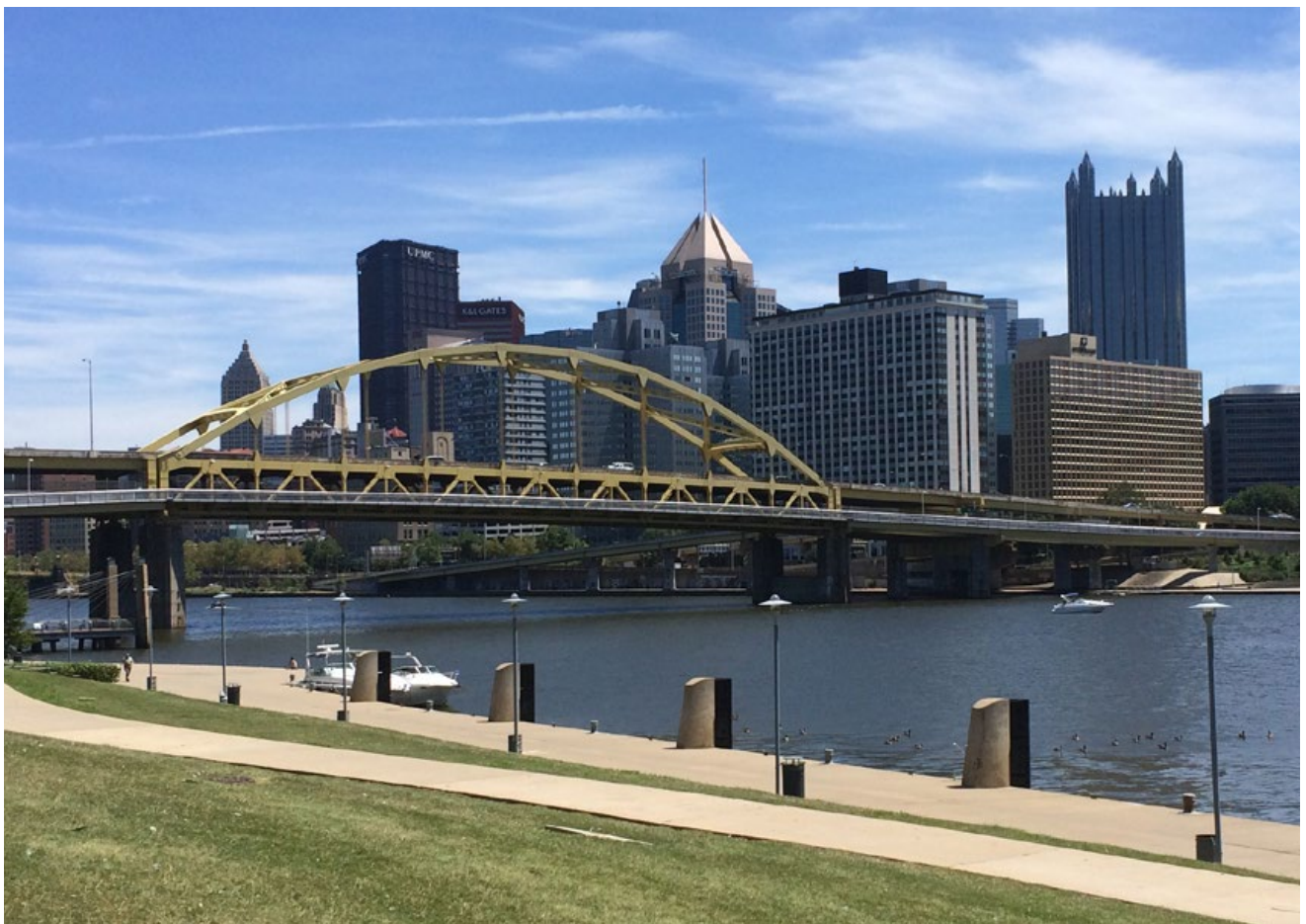
The Fort Duquesne Bridge, awarded funding for improvements, is a steel bowstring arch bridge that opened for traffic in October 1969.
