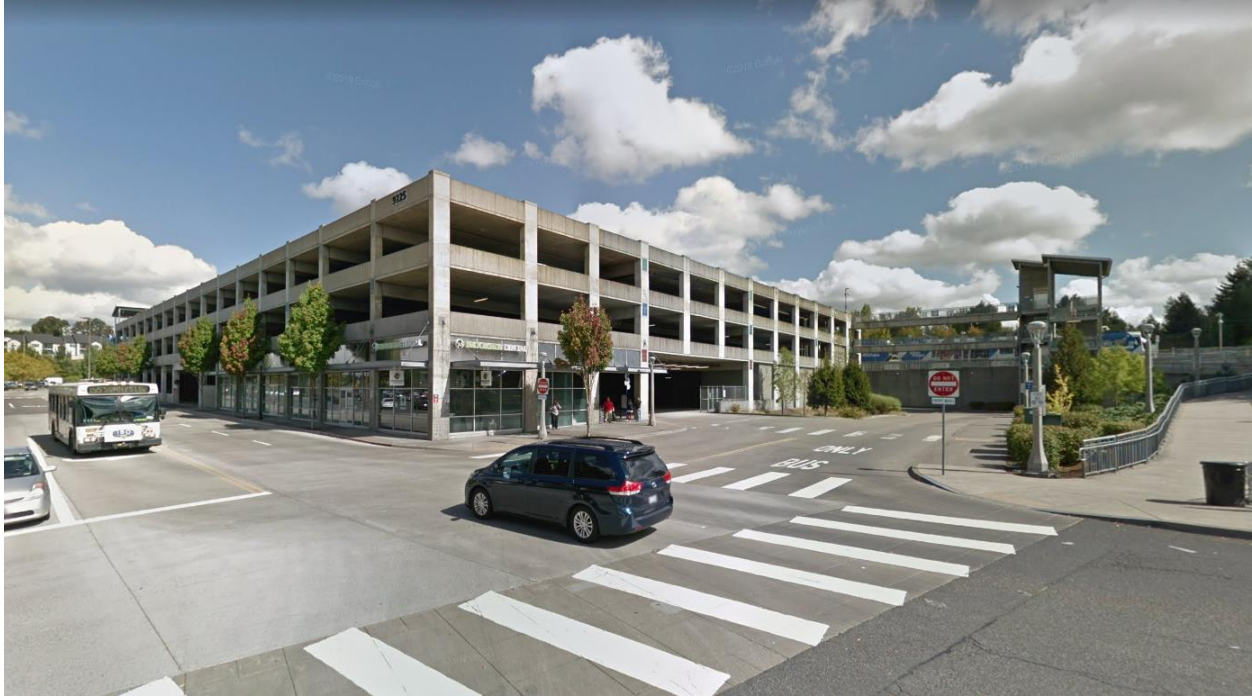
Figure 13 Street view of the Clackamas TC covered parking facility (Google Earth)
