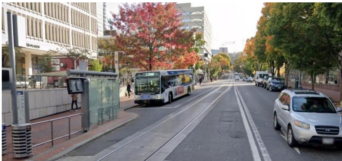
Figure 9 Mall qualities: Bus stop, bus bay, and sightlines of light rail (Google Earth)
