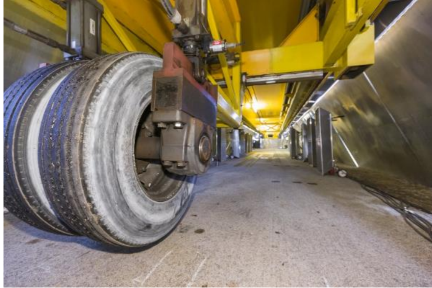
Figure 10. Photo. Inside the temperature control enclosure.
