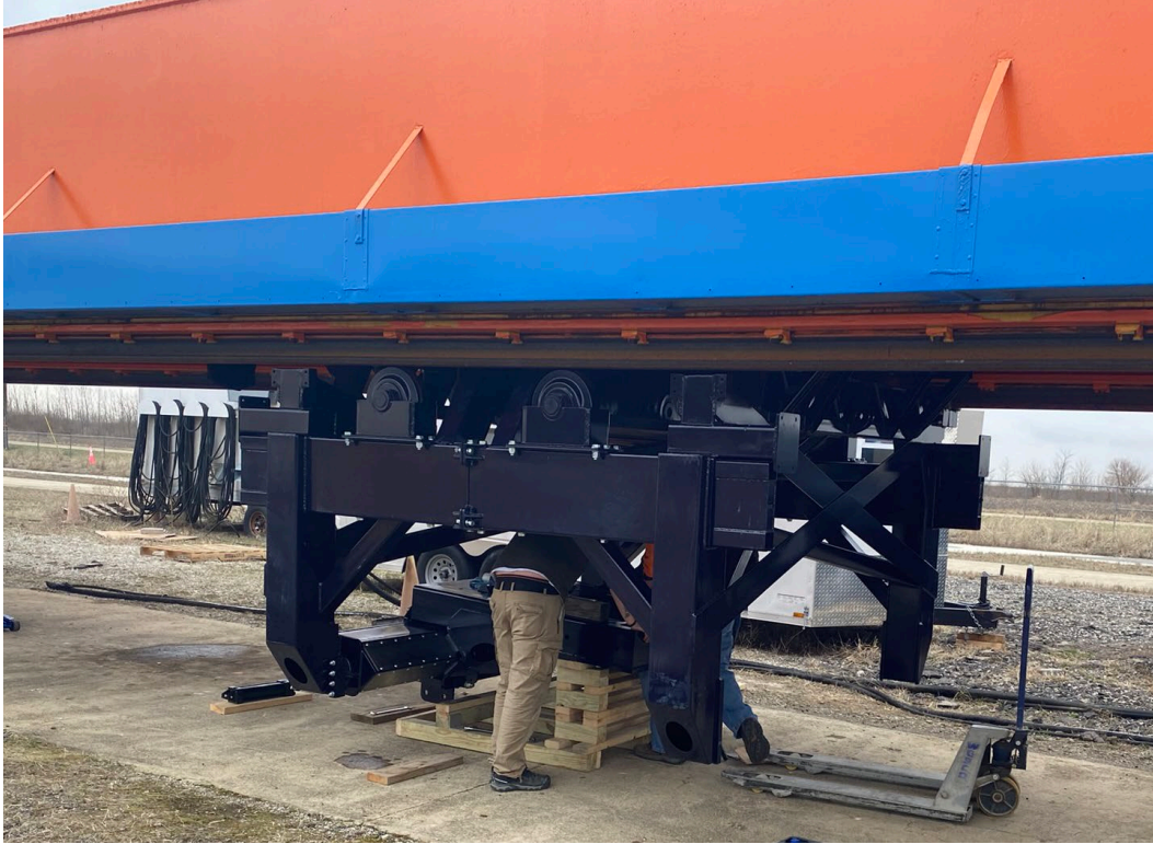
Figure 21. Photo. Swing arm being attached to the new carriage.
