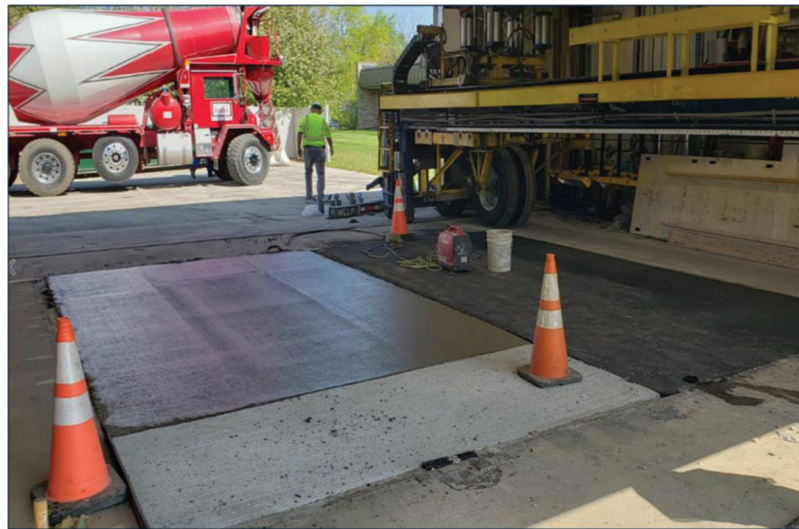
Figure 5.19 Rigid pavement test section after construction.
