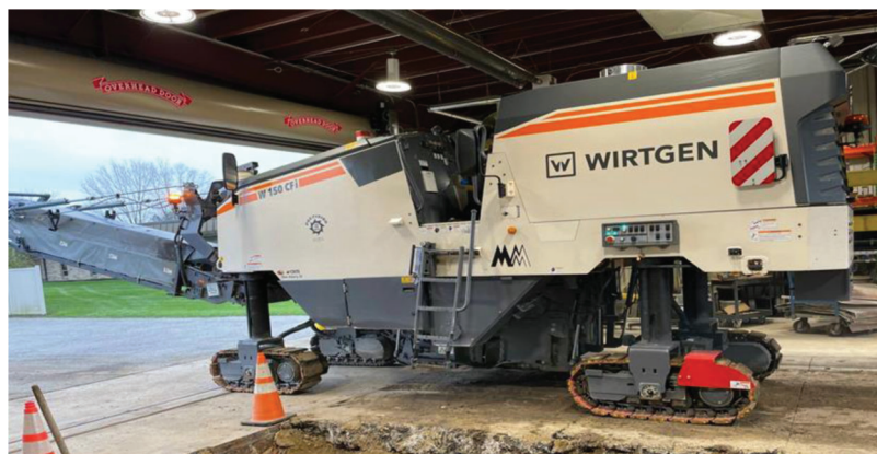
Figure 5.1 Milling machine used to mill the existing asphalt section.
