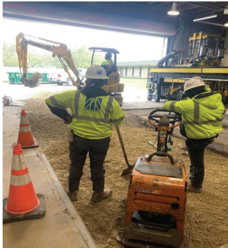
Figure 5.13 Plate compactor used to stabilize aggregate.
