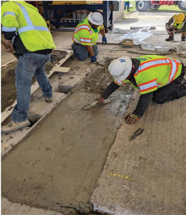
Figure 5.6 Placement of coils over concrete.
