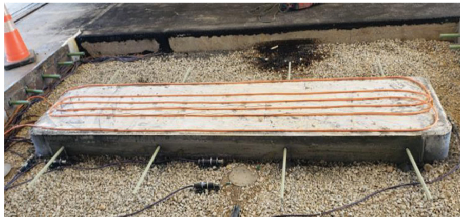
Figure 5.17 DWPT unit made of magnetizable concrete.
