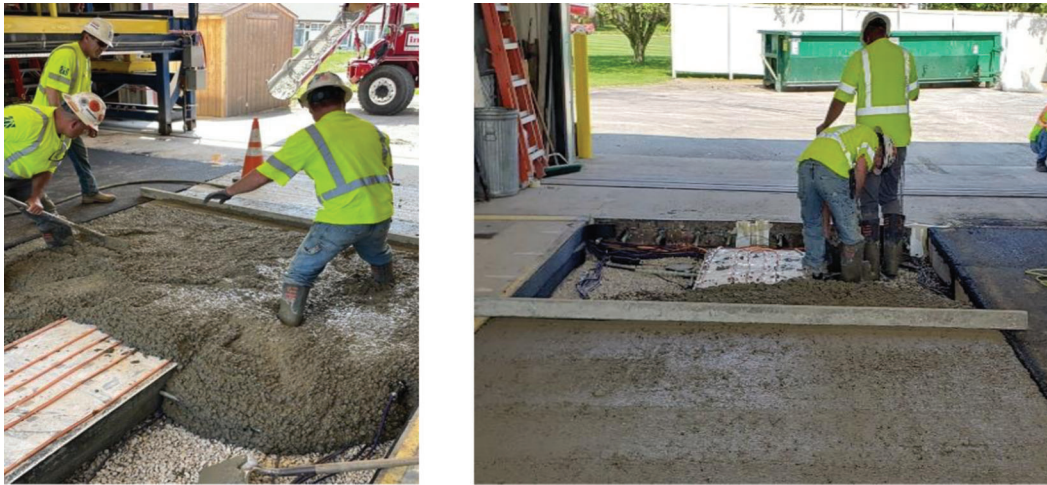
Figure 5.18 Class A concrete placement.
