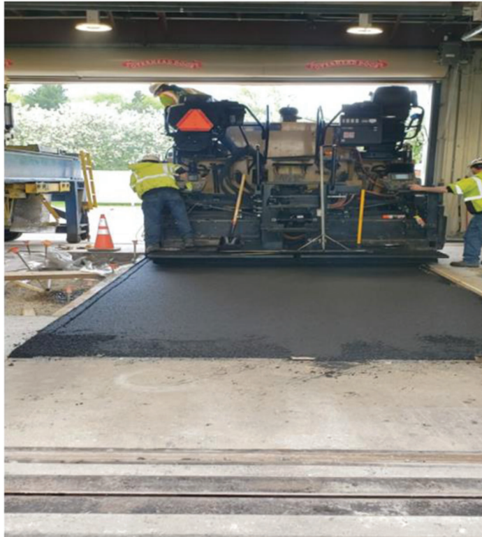
Figure 5.8 Placement of 2-in. HMA surface using asphalt paver.
