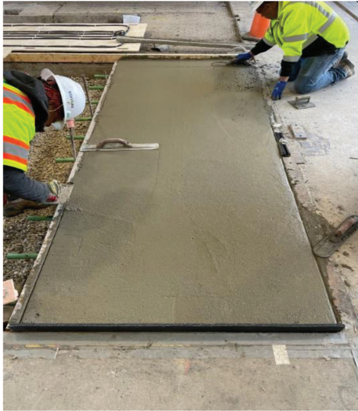
Figure 5.16 Class A concrete poured into joint.
