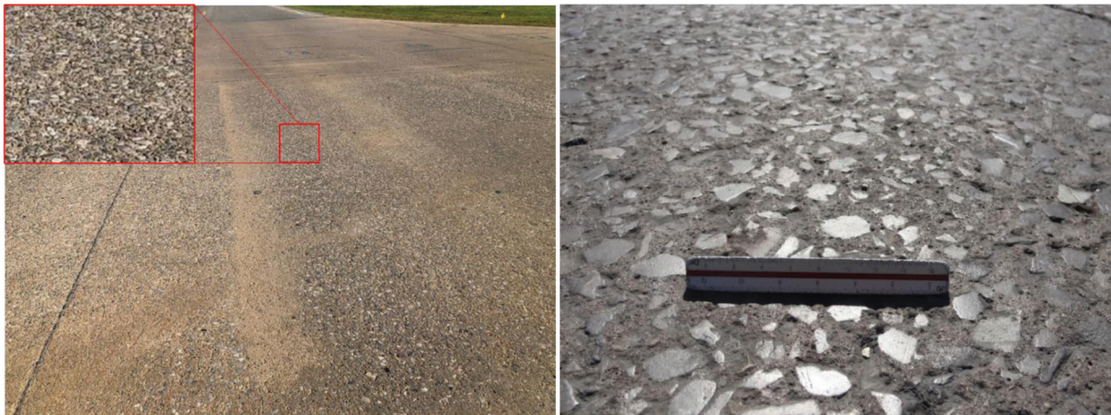
Examples of polished aggregate on the PCC pavement (© Photos by Applied Pavement Technology (APTech)).
