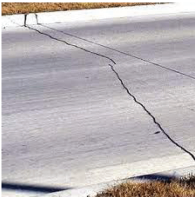
Sealed transverse crack on concrete pavement (Texas Transportation Institute, 2008).
