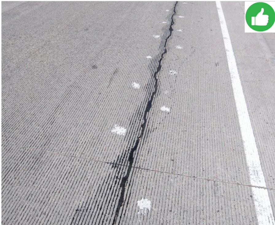
Well-sealed longitudinal crack repaired by cross-stitching (ACPA, n.d.).
