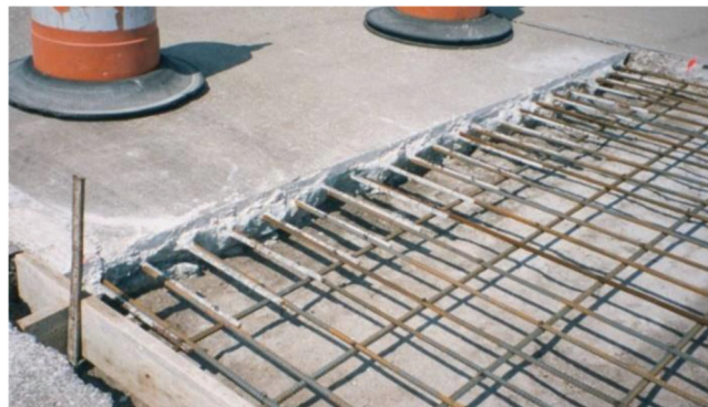
Restoration of both longitudinal and transverse steel in a CRCP FDP project (Step 5) (© Photo by Applied Pavement Technology (APTech)).
