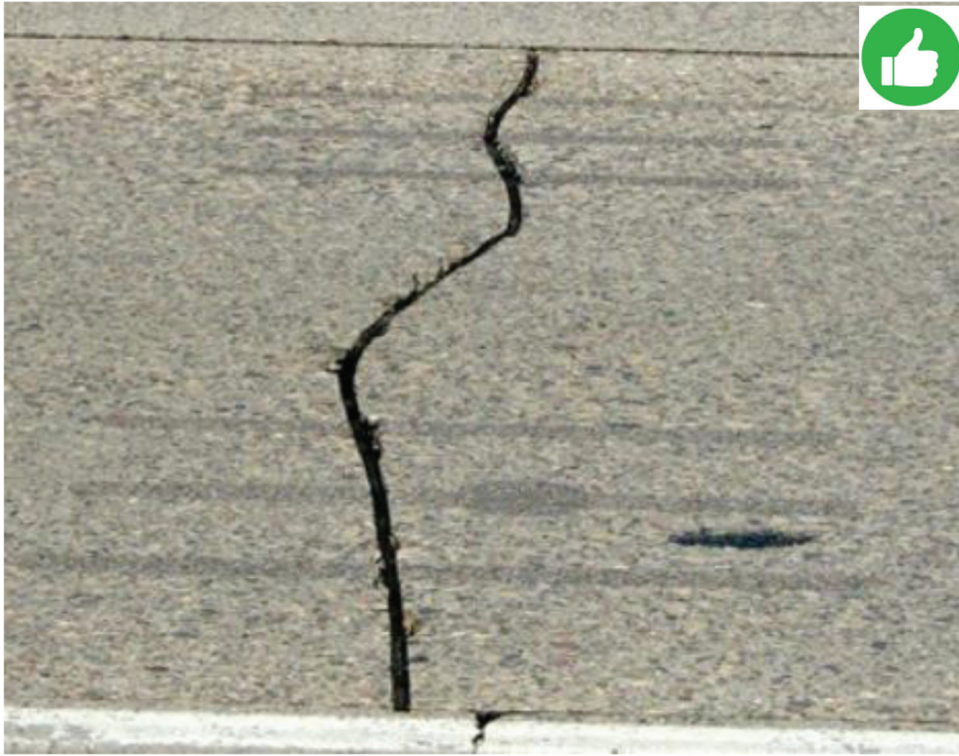
Crack sealing and retrofit load transfer across a moderate-severity transverse crack (Smith et al., 2022).
