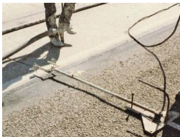
Mechanical methods of monitoring slab uplift using cement grout injection (Smith et al., 2022).
