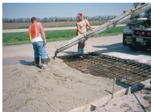
Placement (Step 7) of concrete pavement for FDP implementation for a CRCP (© Photo by Applied Pavement Technology (APTech)).
