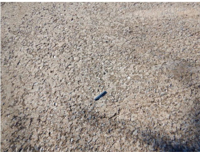
Scaling of concrete pavement (© Photo by Applied Pavement Technology (APTech)).
