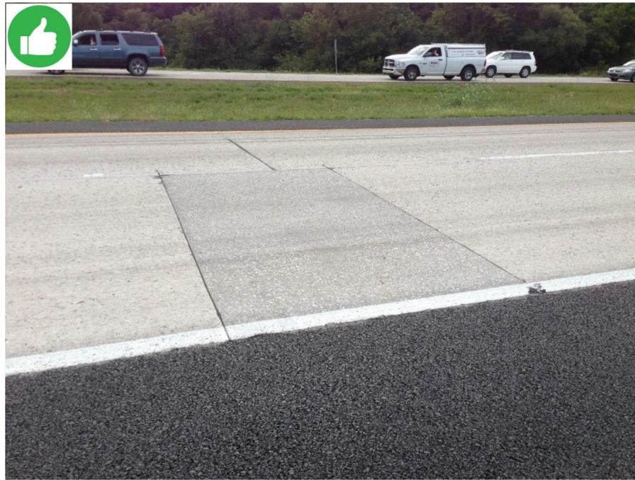
Properly installed full depth patch and associated joints (© Photo by Applied Pavement Technology (APTech)).
