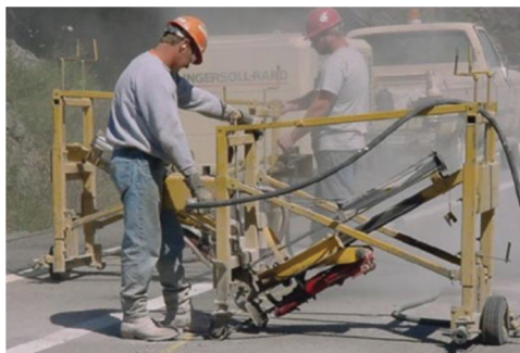
Drilling holes for cross-stitching (Step 1) (Smith et al., 2022).
