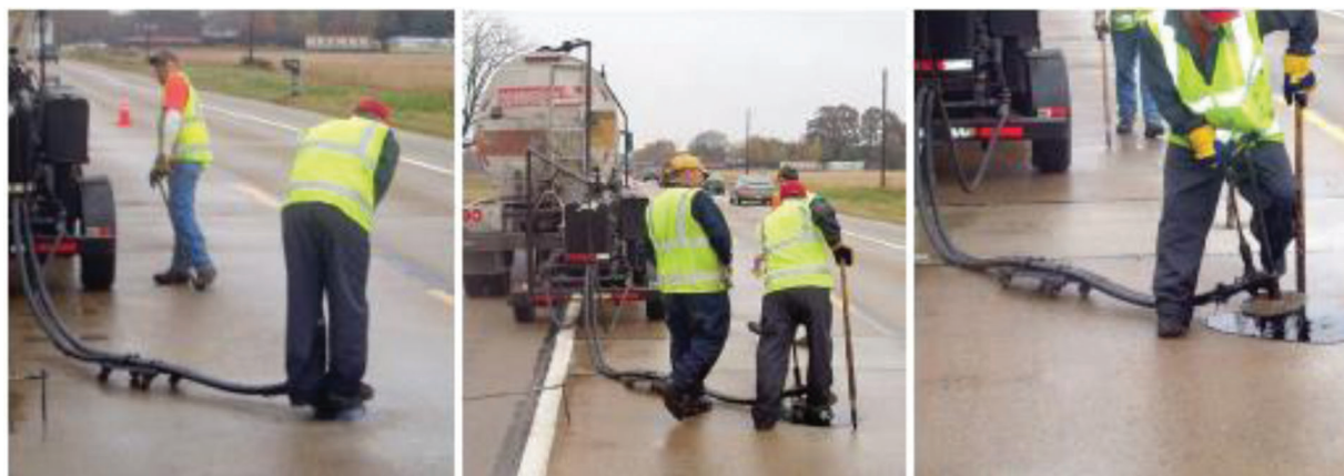
Injection of asphalt undersealing material (Smith et al., 2022).
