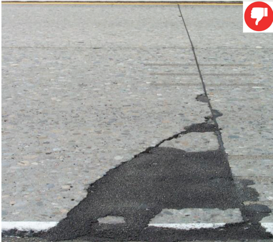
Improper use of asphalt mix patch to repair corner break (© Photo by Applied Pavement Technology (APTech)).
