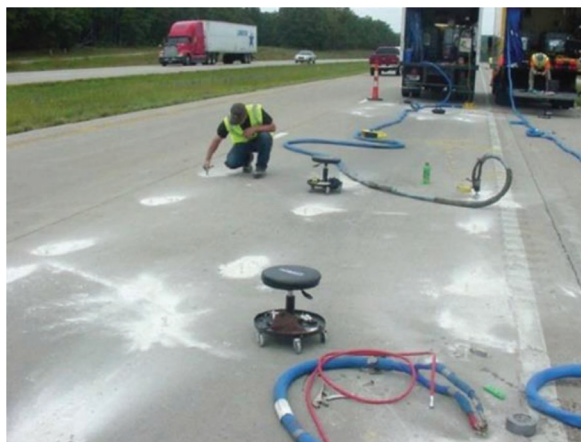
Polyurethane stabilization hole pattern (Smith et al., 2022).
