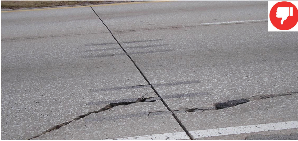
Cracks in the pavement leading to deterioration of grout in the RTL (© Photo by Applied Pavement Technology (APTech)).
