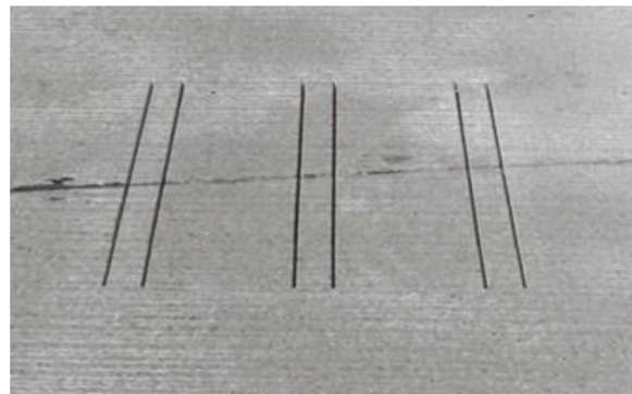
Slot creation (Step 2) of concrete pavement (Photo from J. Uhlmeier, personal communication, May 14, 2024.)
