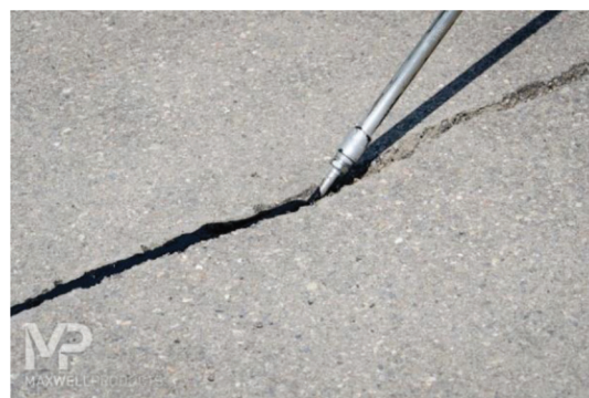
Sealing (Step 4) of a crack in concrete pavement using polymer binder (Maxwell Products, n.d.).
