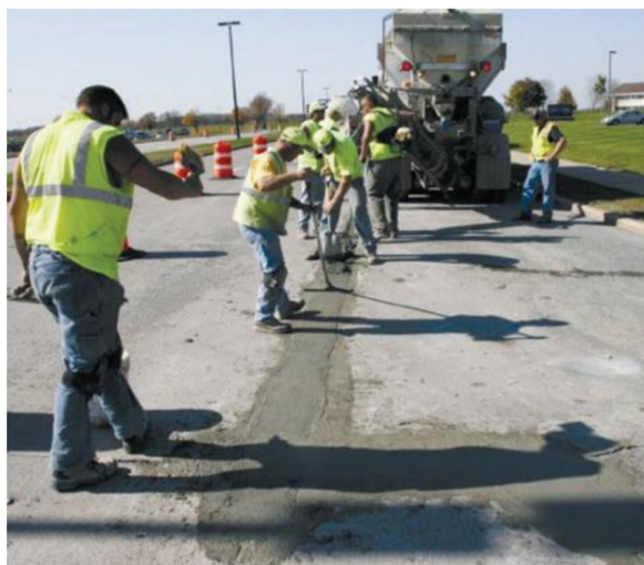
Placement of PDP material for longitudinal joints using mobile concrete truck (Step 6) (Smith et al., 2022).
