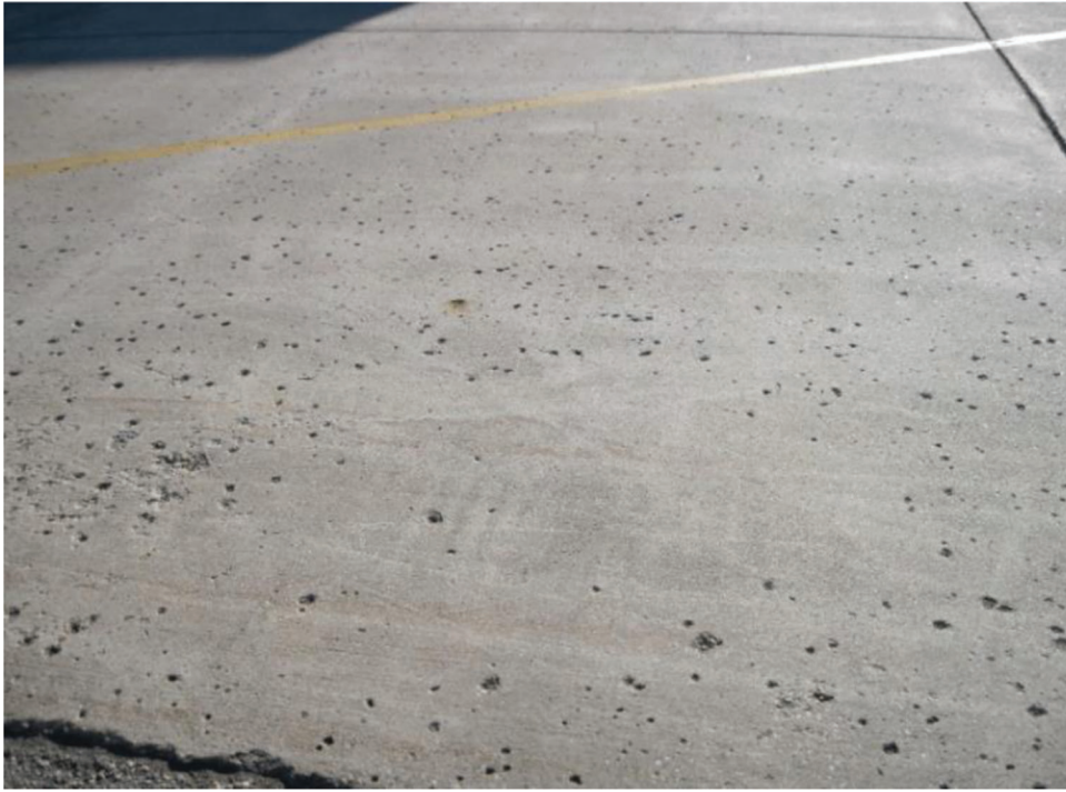
Extensive popouts (i.e., density \geq 3 popouts/yd 2 ) on a PCC pavement (© Photo by Applied Pavement Technology (APTech)).
