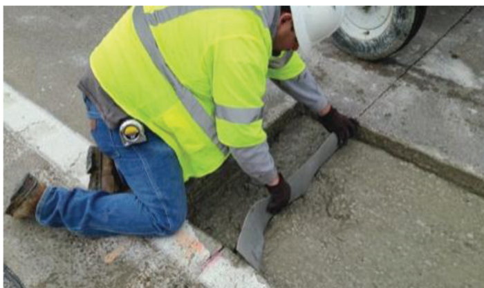
Placement of bond breaker on a PDP project (Step 4) (Smith et al., 2022).
