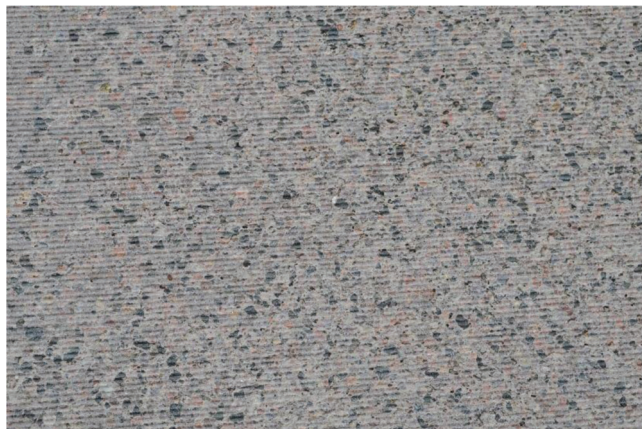
A close view of a uniformly diamond-ground surface of a concrete pavement (© Photo by Applied Pavement Technology (APTech)).
