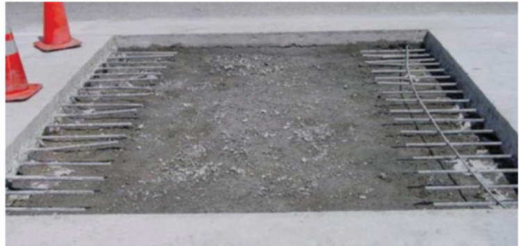
Prepared CRCP repair area (Step 4) with exposed reinforcing steel (Smith et al., 2022).
