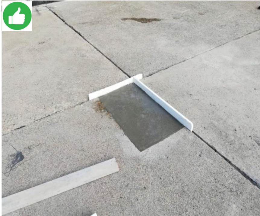
Properly installed PDP to repair spalling of the transverse joint (Rodeco Group, n.d.).
