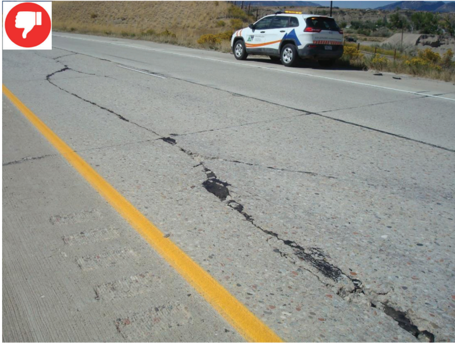
Poorly sealed longitudinal crack (© Photo by Applied Pavement Technology (APTech)).
