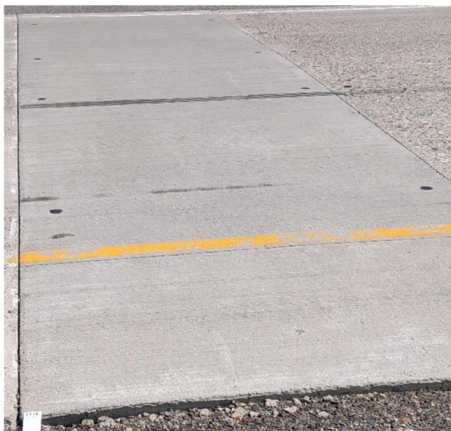
Completed concrete full depth patch on a concrete pavement (© Photo by Applied Pavement Technology (APTech)).
