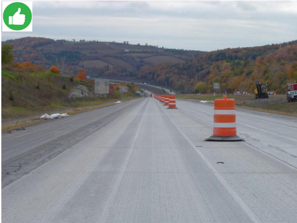
Example of proper diamond grinding to address faulting on JPC pavements (J. Roberts, personal communication, August 7, 2023).
