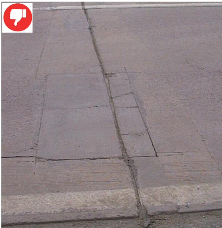
Deteriorated PDP (© Photo by Applied Pavement Technology (APTech)).
