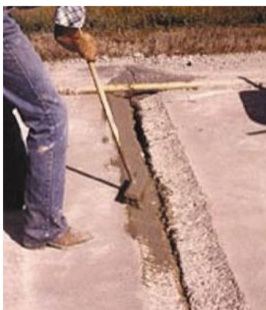
Application of cement grout as bonding agent (Step 5) (Smith et al., 2022).
