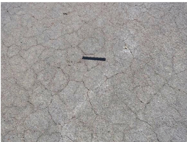
Map cracking on PCC pavement (© Photo by Applied Pavement Technology (APTech)).
