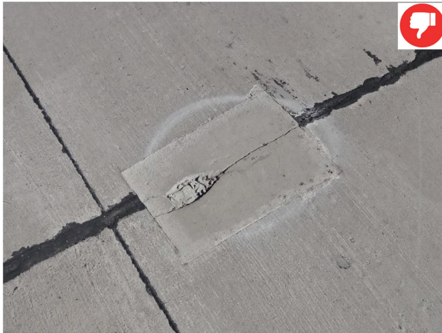
PDP installed without proper joint preparation (© Photo by Applied Pavement Technology (APTech)).
