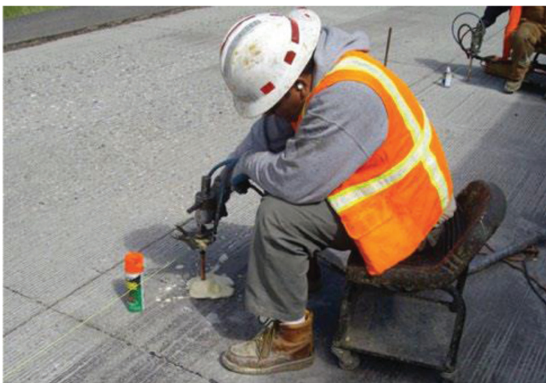
Injecting polyurethane for slab stabilization (Smith et al., 2022).
