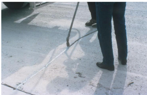
Sealing of a transverse joint in concrete pavement (Part A Step 4 Construction Steps) (© Photo by Applied Pavement Technology (APTech)).
