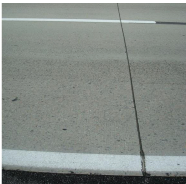
Sealed contraction joint on concrete pavement (© Photo by Applied Pavement Technology (APTech)).
