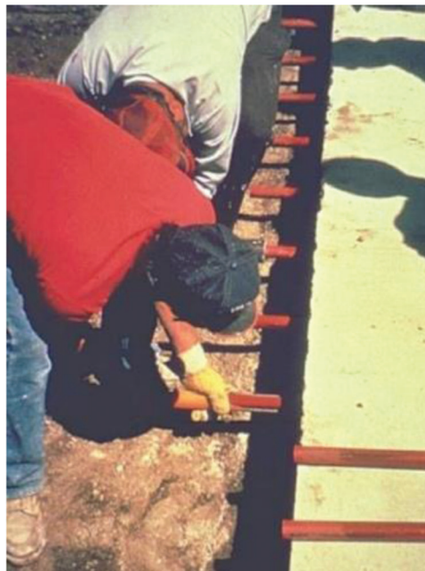
Installation of dowel bar (load transfer) (Step 5) in FDP implementation on a JPCP (© Photo by Applied Pavement Technology (APTech)).
