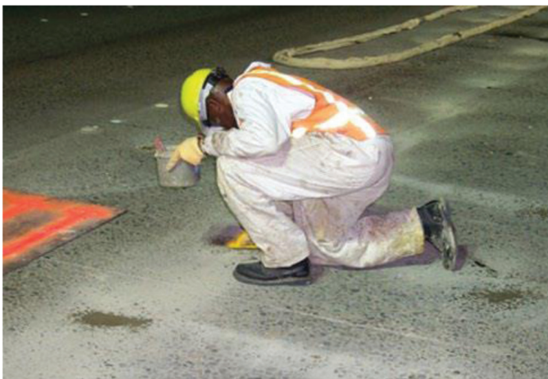
Patching drill holes after removal of temporary plug-in cement grout slab
