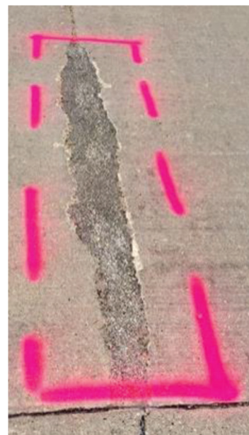
Properly marked PDP area (Step 1) (Smith et al., 2022).
