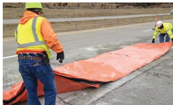
Insulating blanket being placed on finished PDP in cold weather conditions (Step 9) (Smith et al., 2022).
