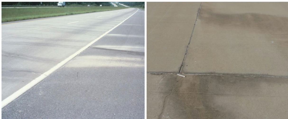
Example of water bleeding and pumping on CRCP (left) and JPCP (right) (© Photos by Applied Pavement Technology (APTech)).
