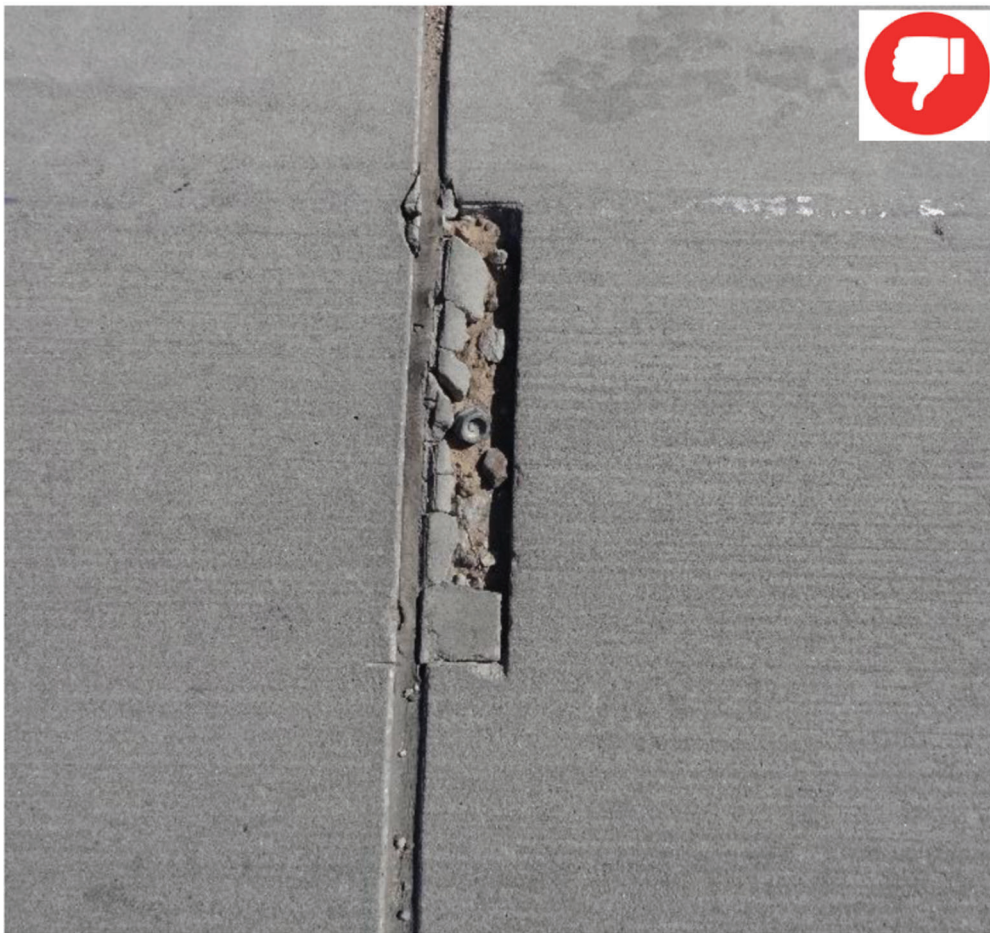
Failed PDP that was used to address joint spalling (© Photos by Applied Pavement Technology (APTech)).
