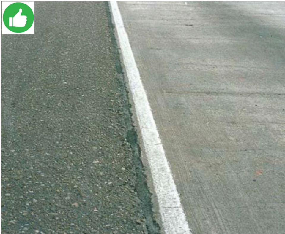
Effective sealing of the shoulder-lane joint (FHWA, 2014).
