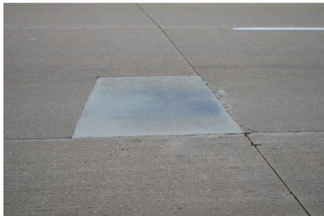
Completed concrete partial depth patch at the corner of a concrete slab (© Photo by Applied Pavement Technology (APTech)).
