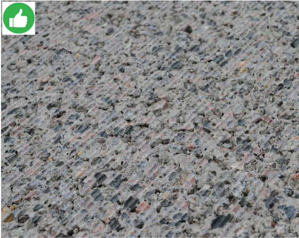
A close-up view of a diamond ground concrete pavement surface (© Photo by Applied Pavement Technology (APTech)).
