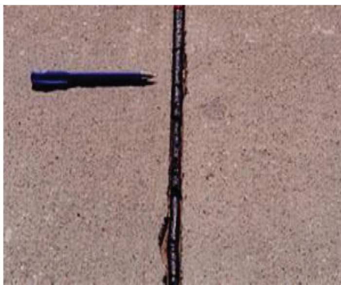
Joint seal damage (INDOT Office of Aviation, 2022c).
