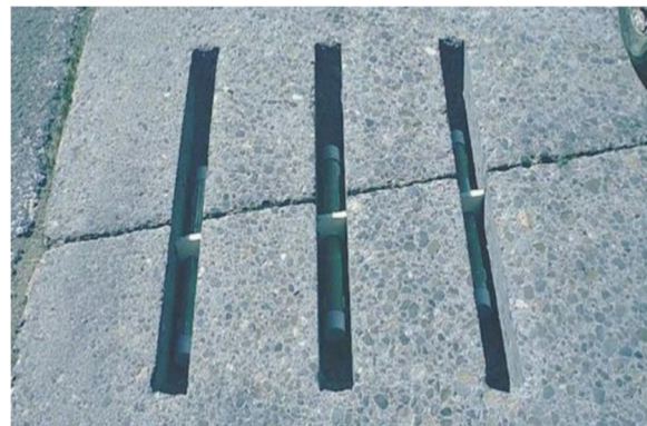
Dowel bar placement (Step 6) into the slots (Photo from J. Uhlmeier, personal communication, May 14, 2024).
