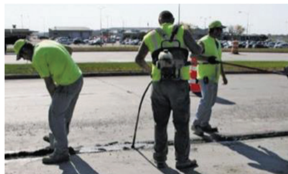
Consolidation of PDP material using small-head vibrator (Step 7) (Smith et al., 2022).
