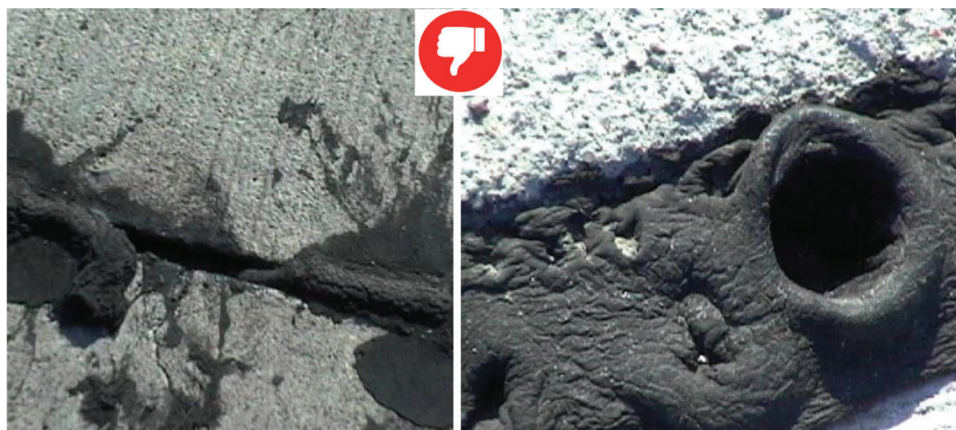
Improperly installed joint sealant (voids and discontinuities in the sealant material) (© Photos by Applied Pavement Technology (APTech)).
