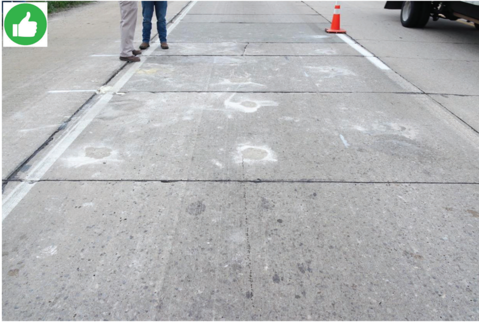
Appropriately completed undersealing using polyurethane foam (T. Nantung, personal communication, August 14, 2023).
