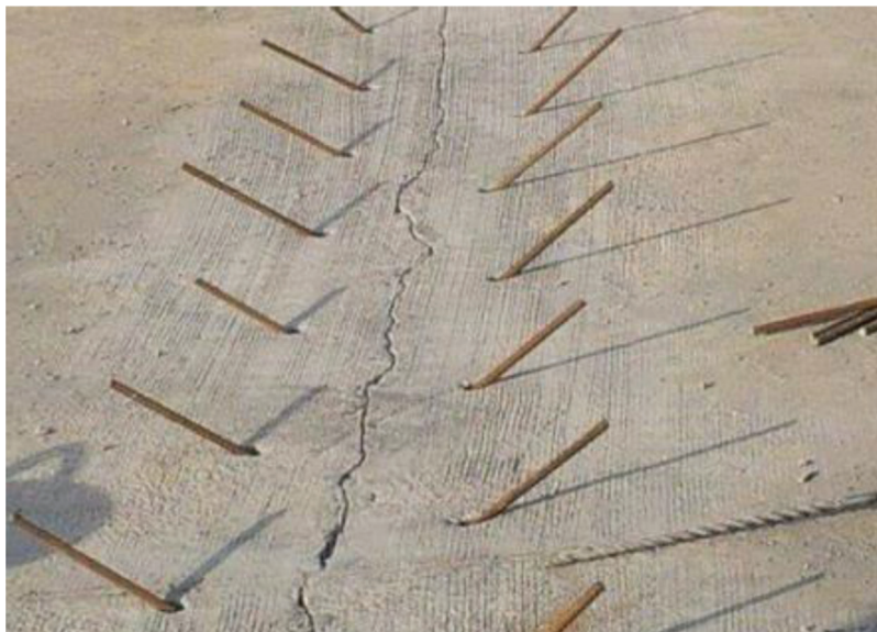
Implementation of a cross-stitching method to repair a longitudinal crack (Daily Civil, n.d.).
