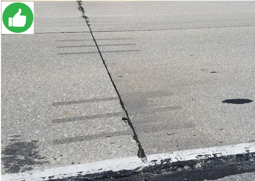
An RTL (Retrofit Load Transfer) device installed on a faulted joint of a PCCP (© Photo by Applied Pavement Technology (APTech)).
