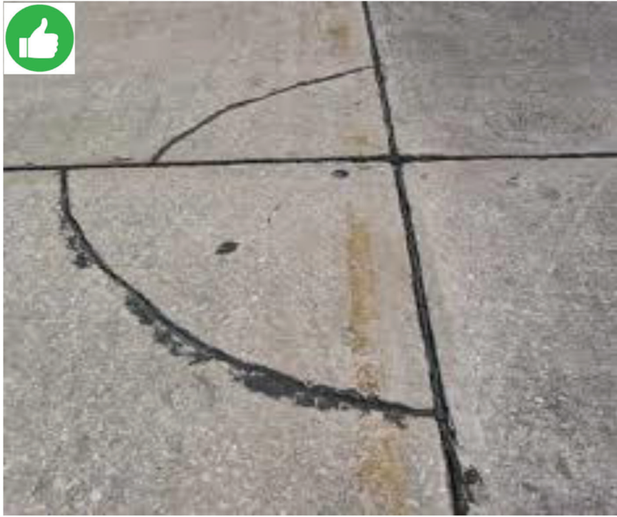
Sealed low-severity corner break (© Photo by Applied Pavement Technology (APTech)).
