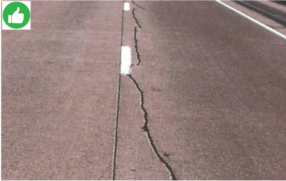
Properly sealed longitudinal crack with moderate severity (© Photo by Applied Pavement Technology (APTech)).
