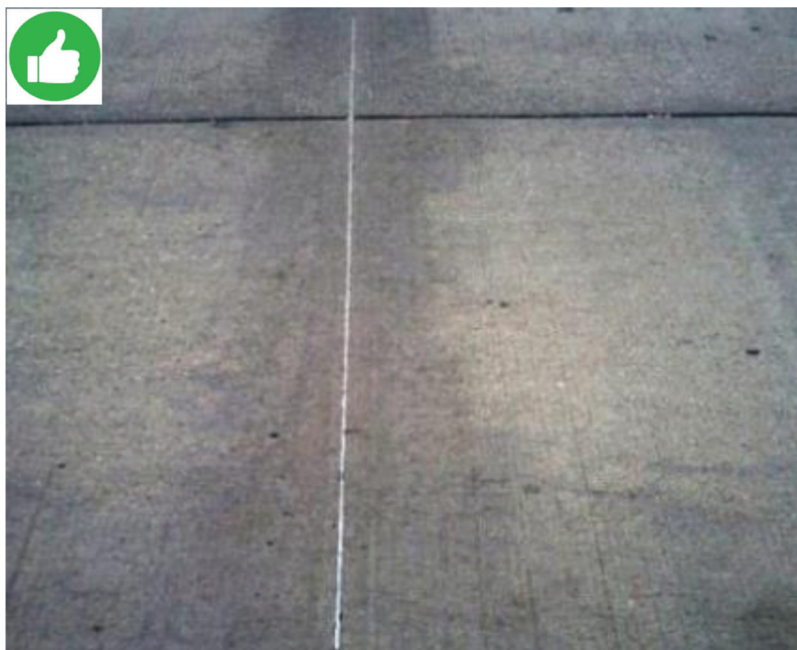
A well-sealed joint that helps reduce the ingress of moisture which may exacerbate “D” cracking (Zhang, 2013).
