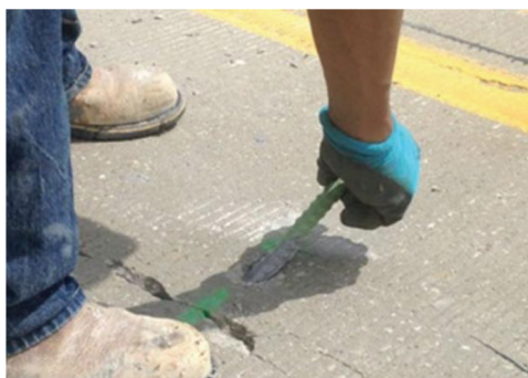
Inserting a tie bar into a drilled hole (Step 4) (Smith et al., 2022).
