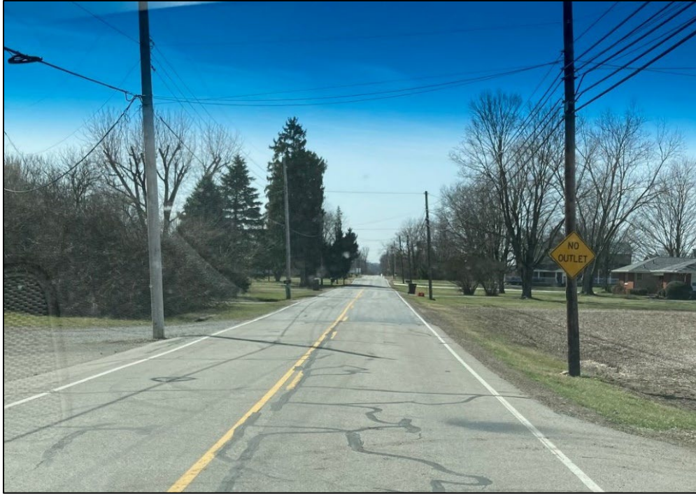
Figure B-2. Photo of Lower Valley Pike Test Site
