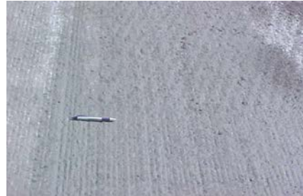
Surface after Milling and Cleaning
