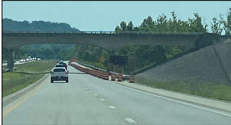
Figure 3.2 Right Lane Closure on Interstate Pavement Rehabilitation Project
