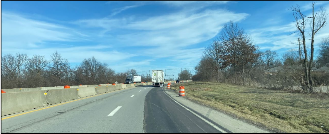
Figure 2.1 Temporary Asphalt Pavement on Outside Shoulder on Multi-Lane Divided Highway Project
