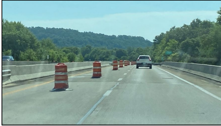
Figure 3.4 Lane Shift on an Interstate Pavement Rehabilitation Project
