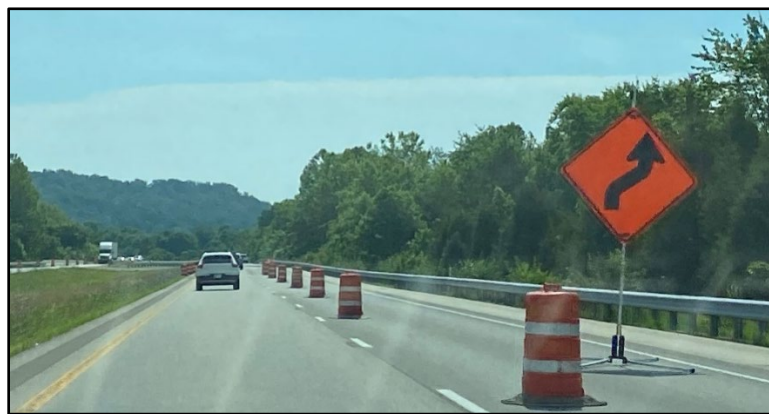
Figure 3.3 Approaching a Lane Shift on Interstate Pavement Rehabilitation Project
