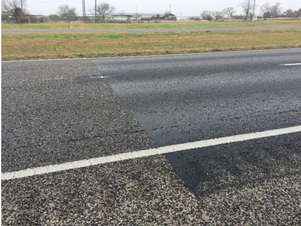
Figure 29. IH 35 after 3 years of traffic showing wear off the Onyx surface treatment.
