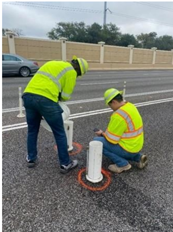
Figure 121. Water flow testing on MoPac.
