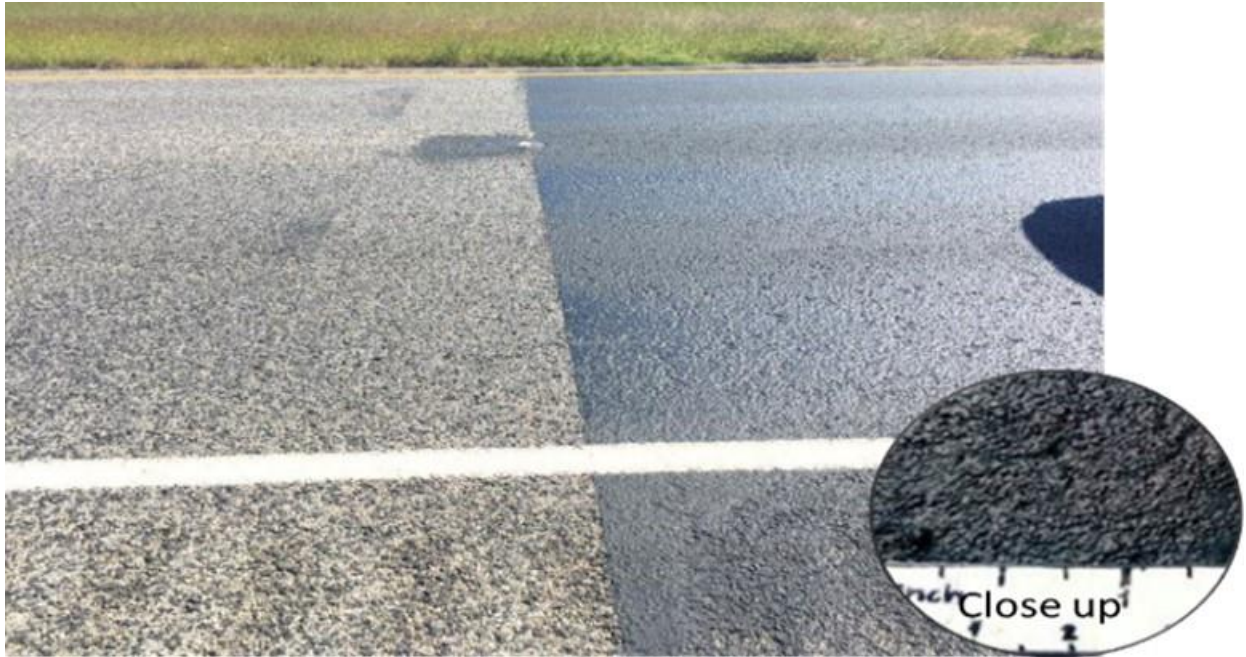
Figure 27. IH 35 existing PFC and beginning of Onyx application.
