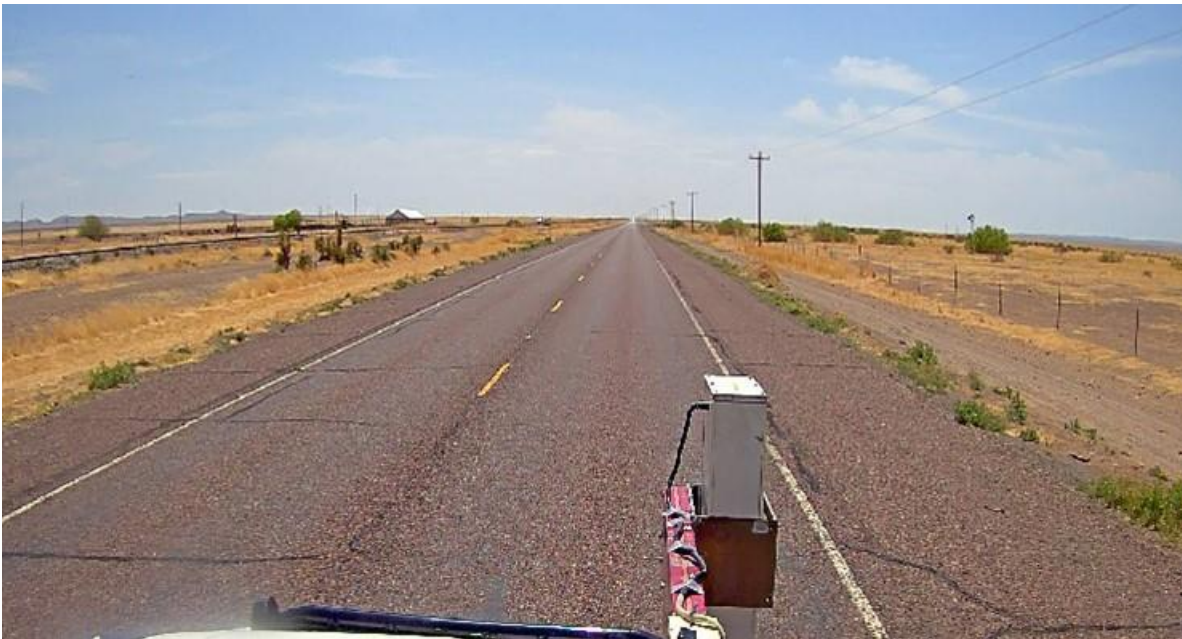
Figure 42. Current condition of US 90 at western end of project near Presidio County Line (April 2022).
