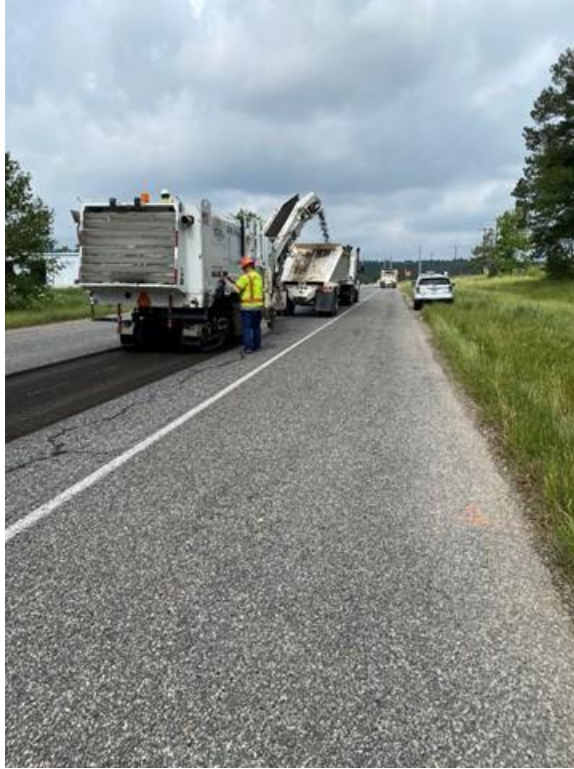
Figure 100. Milling the old surface to provide smooth transition to new overlay.
