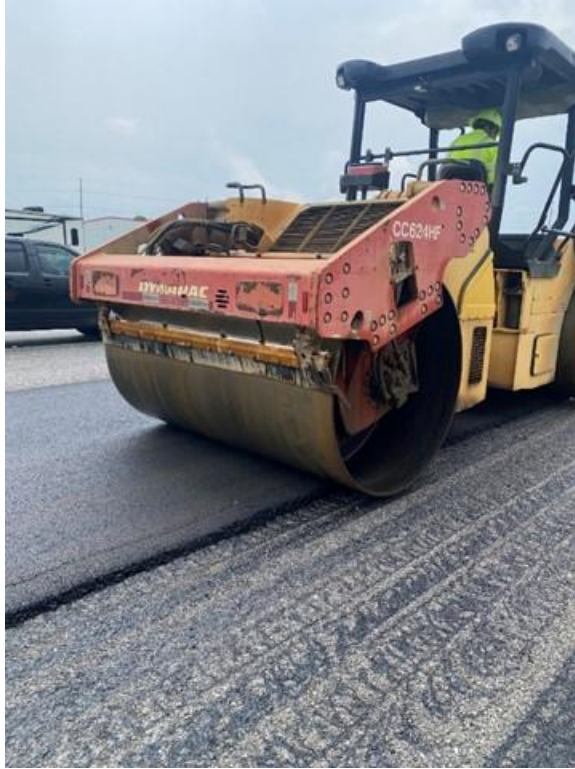
Figure 107. Additional static rolling on the problem areas after mat cooled down.
