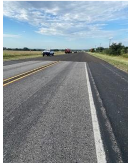
Figure 6. Seal coat application on PFC.
