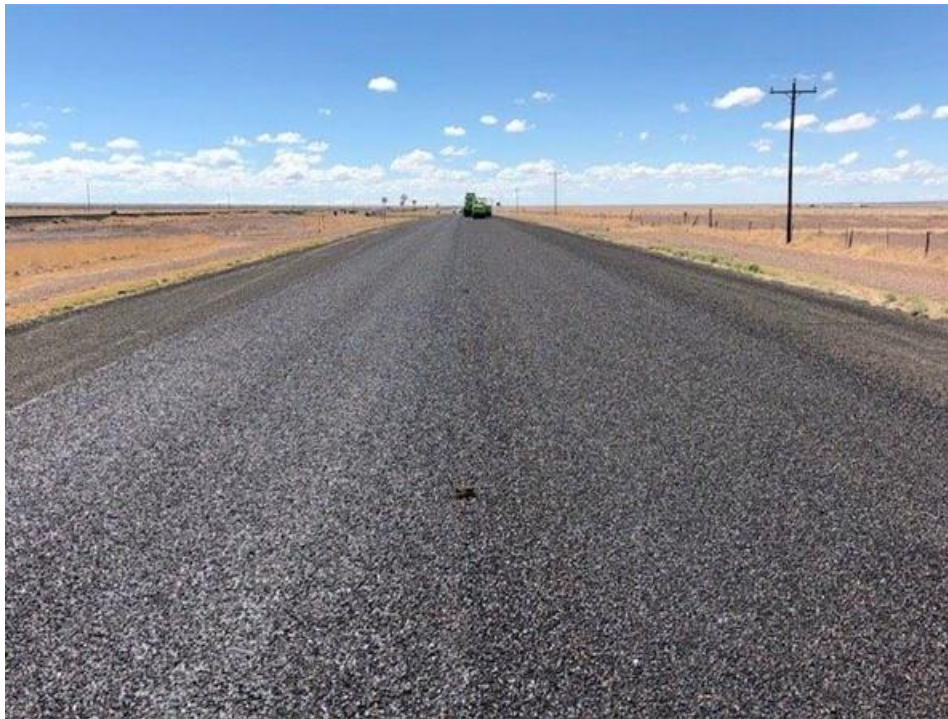
Figure 40. Seal coat construction on US 90 in El Paso District.
