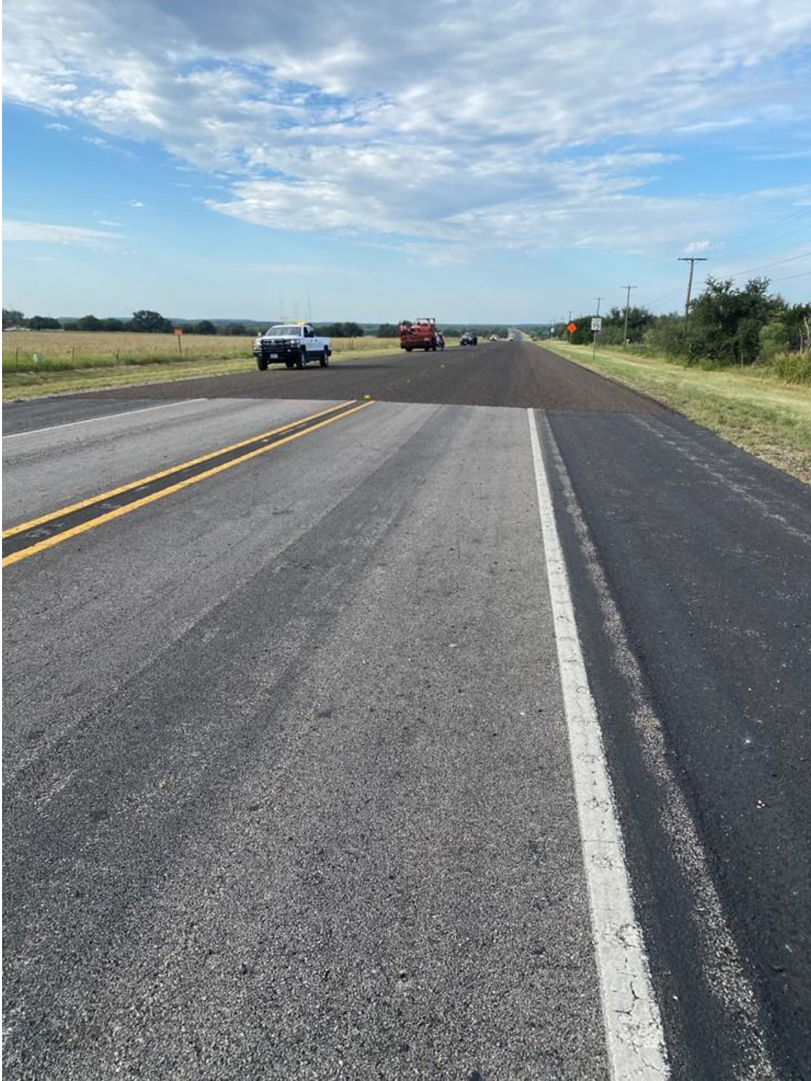
Figure 120. View of seal coat and PFC surface.
