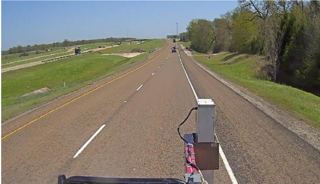
Figure 44. Current condition of SH 6 FR (April 2022).
