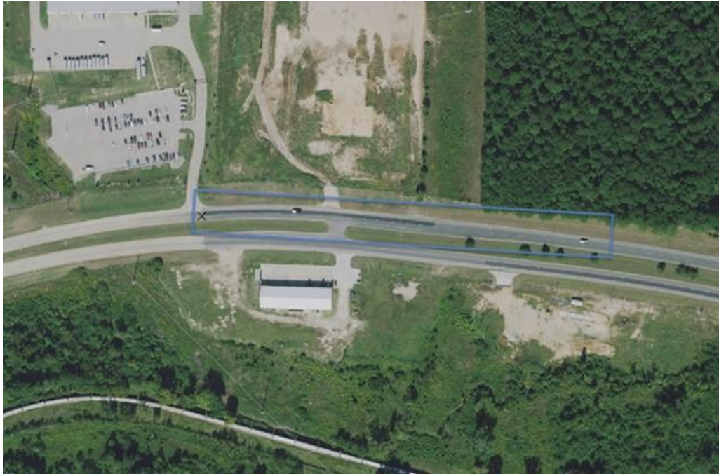
Figure 52. Image of test section location on US 69 Lufkin.
