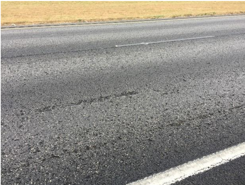
Figure 30. IH 35 after 3 years of traffic showing signs of raveling.
