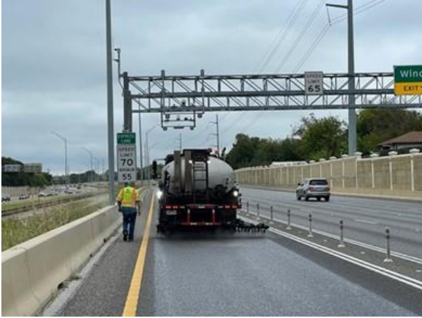
Figure 5. Rejuvenating fog seal application on PFC.
