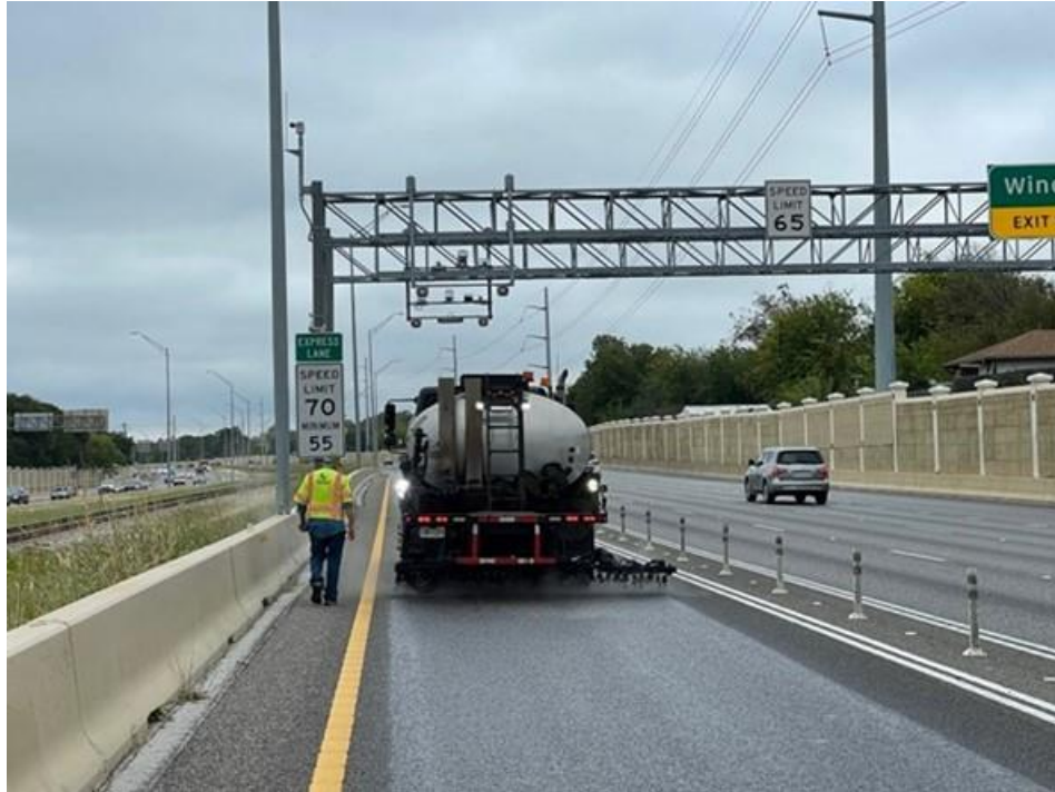
Figure 124. Construction of fog seal on MoPac.
