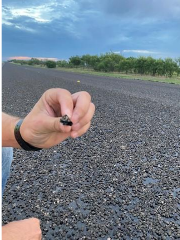
Figure 115. Initial embedment after rolling.
