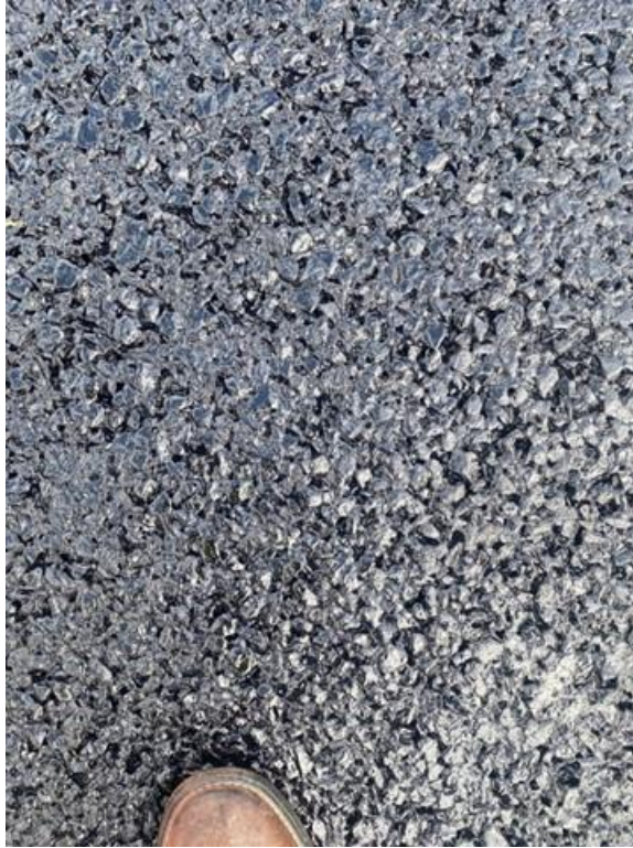
Figure 125. Close-up of fog seal application on PFC.
