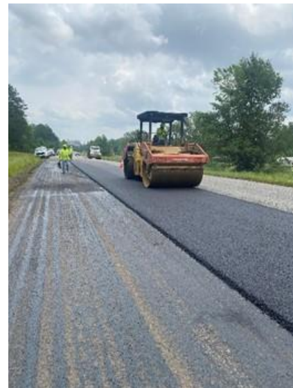
Figure 7. Hot-mix application on PFC.
