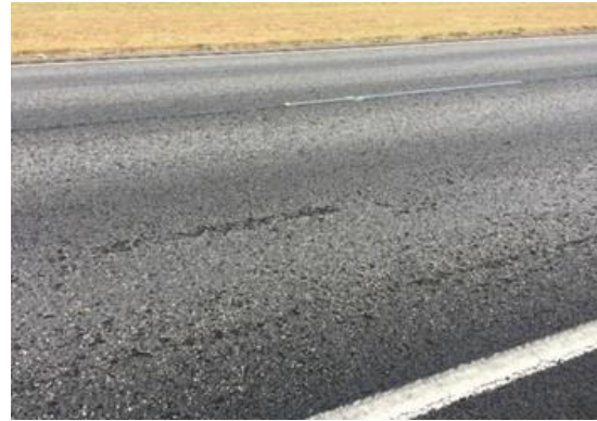
Figure 1. Raveling distress in aged PFC.
