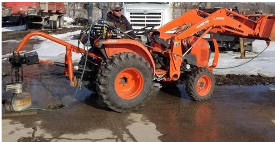
Figure 12. Equipment used to obtain 16-inch diameter cores from the PFC pavement.
