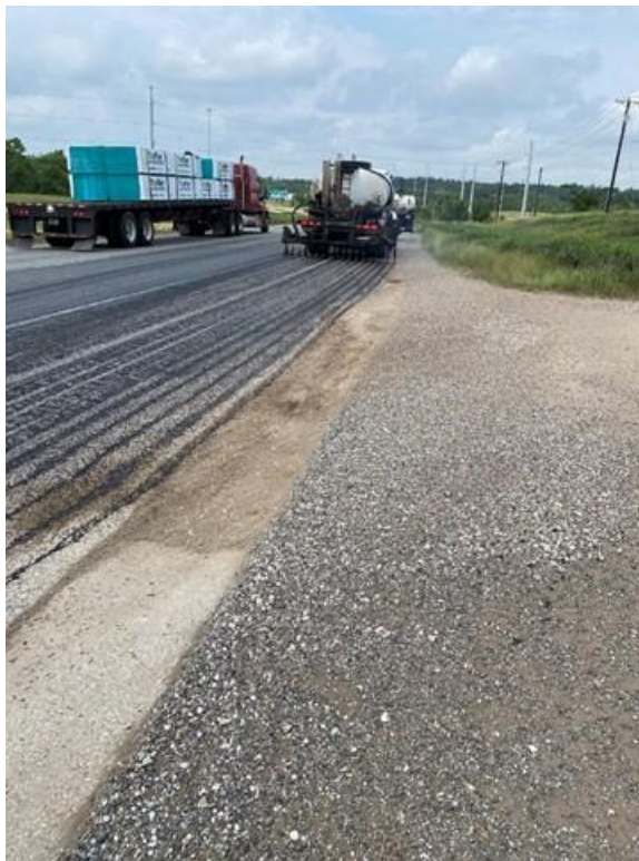
Figure 101. Non-tracking tack coat applied first to travel lane and then shoulder.
