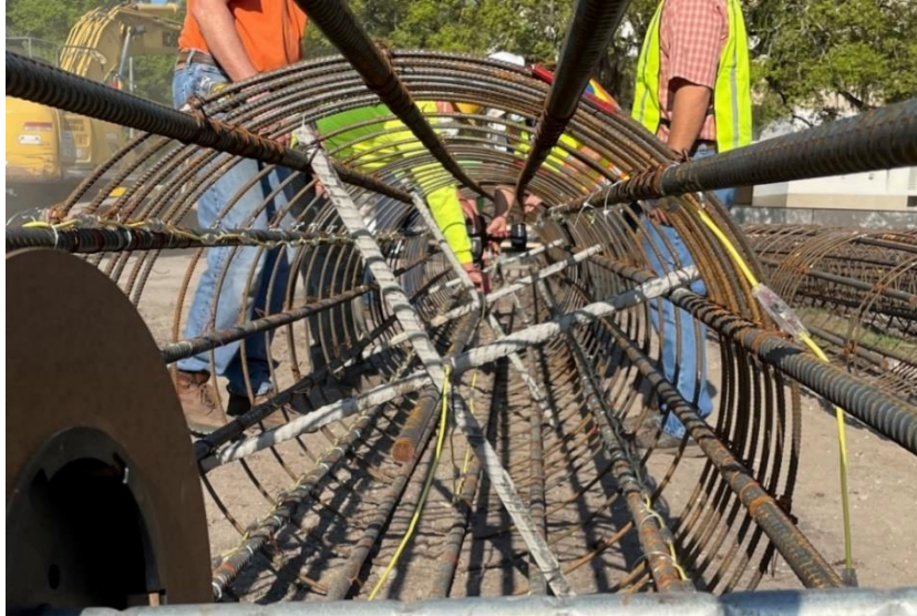
Figure 3.3 Installation of center wire along additional center rebar.
