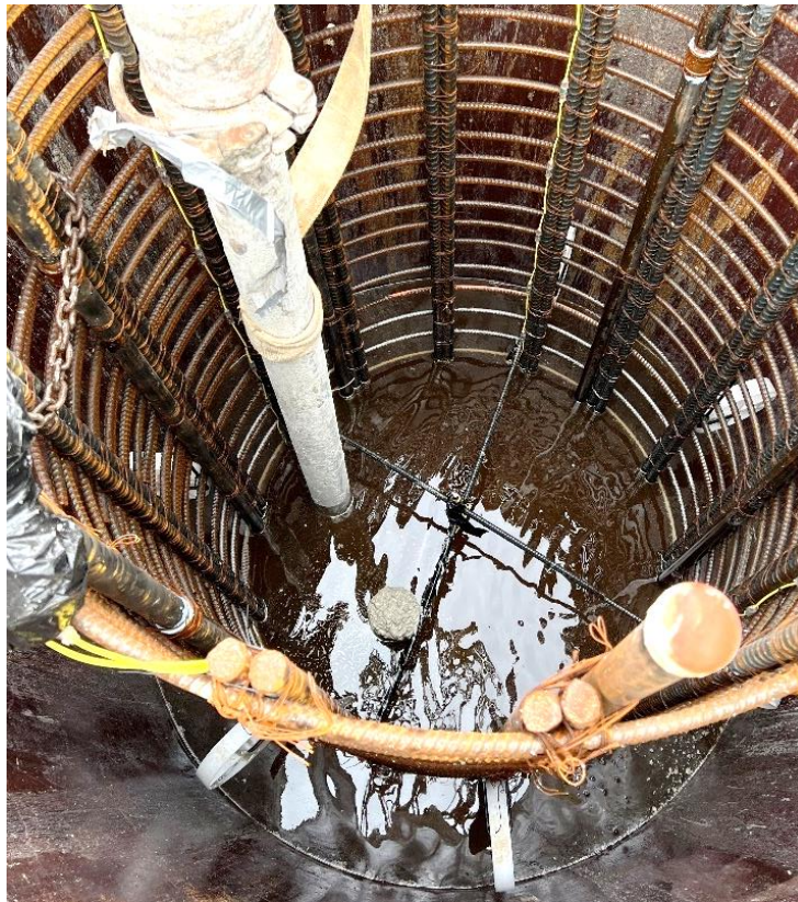
Figure 3.22 Tremie separation during OC-13 concrete placement.
