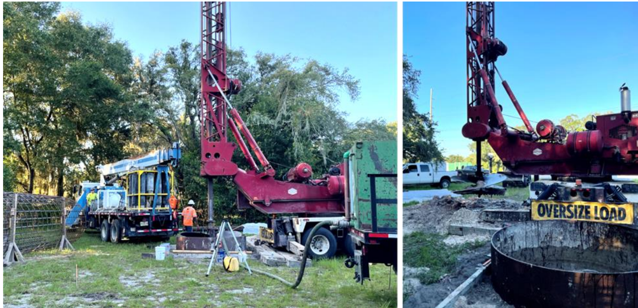
Figure 1.4 Drilled shaft excavation.
