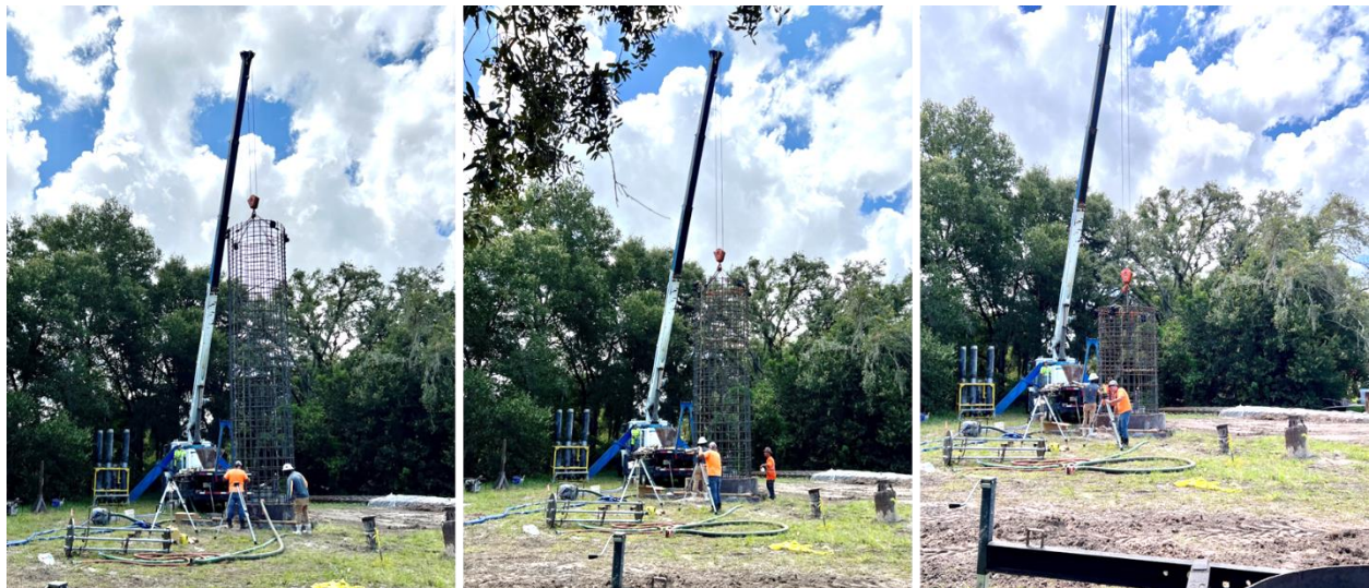
Figure 1.5 Drilled shaft reinforcement cage placement.
