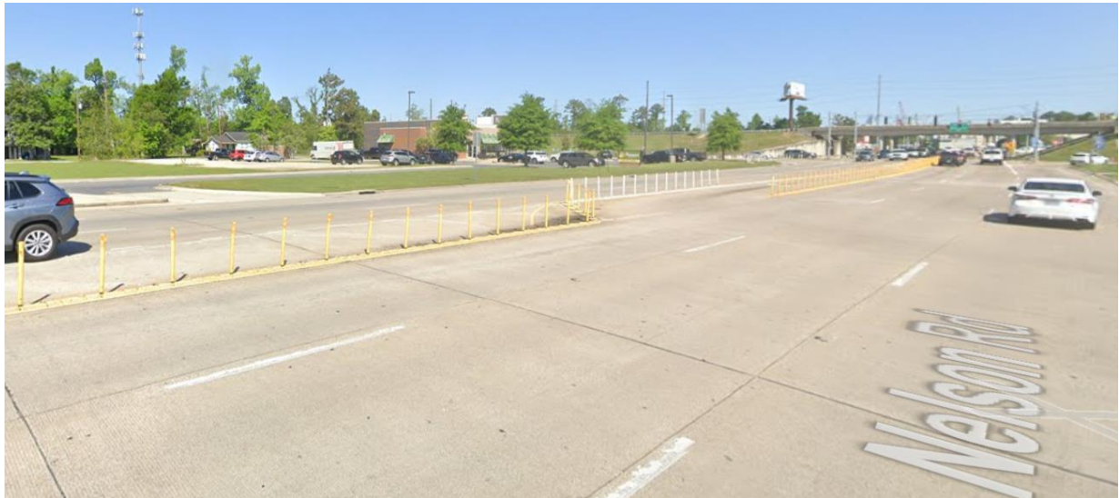
Figure 15. Raised Curb Channelization (Nelson Road - 30.195263, -93.249429) Post-Treatment
