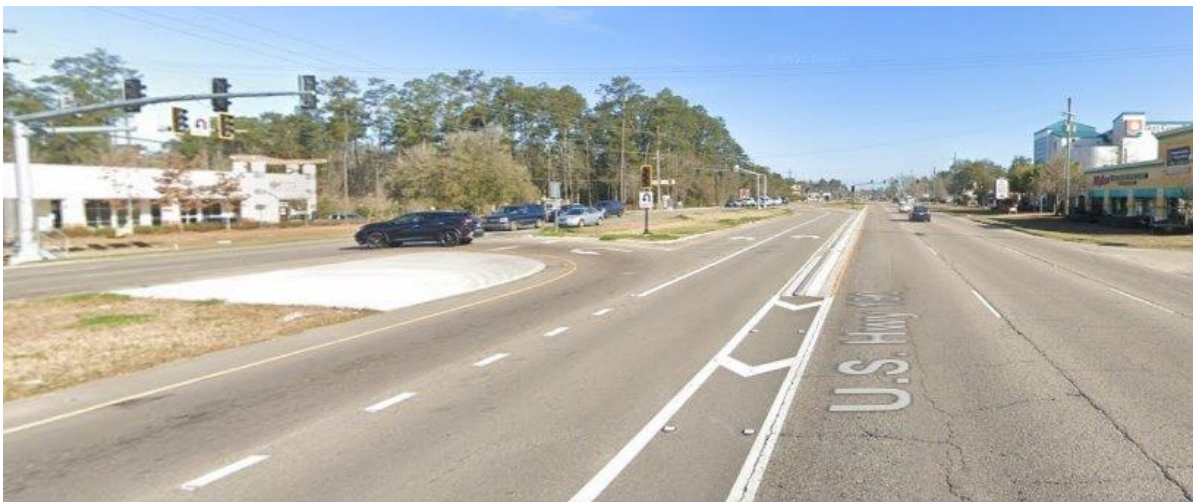
Figure 7. J Turn Installation (US 190/Tammany Pkwy - 30.447358, 90.082012) Post-Treatment
