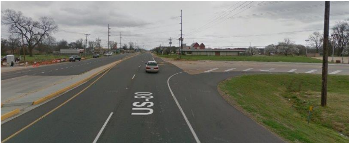
Figure 11. Right-in-Right-out Installation (East Texas Street / US 80 - 32.533706, -93.671444) Post-Treatment
