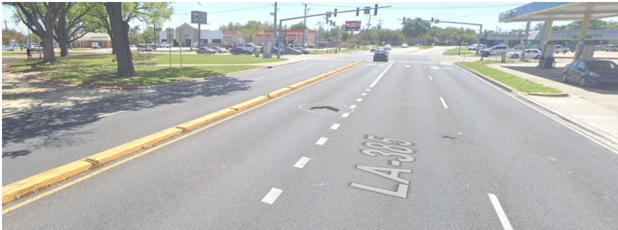
Figure 9. Raised Median (Ryan Street - 30.176669, -93.218558) Post-Treatment
