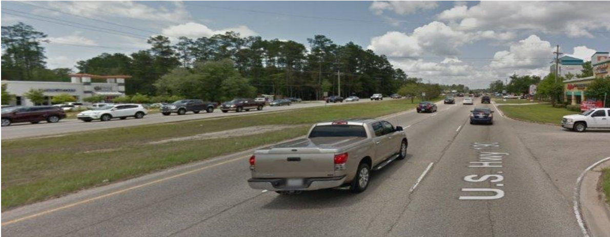
Figure 6. J Turn Installation (US 190/Tammany Pkwy - 30.447358, -90.082012) Pre-Treatment
