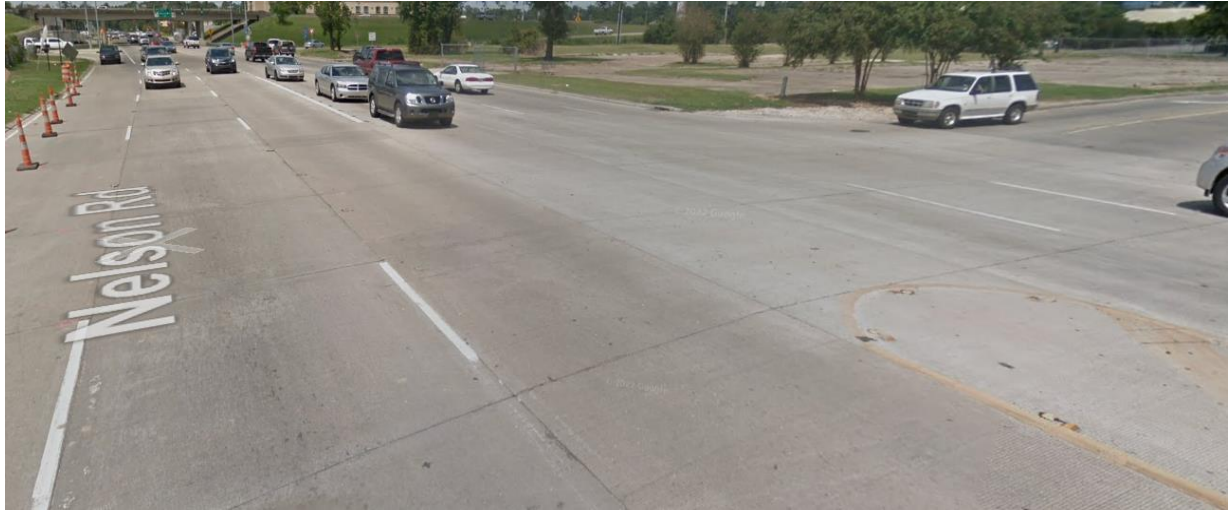
Figure 14. Raised Curb Channelization (Nelson Road - 30.195263, -93.249429) Pre-Treatment
