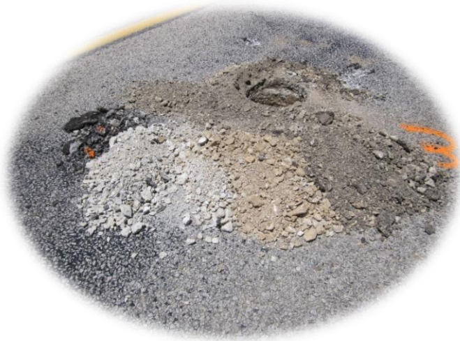
Material nonuniformity must be captured and considered in mix design
