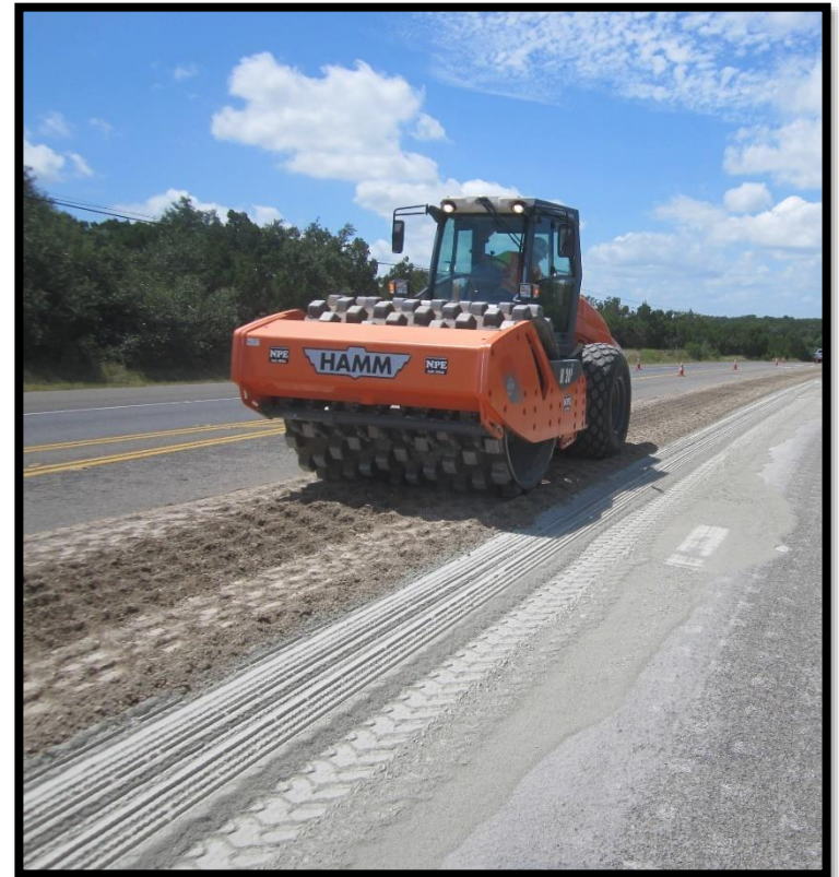
Compacting FDR mix
