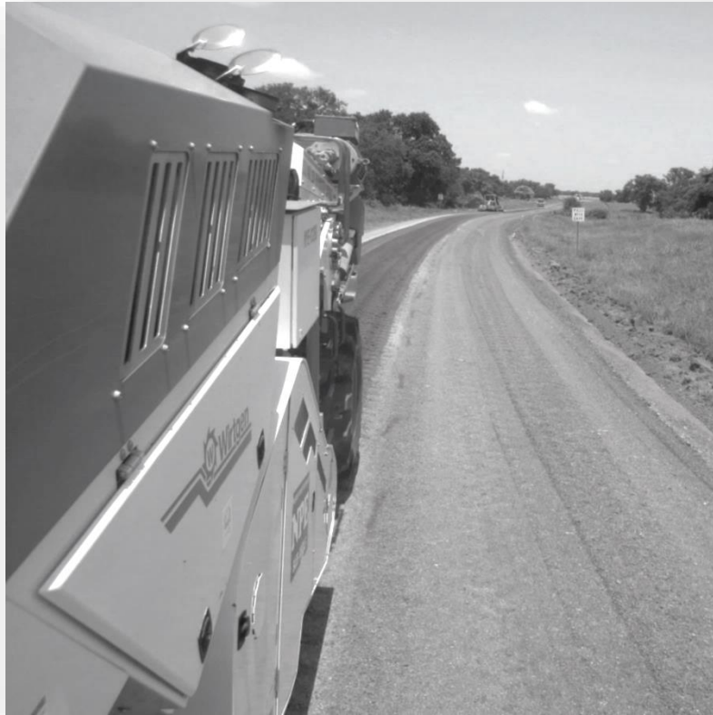
FDR in progress Must complete all 3 steps in 1 day
