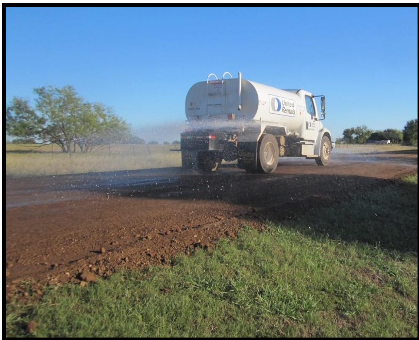
Sprinkling to preserve surface moisture during finishing
