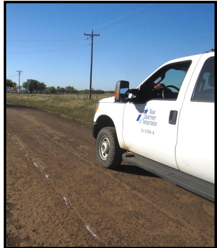
Painted cut line for reclaimer to follow
