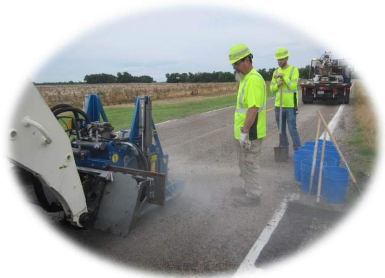
Generating sample for mix design
