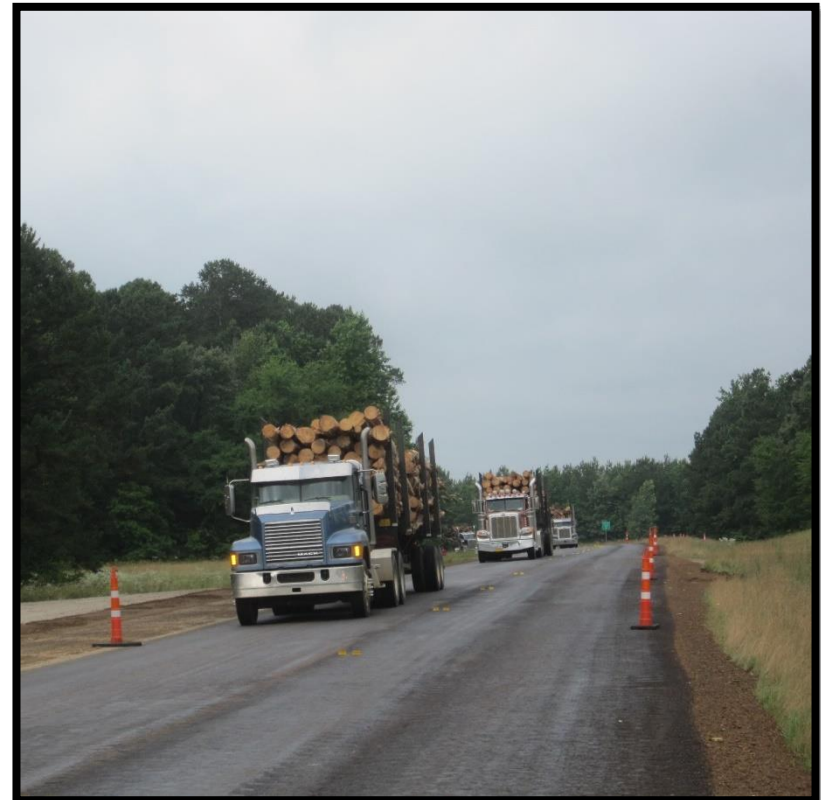
Truck traffic on FDR section (foam) with fog seal applied
