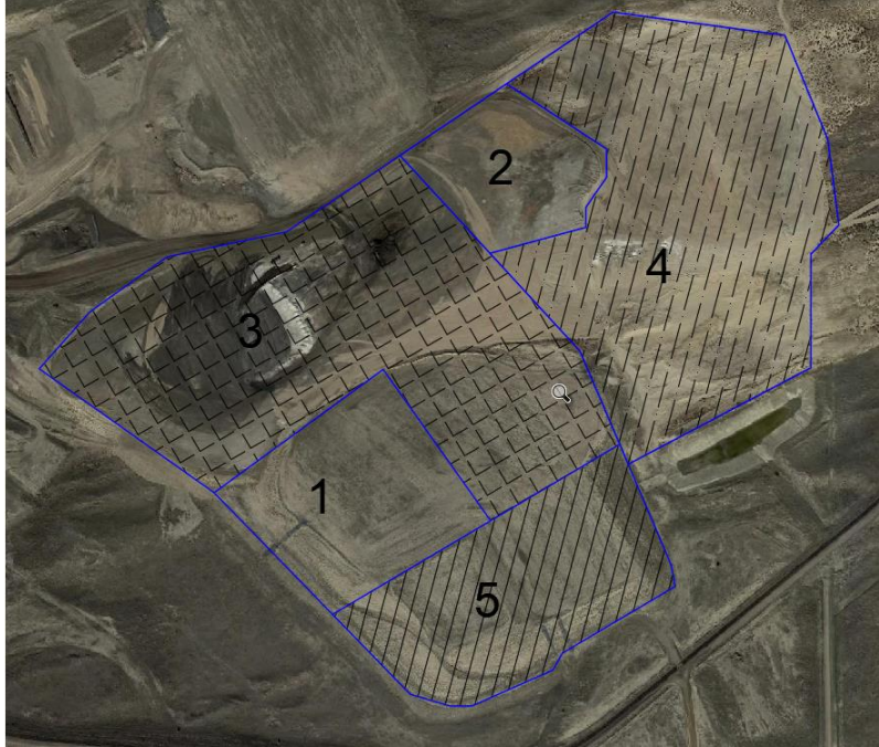
Figure 2.8 Expansion landfill at Dave Johnston Power Plant
