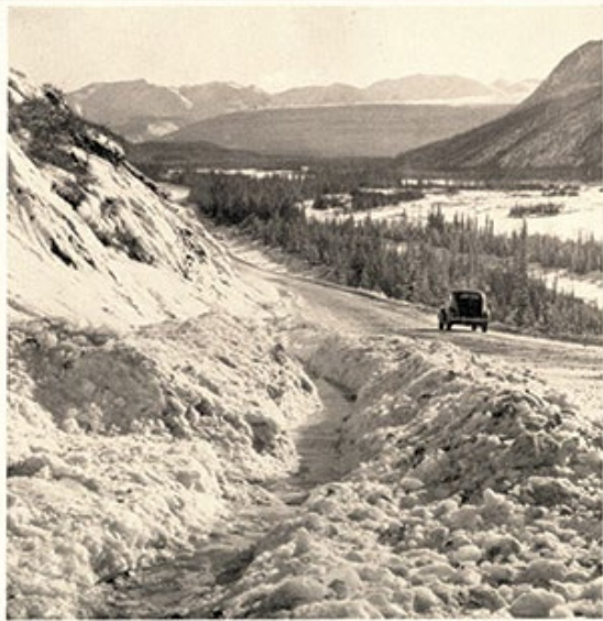
DITCH BLASTED IN ICE—ALASKA HIGHWAY
