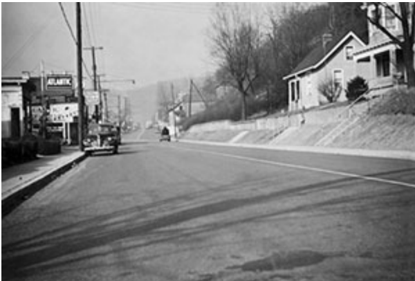
This section of the National Road (U.S. 40) in Wheeling, WV, was reconstructed in 1941 to provide a road width of 12 meters (40 feet).
