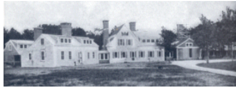
General View of the Association's 'Workshop' South Yarmouth, Massachusetts.
