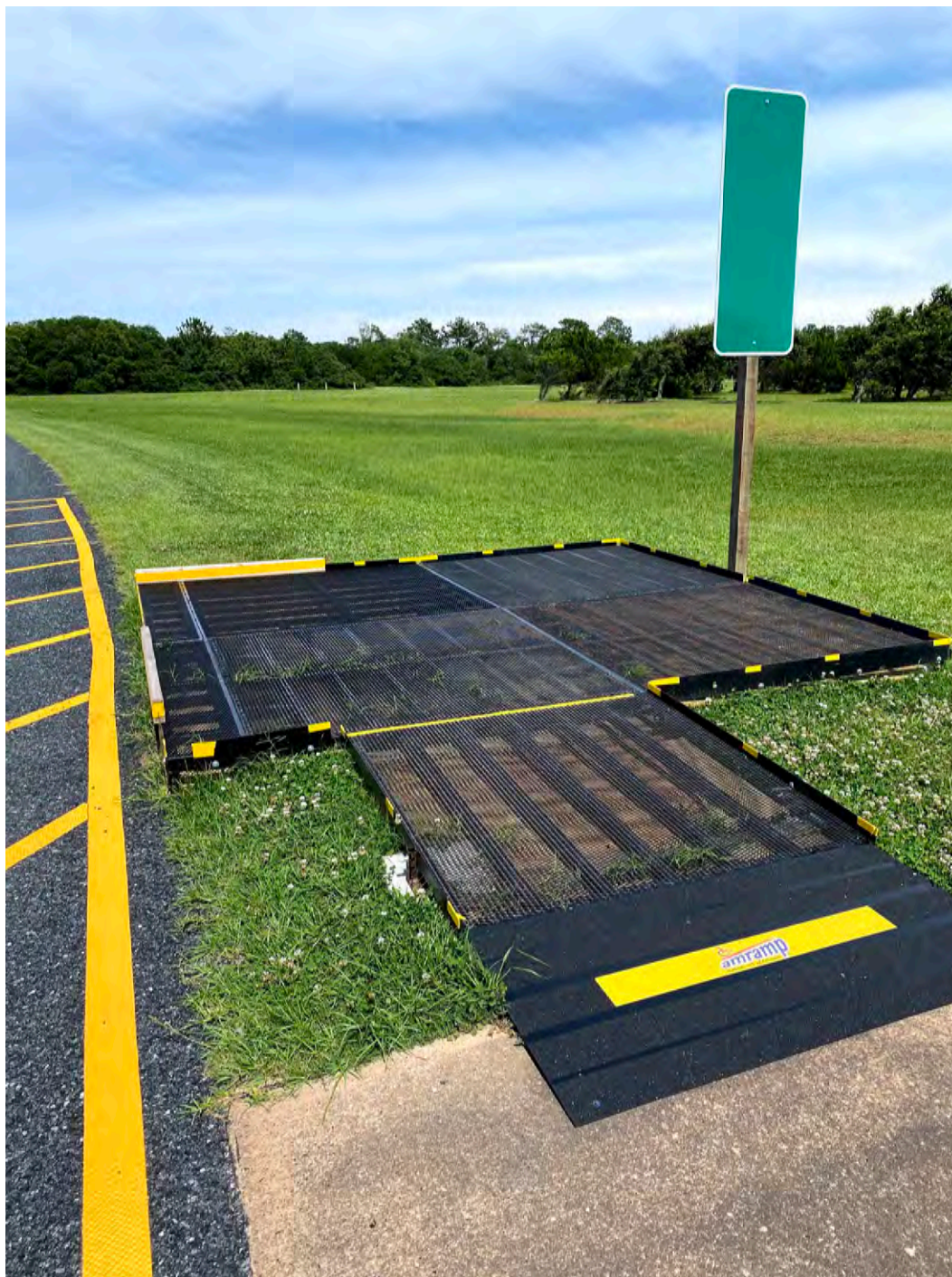
Figure 29: Accesible Ramp and Platform Installed at Sculpture Stop
