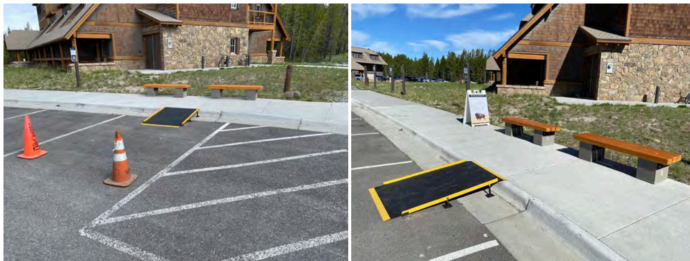
Figure 13: Ramp Installation at the Washburn Stop
