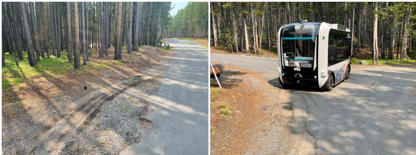
Figure 7: Road Damage Resulting from a Repeated Shuttle Turn
