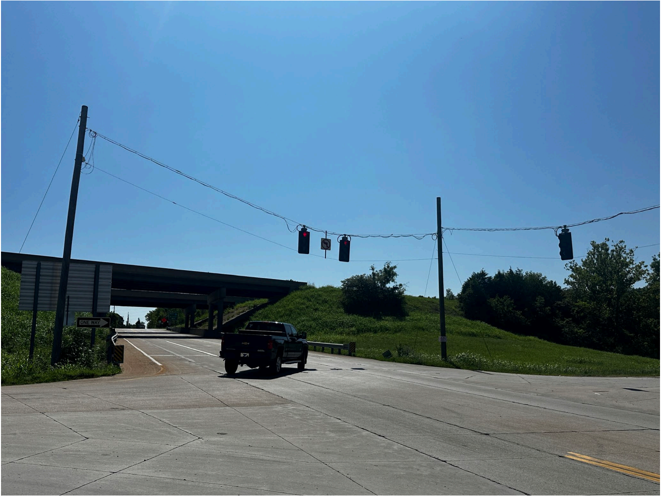
Figure 100. Photo. Example of span wire tension in fair condition.
