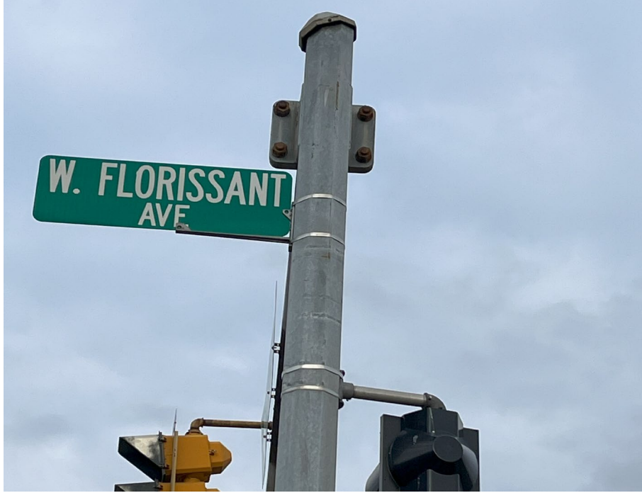
Figure 82. Photo. Example of bolted aerial connection in fair condition.
