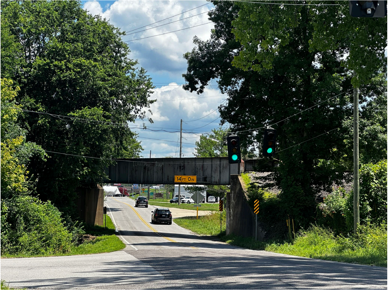
Figure 99. Photo. Example of span wire tension in fair condition.
