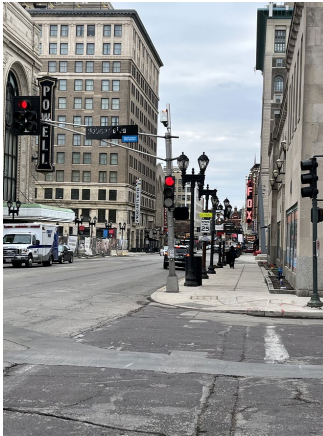
Figure 89. Photo. Pole and post plumbness in fair condition.
