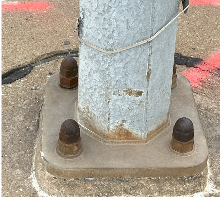
Figure 78. Photo. Example of foundation and base plate connection in fair condition.
