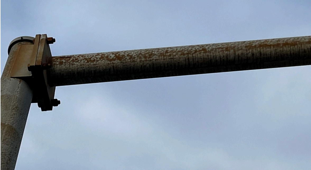
Figure 92. Photo. Example of mast arm in fair condition.
