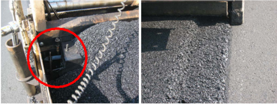
Figure 2.25: Notched Wedge Joint Maker by TransTech Systems, Inc. (Williams 2011)
