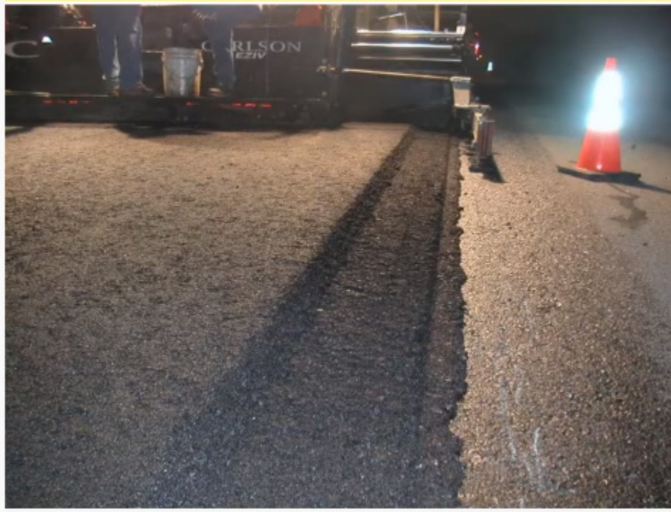
Figure 2.14: Notch wedge joint. ( https://www.equipmentworld.com )
