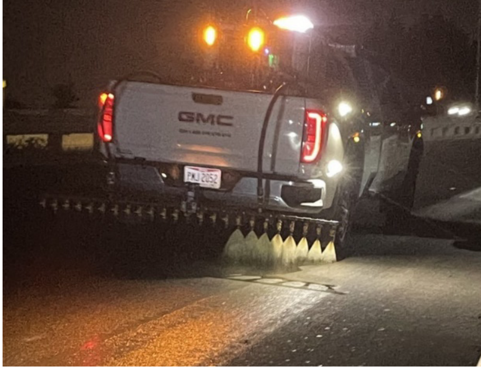
Figure 5.7: Topical emulsion applied on the I5-Kuebler project.
