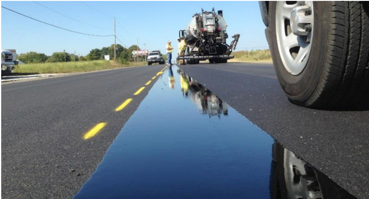
Figure 5.9: Void Reducer applied on the pavement surface (Heritage Inc.).
