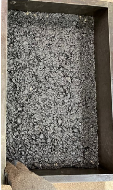
a) Base for longitudinal joint construction
