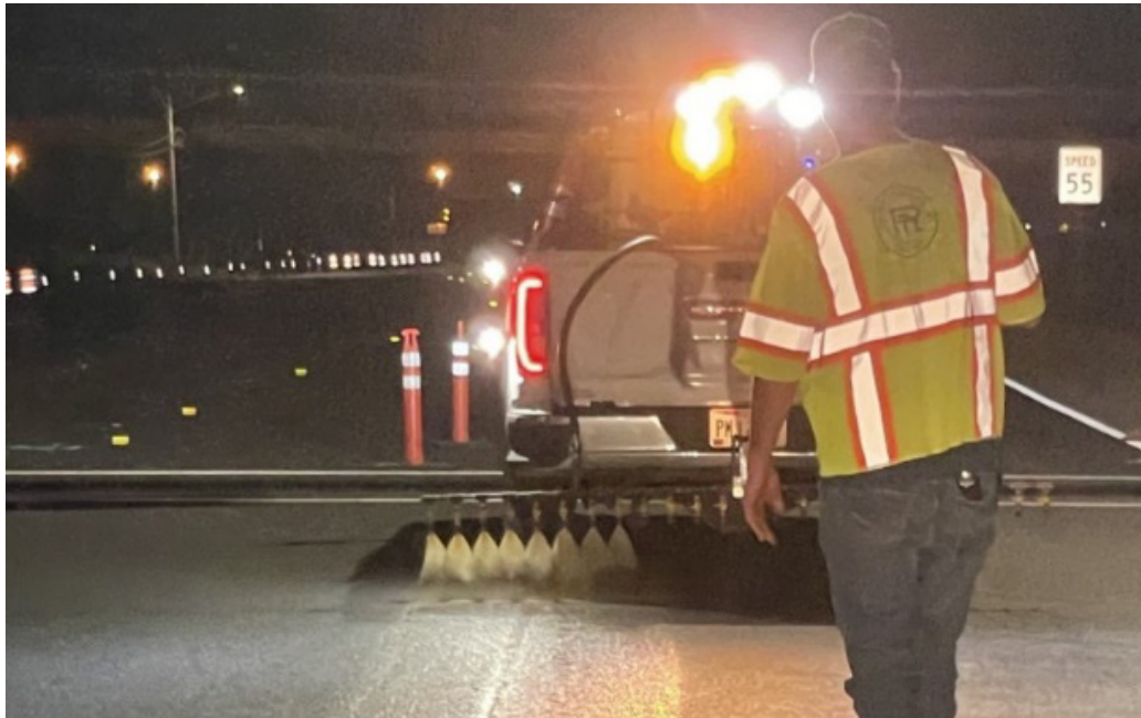
Figure 5.8: Topical emulsion applied on the OR18-McMinnville project.
