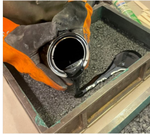
b) Application of emulsion over the base
