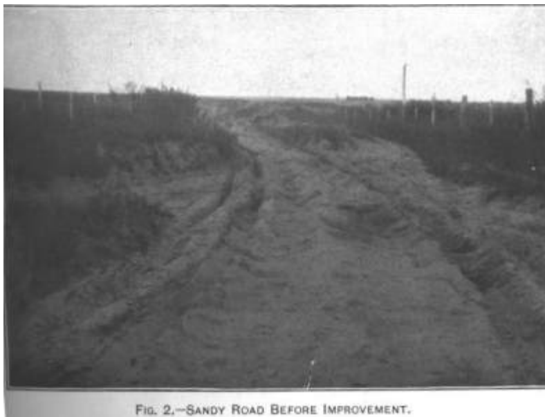
FIG. 2.—SANDY ROAD BEFORE IMPROVEMENT.
