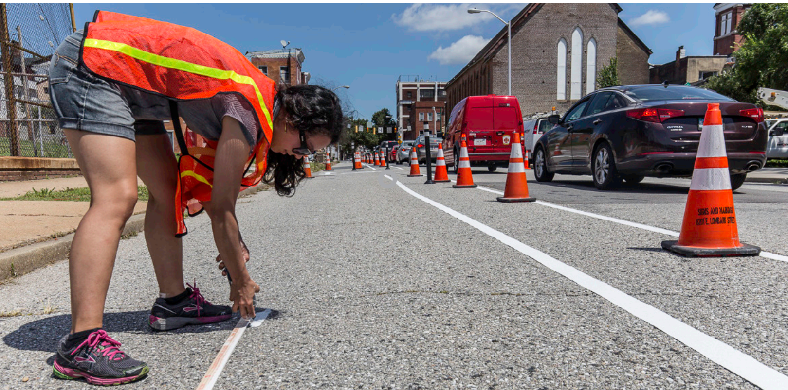
A quick-build, temporary bike lane. Source: Kittelson & Associates, Inc.
