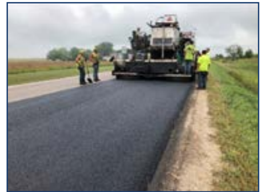
Figure 1. Freshly paved UTBWC section. (Source: MnDOT)
