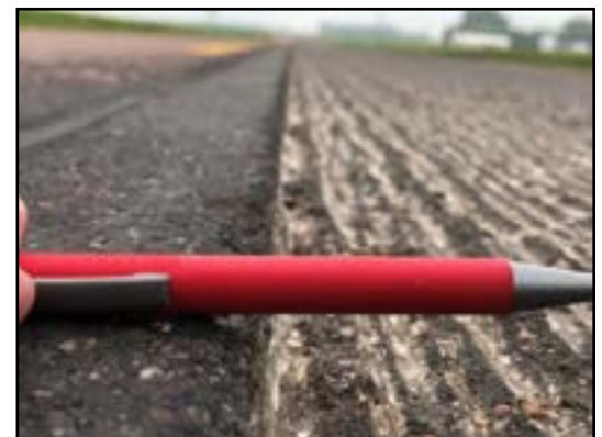
Figure 12. Micromilled surface. (Source: MnDOT)
