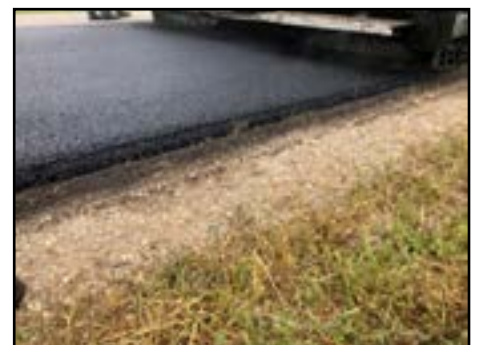
Figure 3. UTBWC paving. (Source: MnDOT)
