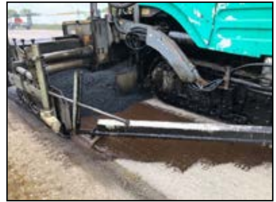
Figure 14. HMA placement on asphalt emulsion membrane during UTBWC installation. (Source: MnDOT)
