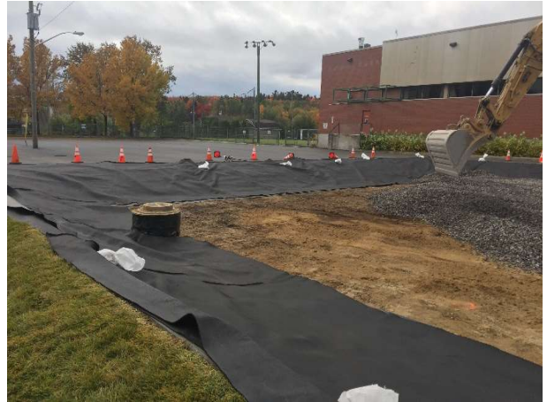
Figure 7. Photo. Geotextile/Impermeable Liner Installation.
