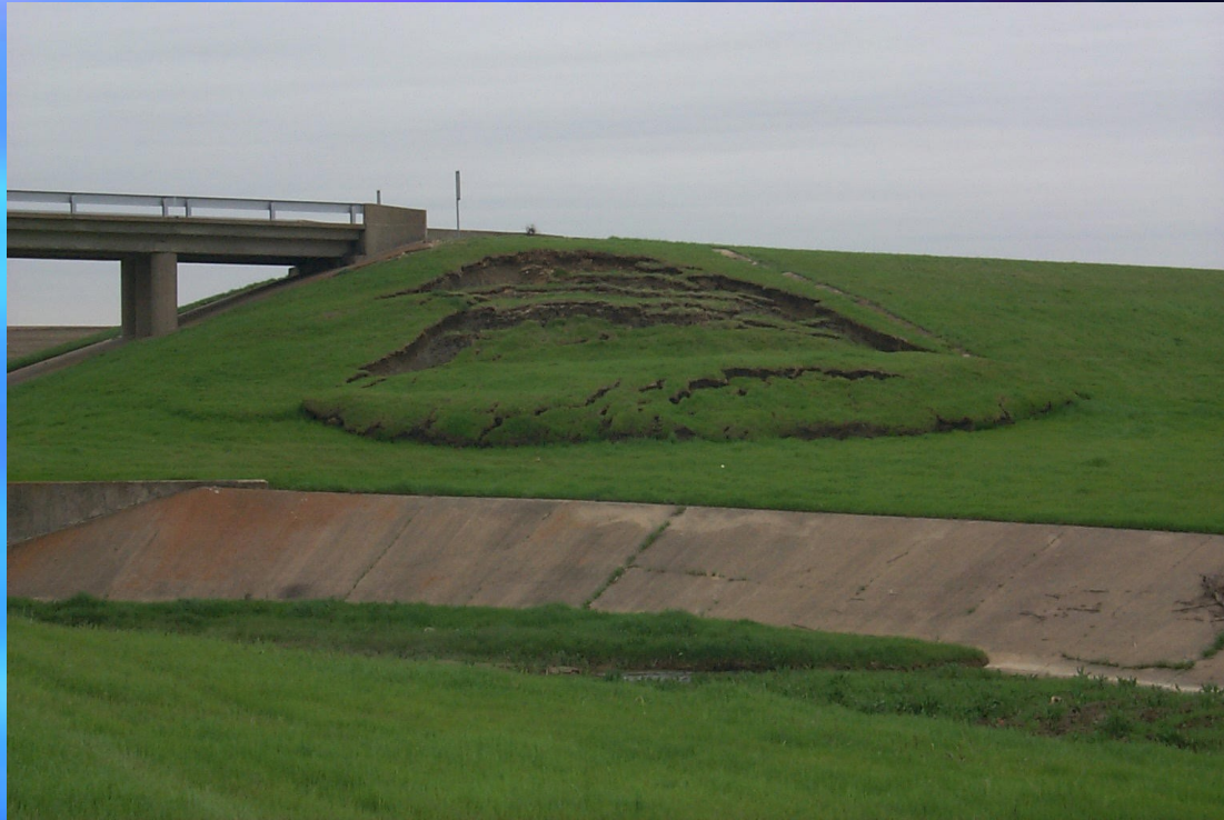
Slope failure
