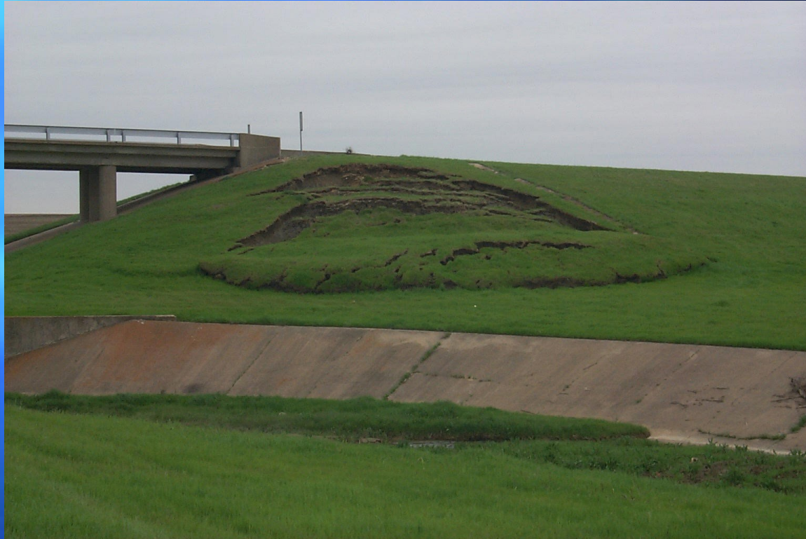
Slope failure
