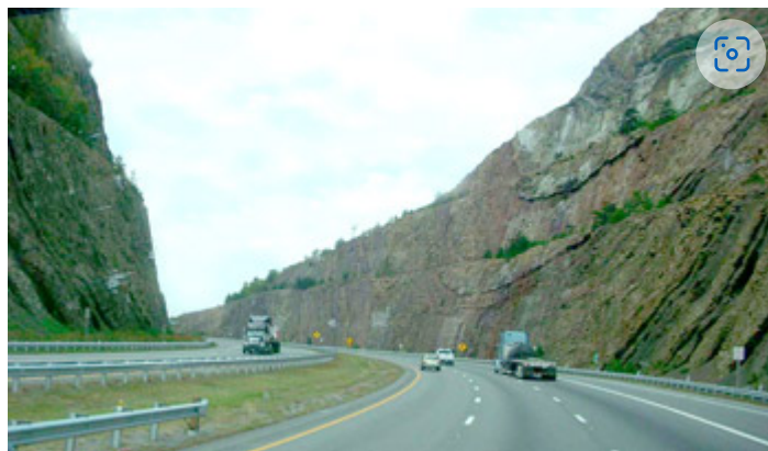
Looking west on Sideling Hill, Maryland. Photo by Rickie Longfellow.
