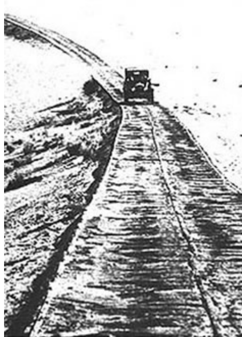
Historic Plank Road of the 1920s. Used with permission from Jim Bremner of Desert USA.
