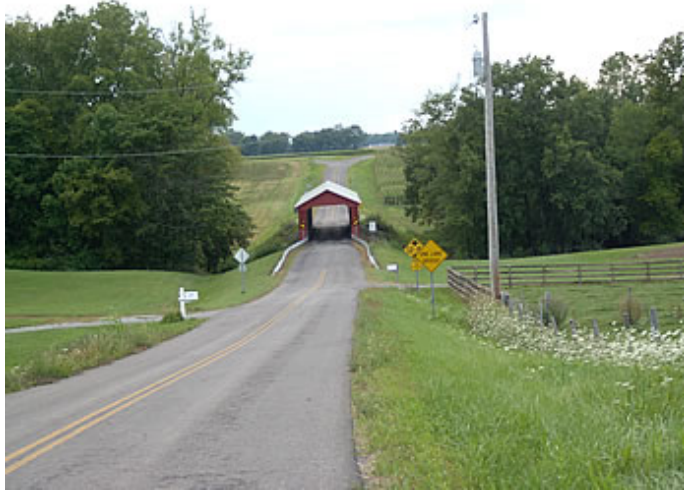
The McColly Covered Bridge was built in 1876. Located near Lewistown, Ohio on CR 13, the 125 foot long bridge crosses the Great Miami River.
