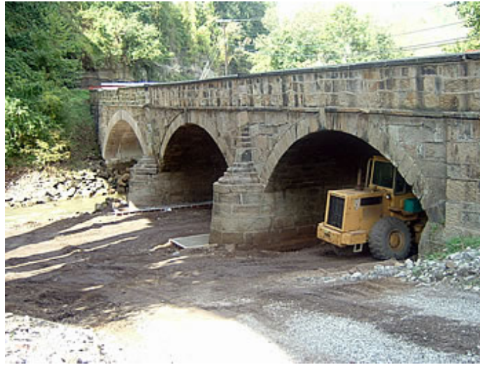
Westerly view of 3 arches of the Blaine Bridge.
