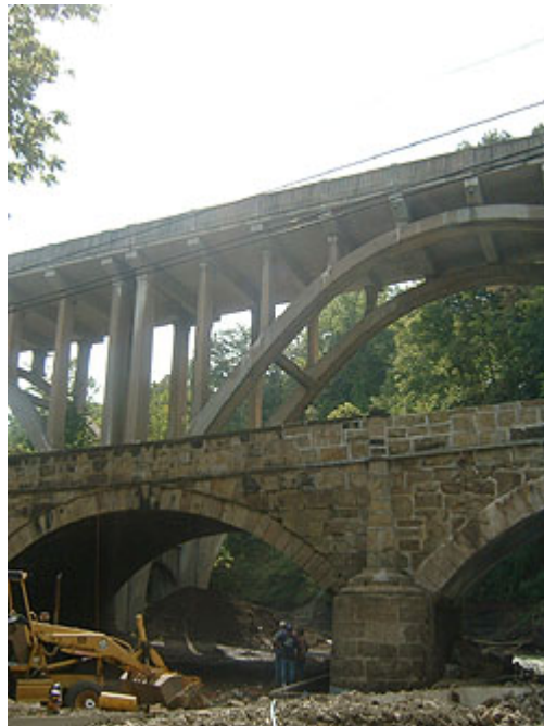
The Blaine Bridge, looking south with SR-40 overhead.
