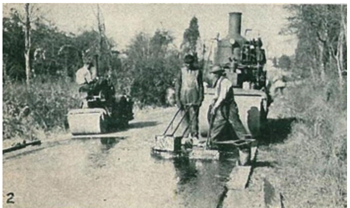
Putting on the seal coat.
