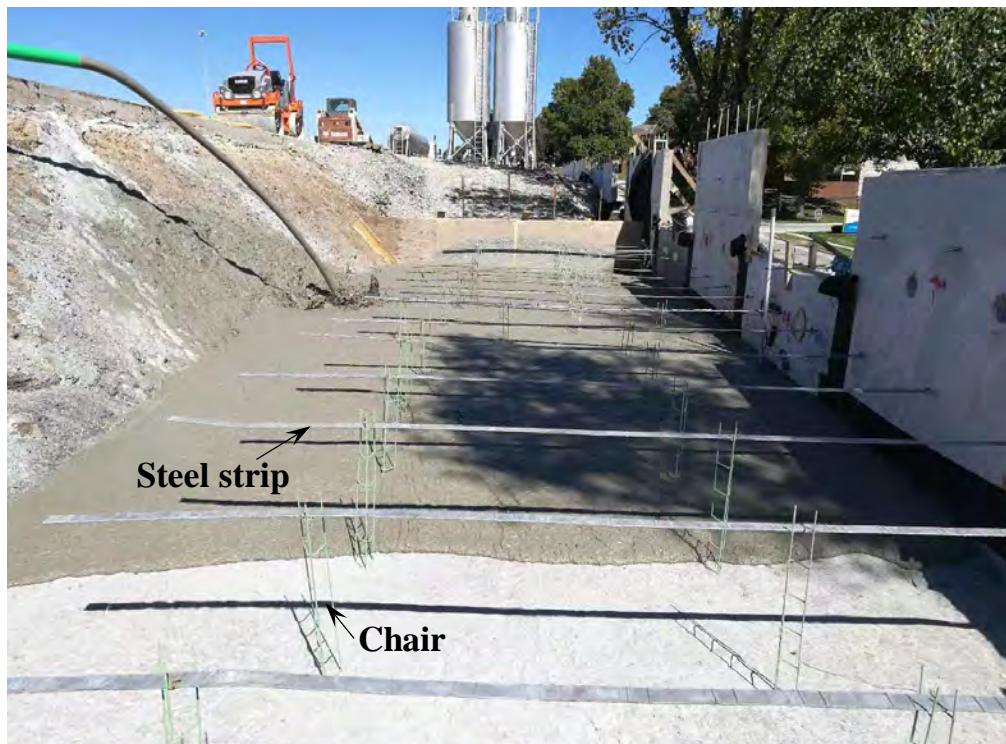
Figure 2.5: Placement of the Second LCC Layer
