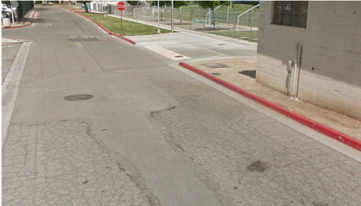
Figure 7. Site #1 on Fresno State Campus, Cracking, Joint Deterioration, Roughness, Surface Defects
