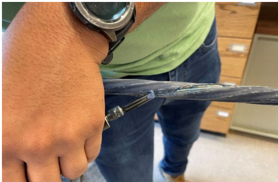
(b) Removing epoxy with electric chisel
