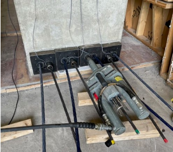
(a) Stressing uncoated strand in box-beam specimen
