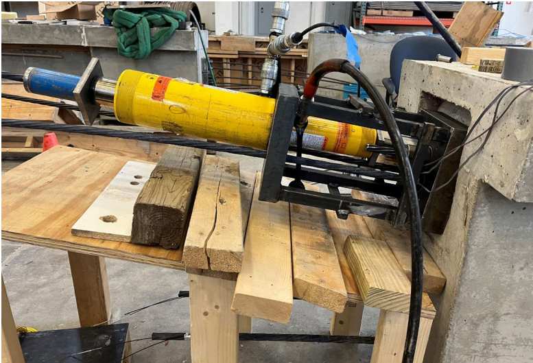
(b) Stressing epoxy-coated strand in I-beam specimen
