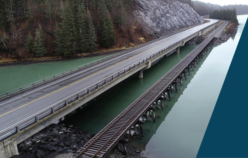
Figure 11: FRA's Consolidated Rail Infrastructure and Safety Improvements Program awarded funding to the Alaska Railroad Corporation to replace an aging bridge along the main rail route between Anchorage and Fairbanks, AK. (Photo Credit: Alaska Railroad Corporation) 51
