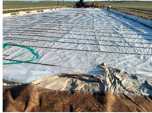
Curing ongoing at FM 119
