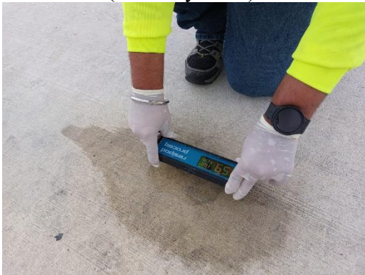
SR tests on deck, Span 3 (August 2023)
