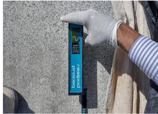
SR tests on deck, Span 8 (August 2023)
