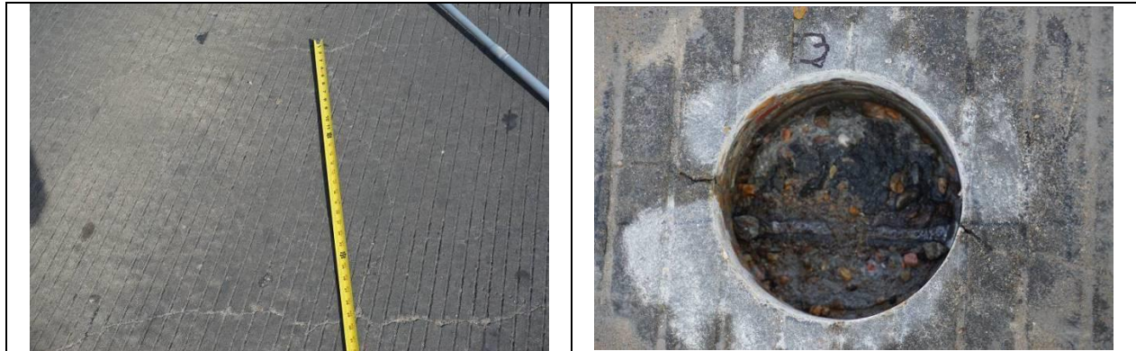
Core on top of rebar (shows corrosion) at transverse crack location on Bridge Deck #8
