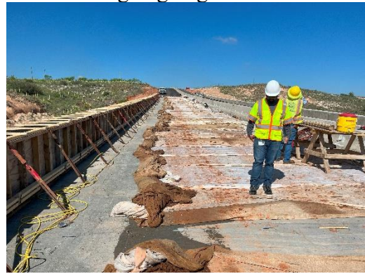
FM 2277 Bridge deck at the time of visit
