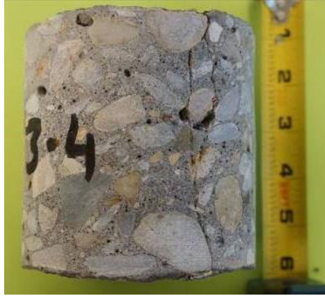
Full depth transverse crack propagation on core from Bridge Deck #3
