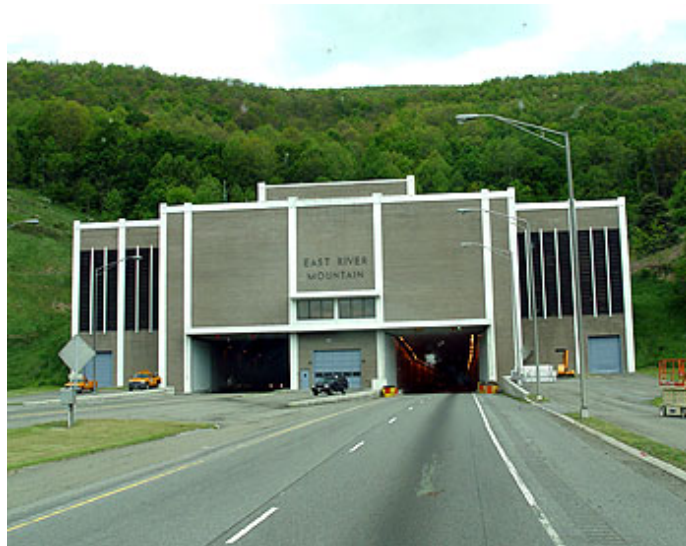
East River Mountain Tunnel.
