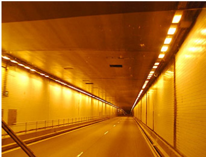
Inside of East River Mountain Tunnel.
