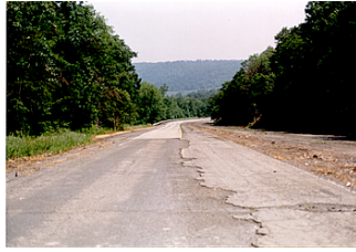
The eastbound lanes of the abandoned turnpike west of Ray's Hill tunnel.
