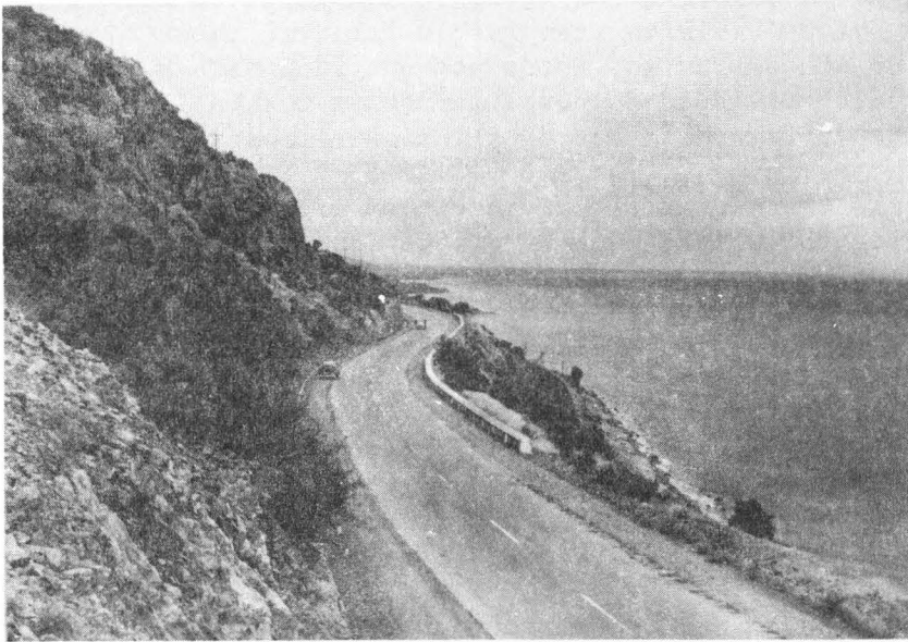
Izmit-Hereke Road along the shore of the Sea of Marmara
